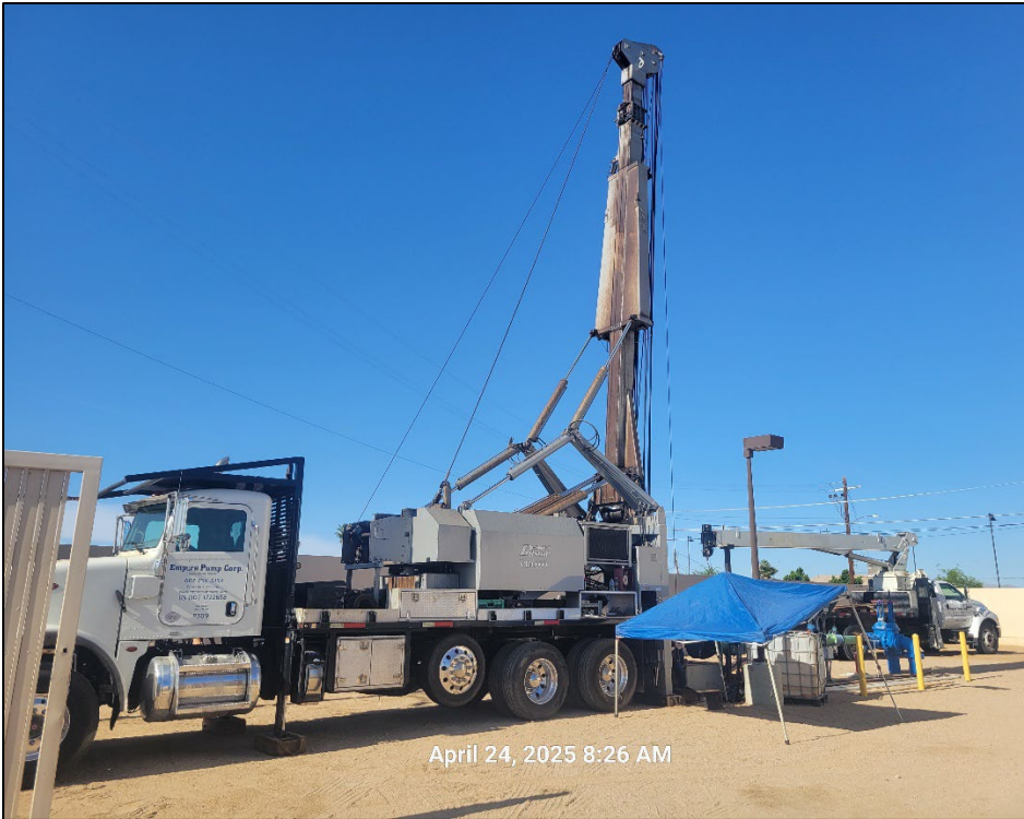
Alto Well Project – Column Pipe Removal
