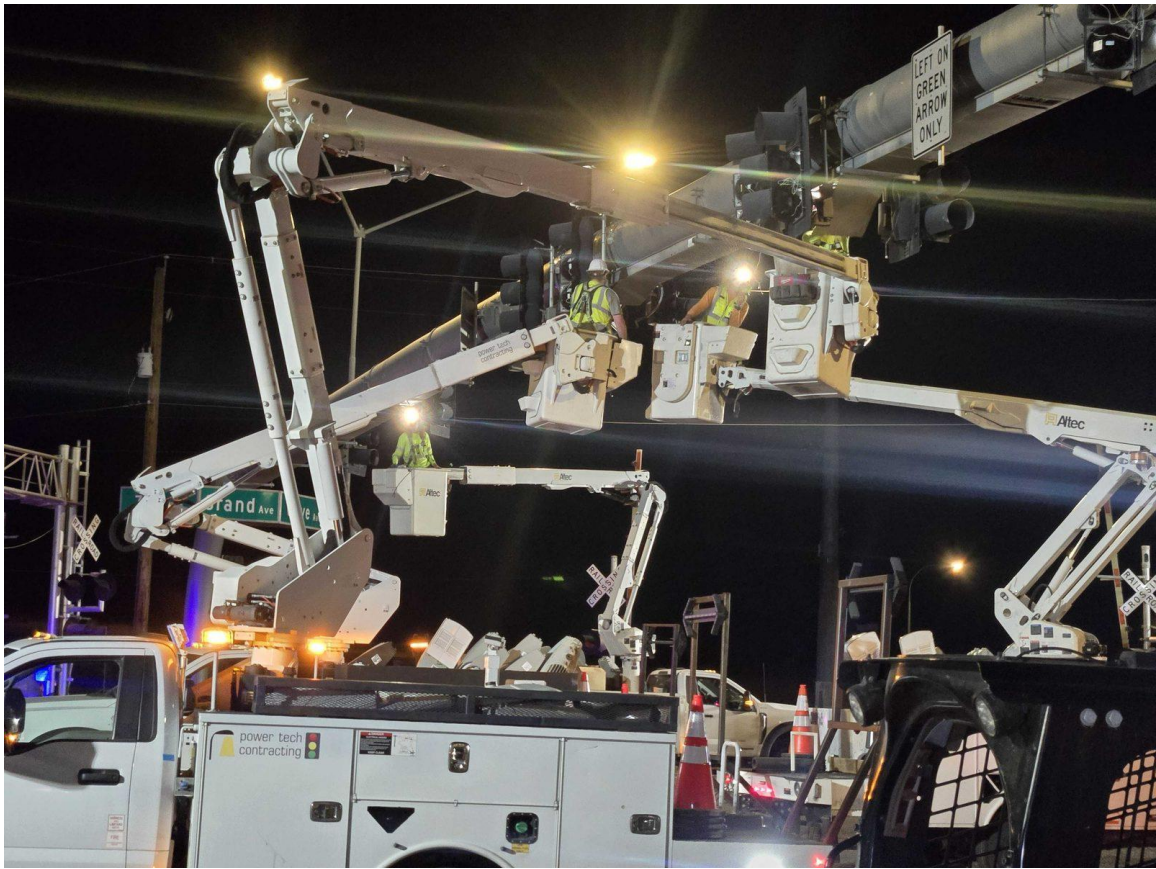
Power Tech crews performing overnight traffic signal work with company-owned aerial equipment.
