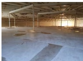
Canterbury Water Tank
