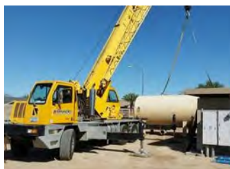
Cottonwood Tank Removal
