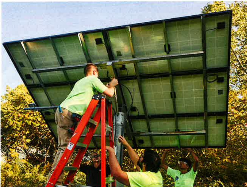
- International Brotherhood of Electrical Workers installing Solar Panels
