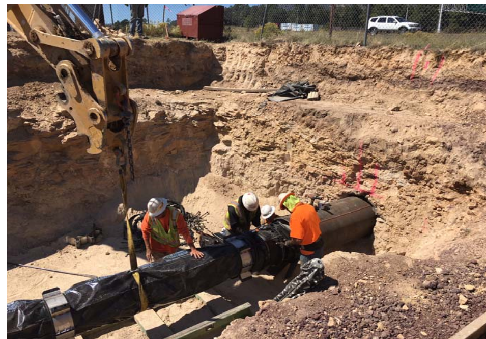
Replacement of water line under I-40
