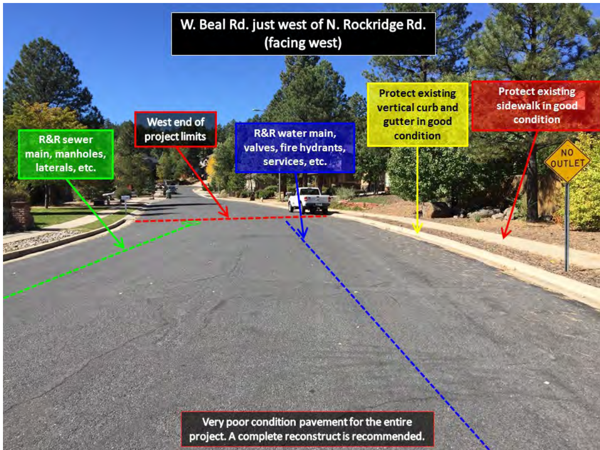
Figure 2. R&R water/sewer mains & appurtenances, and pavement section.
