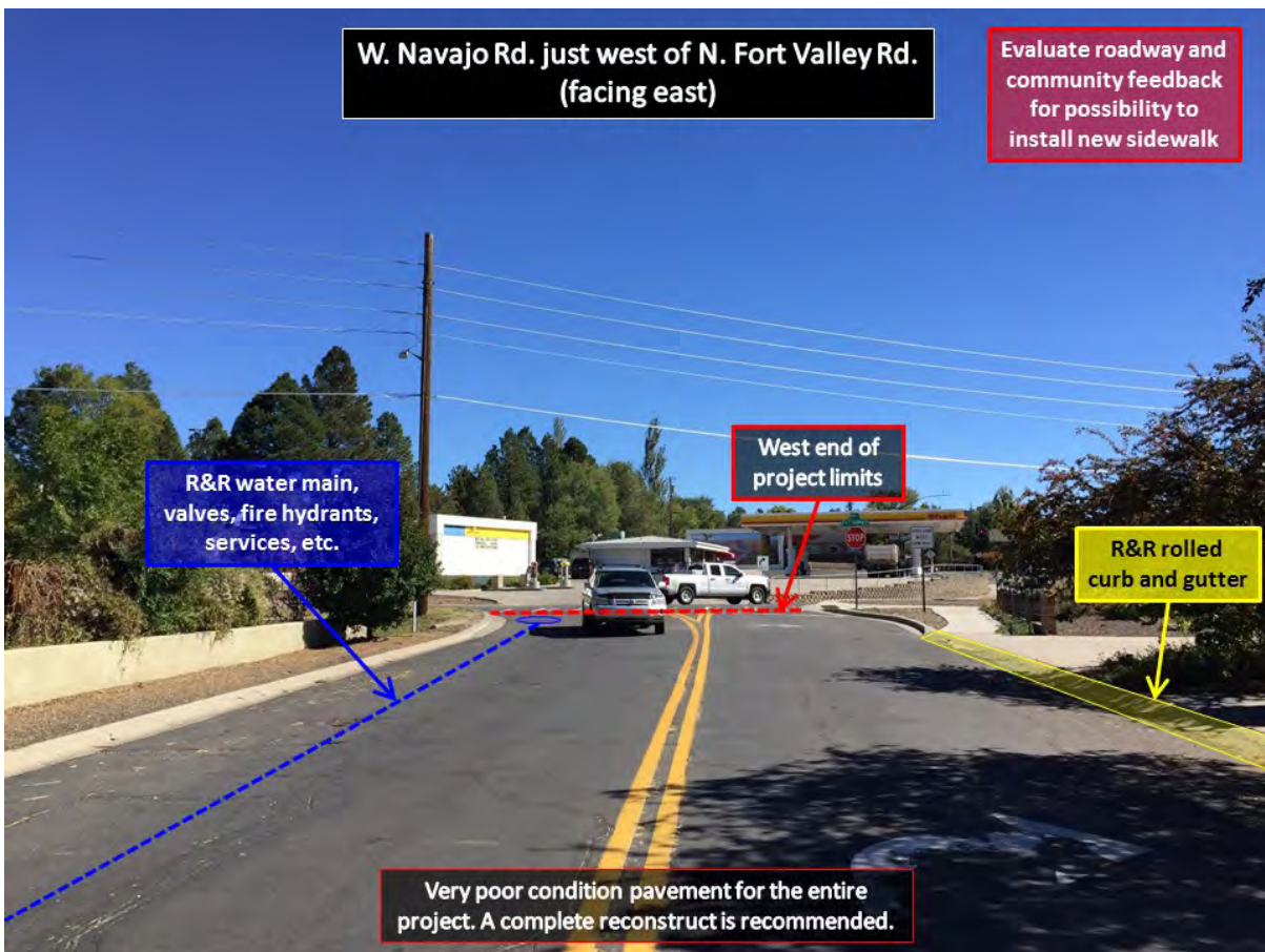
Figure 18. R&R water main and appurtenances, pavement section, and rolled curb and gutter.
