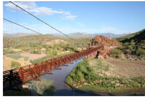
Figure 8 – Source: bridgemeister.com. Replica suspension bridge at Verde River.
