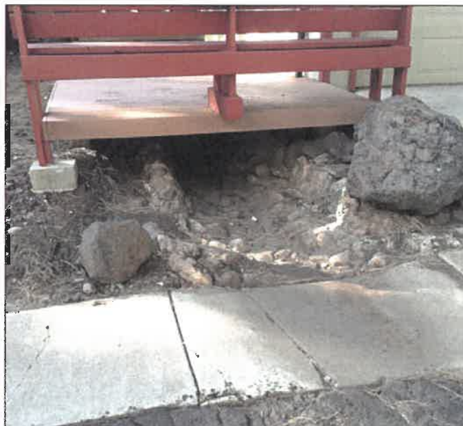
Figure 8: Rock Channel Termination Under Unit 23 Deck (Looking West)
