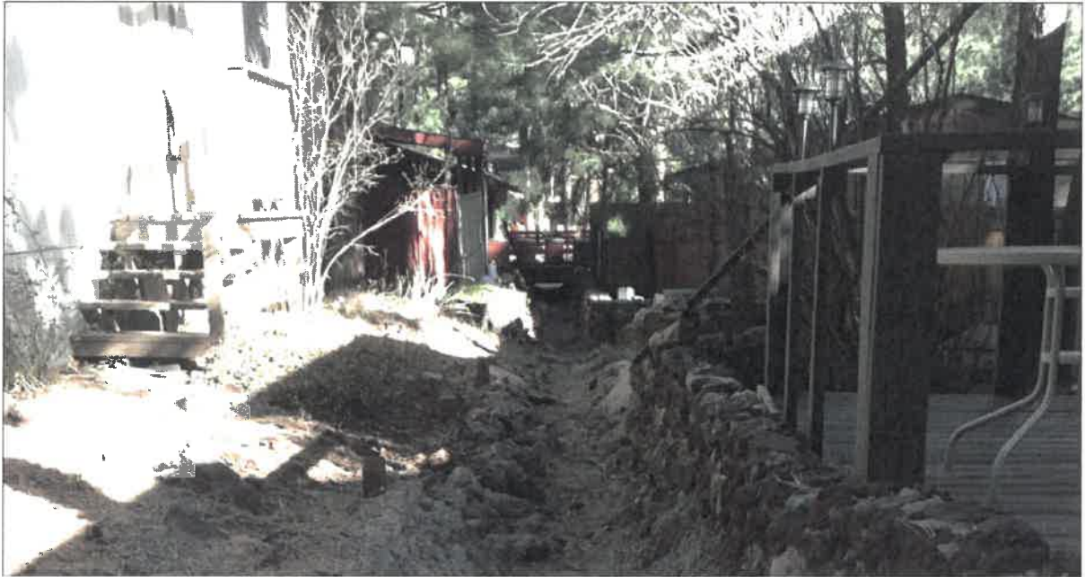
Figure 7: Rock Channel Between Units 17, 18, 23 And 24 (Looking East)
