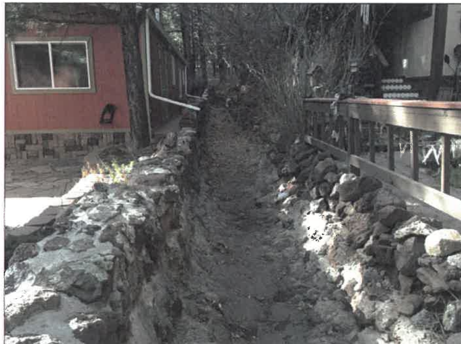
Figure 5: Rock Wall Channel Between Units 8 And 9 (Looking West)
