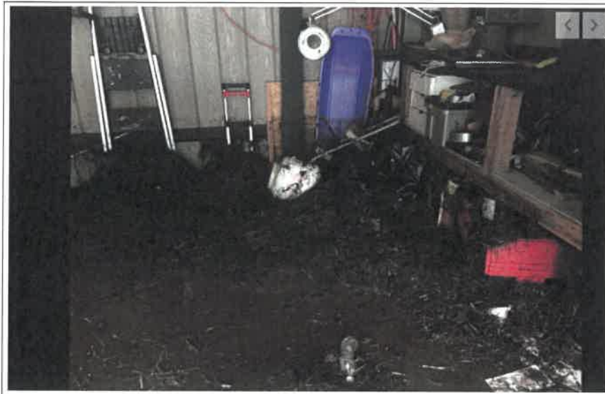
Floods in the Wildwood Hills Mobile Home Park caused extensive damage to homes and garages.
