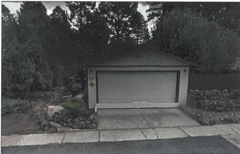
Figure 11: Image of Gates At Garage Installed By Residents (Unit 17)
