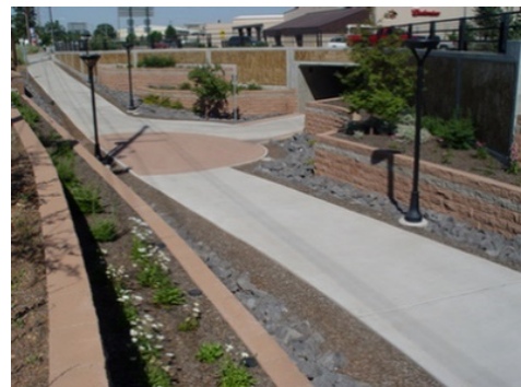
Figure 4: Butler Ave-Enterprise Underpass
