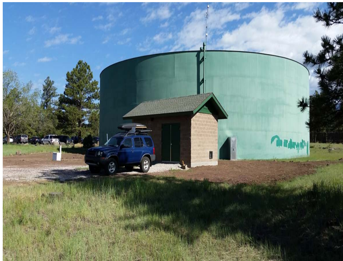
Buffalo Park Reclaimed Water Tank
