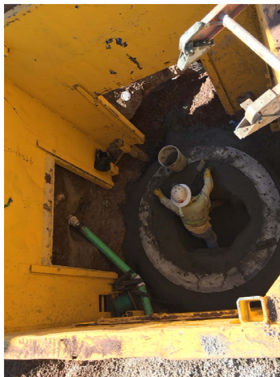
Replacing undersized west-side sewer line
