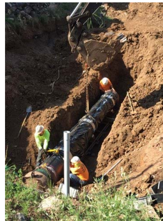
Replacing undersized west-side sewer line
