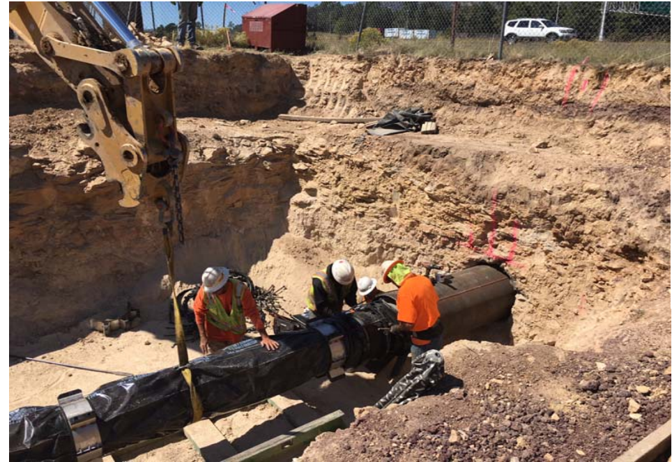
Replacement of water line under I-40
