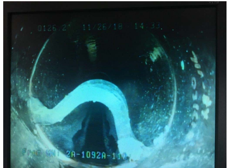
Sewer TV inspection shows gasket installed wrong
