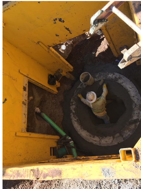
Replacing undersized west-side sewer line
