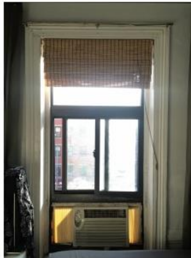
Emergency escape and rescue opening operation in existing b
