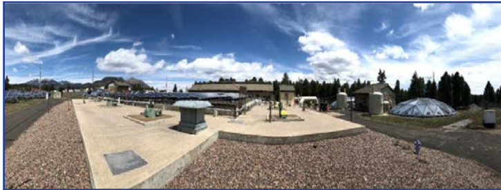
The RDFWRP currently treats about 2 mgd. Although all solids produced at the facility are sent to the WHWRP for treatment, the RDFWRP has full liquids treatment capability.
