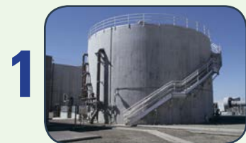
1 Digester Expansion at WHWRP
