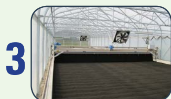
3 Biosolids Solar Drying at WHWRP
