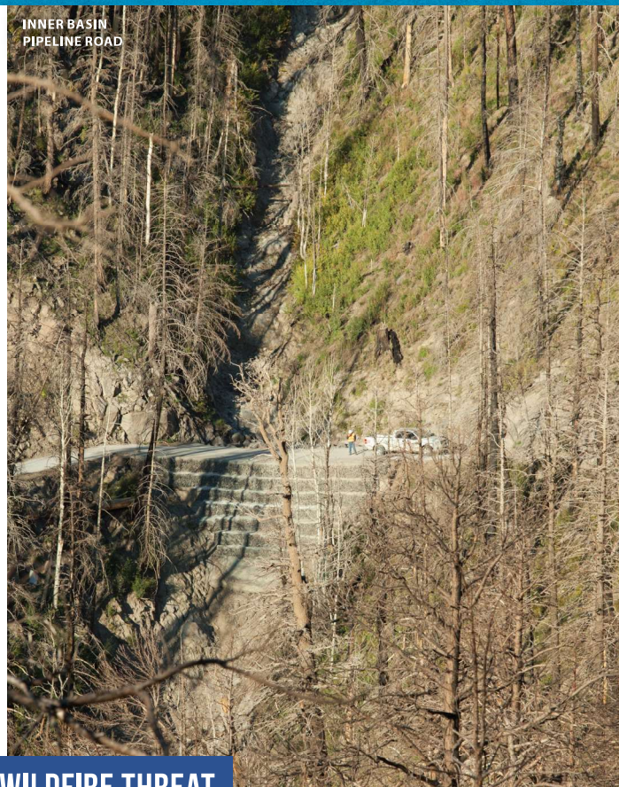
NEWMAN FIRE PROTECTION, INCIWEB IMAGE
