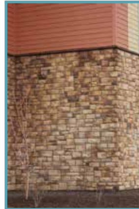
Rough face cut stone, red sandstone, limestone, granite or others with mortar joints
