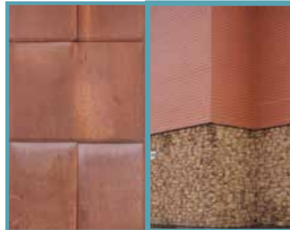
Metal shall be panels of 6" plus face with folded or standing seams. Corrugated galvanized metal is not allowed.
