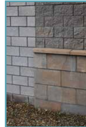
Cement block (CMU) split face or textured face, used similar to rough cut stone, encourage colored block vs. plain cement, or utilize a combination of colored and cement
