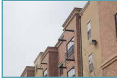
Brick may be carried up from the base floor, and applied part way up or full height as a vertical accent for an area of the facade complimenting adjacent materials. The brick may also be the facade of the entire building, but the base first floor should have some differentiation and horizontal separation and/or detailing
