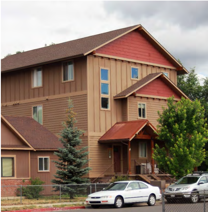
Figure 7: New duplex on South Leroux Street
