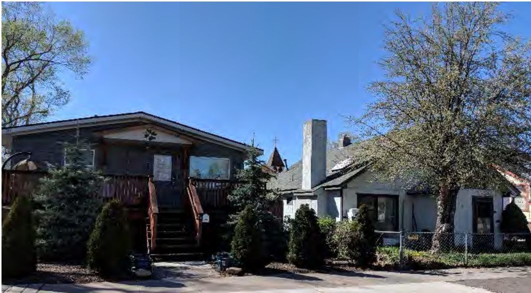
Figure 34: A home raised above the flood depth and one grandfathered in side-by-side
