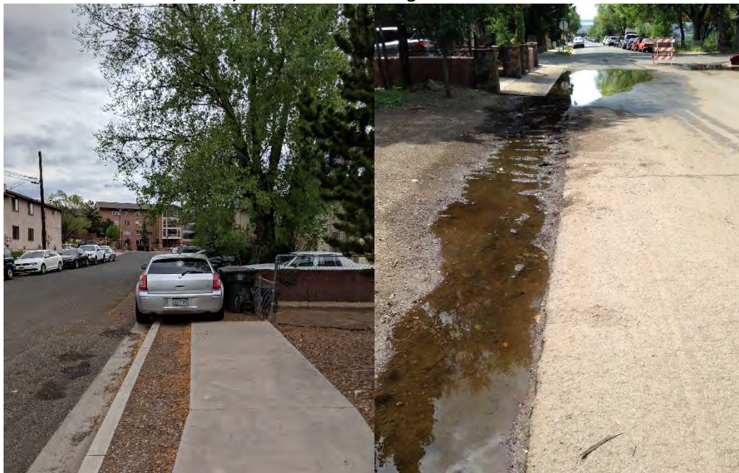
Figure 27: Examples of missing local stormwater, sidewalk, and curb infrastructure in the Southside
