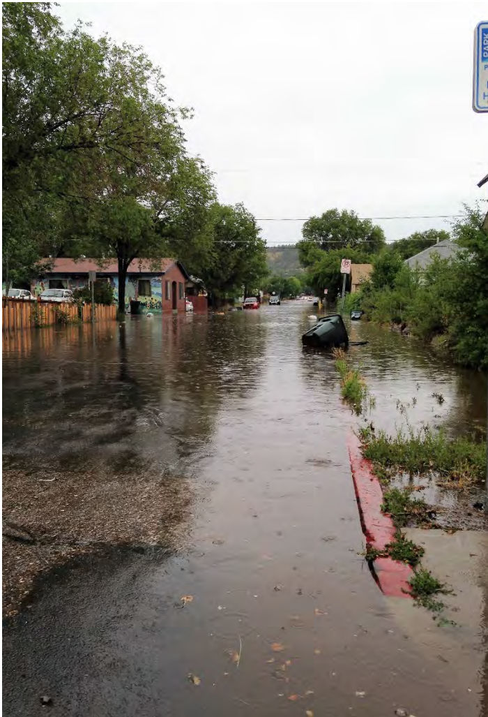
Figure 35: Localized flooding sometimes called "Lake Dupont" on Dupont Avenue
