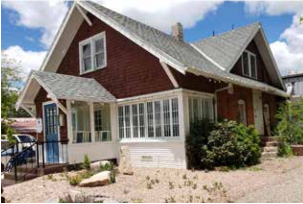
Craftsman house on Cottage Avenue currently operating as a restaurant
