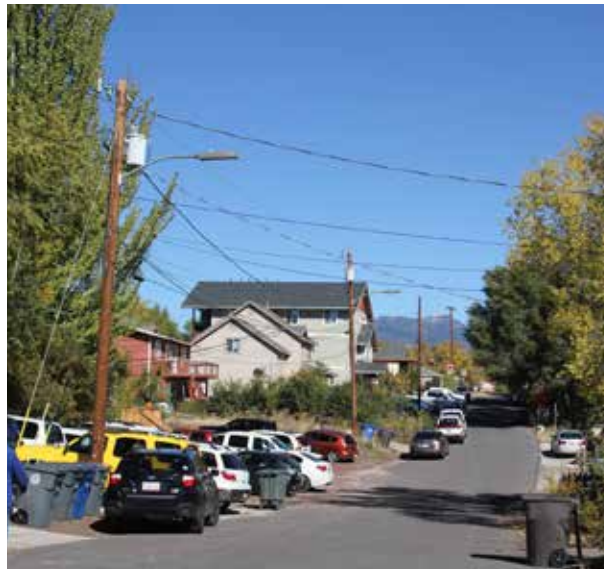
South Fontaine Avenue south of Franklin Avenue demonstrating irregular parking due to lack of curb, gutter and sidewalk
