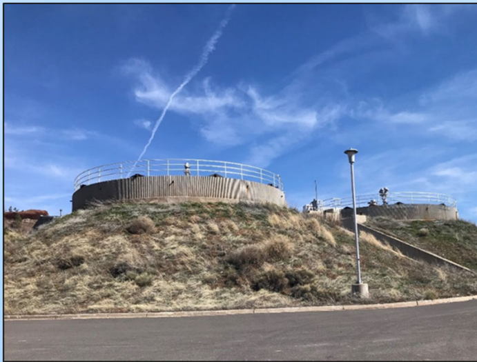
Existing Anaerobic Digesters at Wildcat Hill WRP
