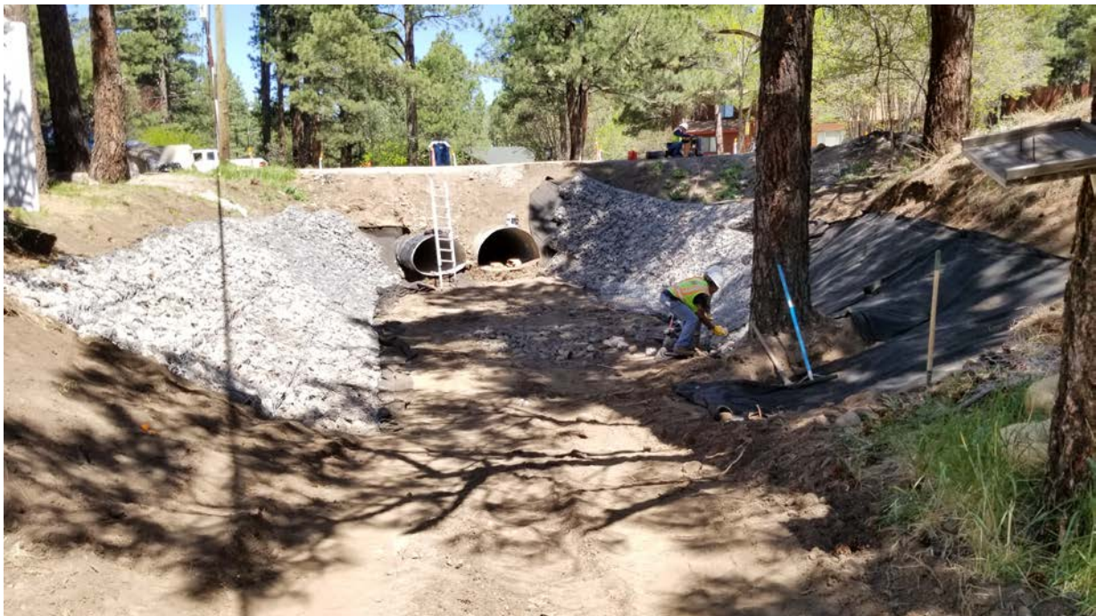
I-40/Fourth St Bridges -
