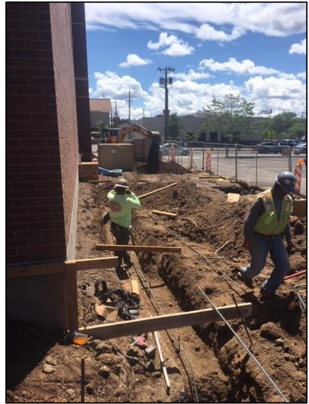
Sally Port area at the south of building
