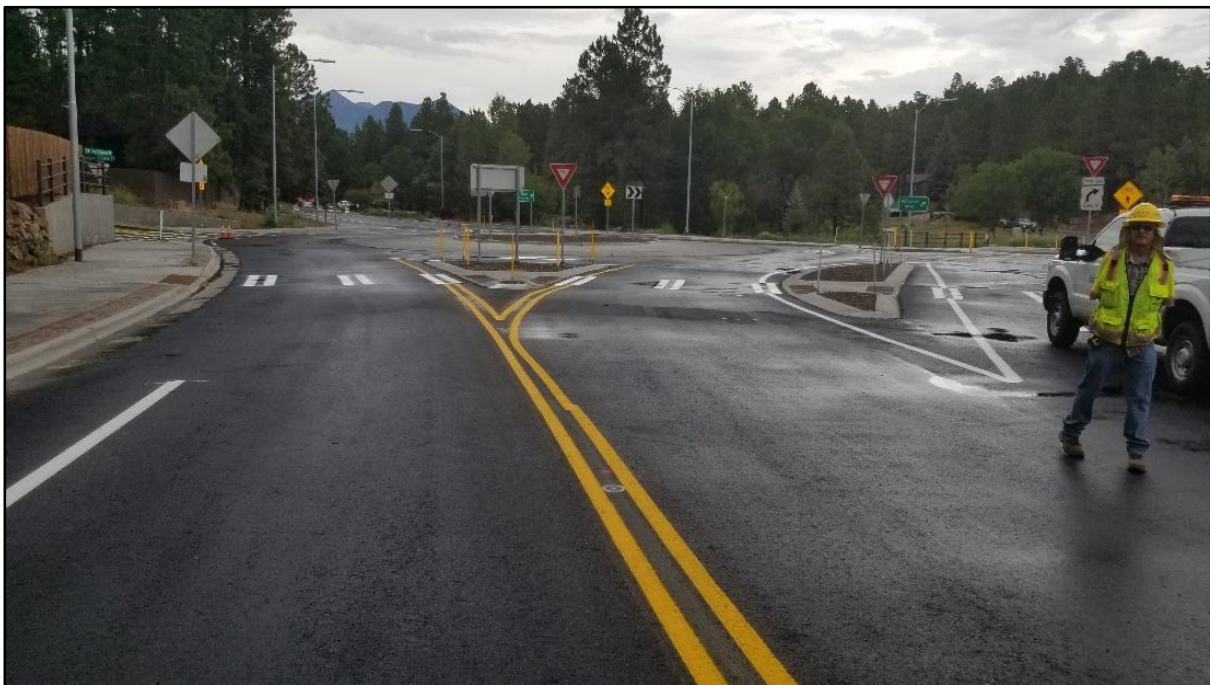
Corrected pavement looking north
