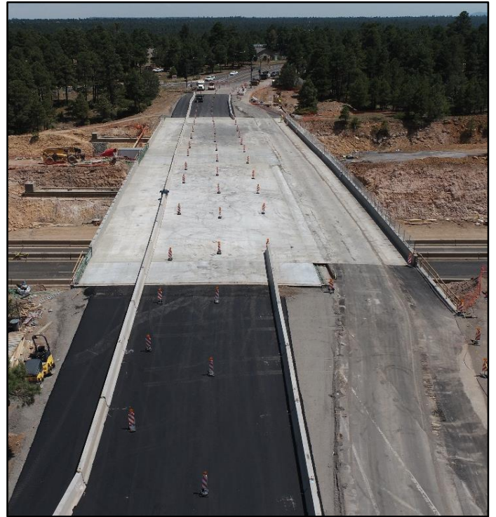
Fourth Street Bridge – Just Before Opening to Traffic
