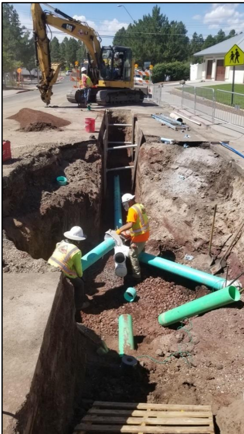
Sewer main replacement Navajo/Hopi looking south
