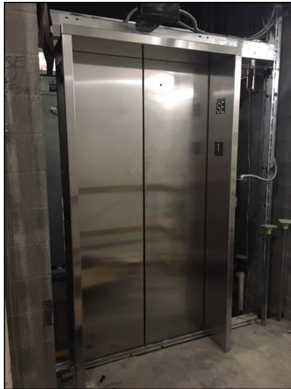
Staff Elevator is substantially complete
