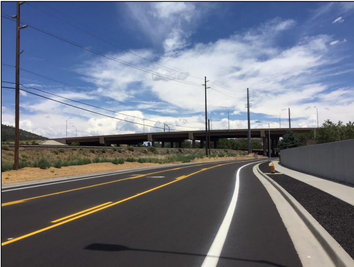
Roadway During Construction & Final Improvement
