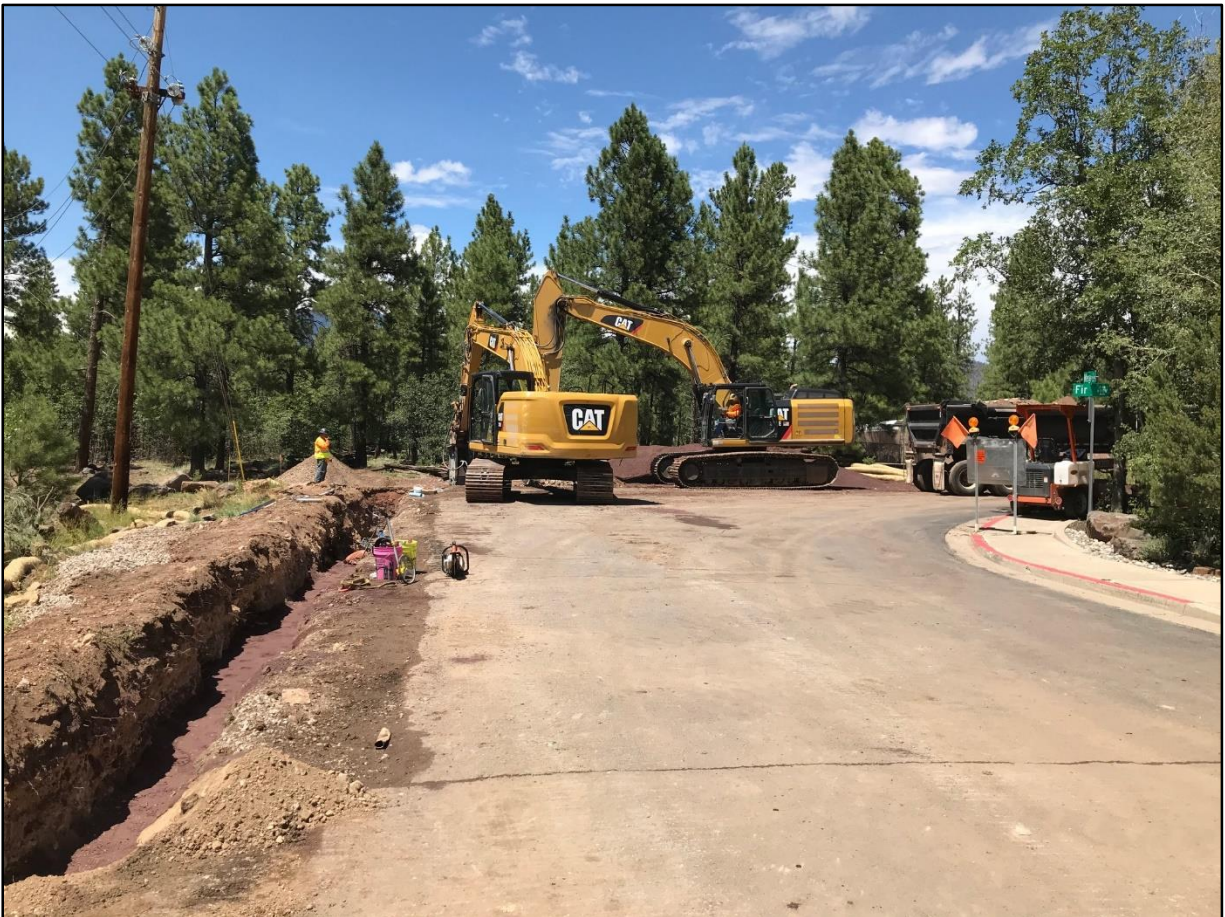
Backfilling a trench
