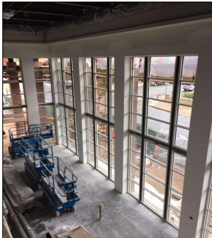
Lobby windows are installed.
