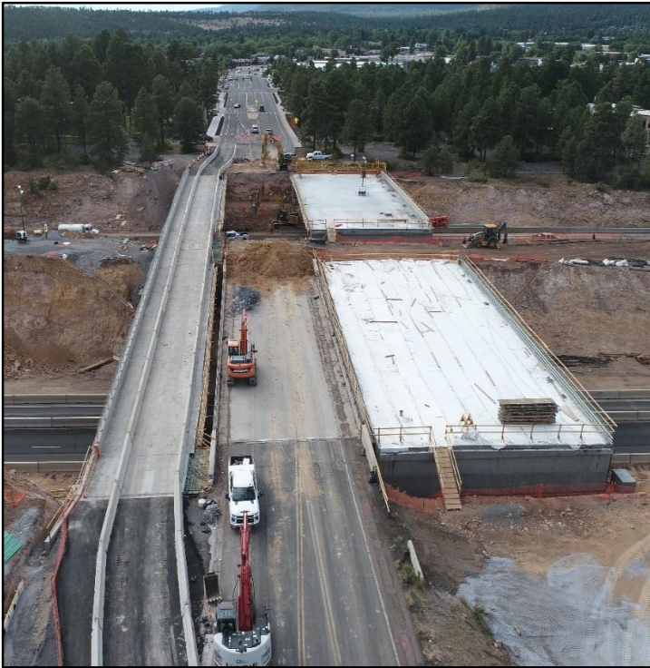
Fourth St. Bridge – Before bridge slides
