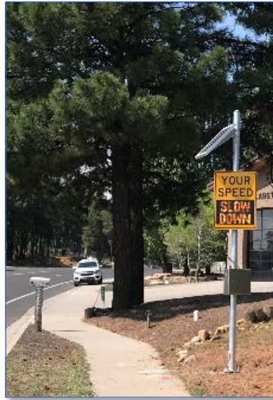
Radar Feedback signs with 32 MPH speed displayed and SLOW DOWN message displayed.
