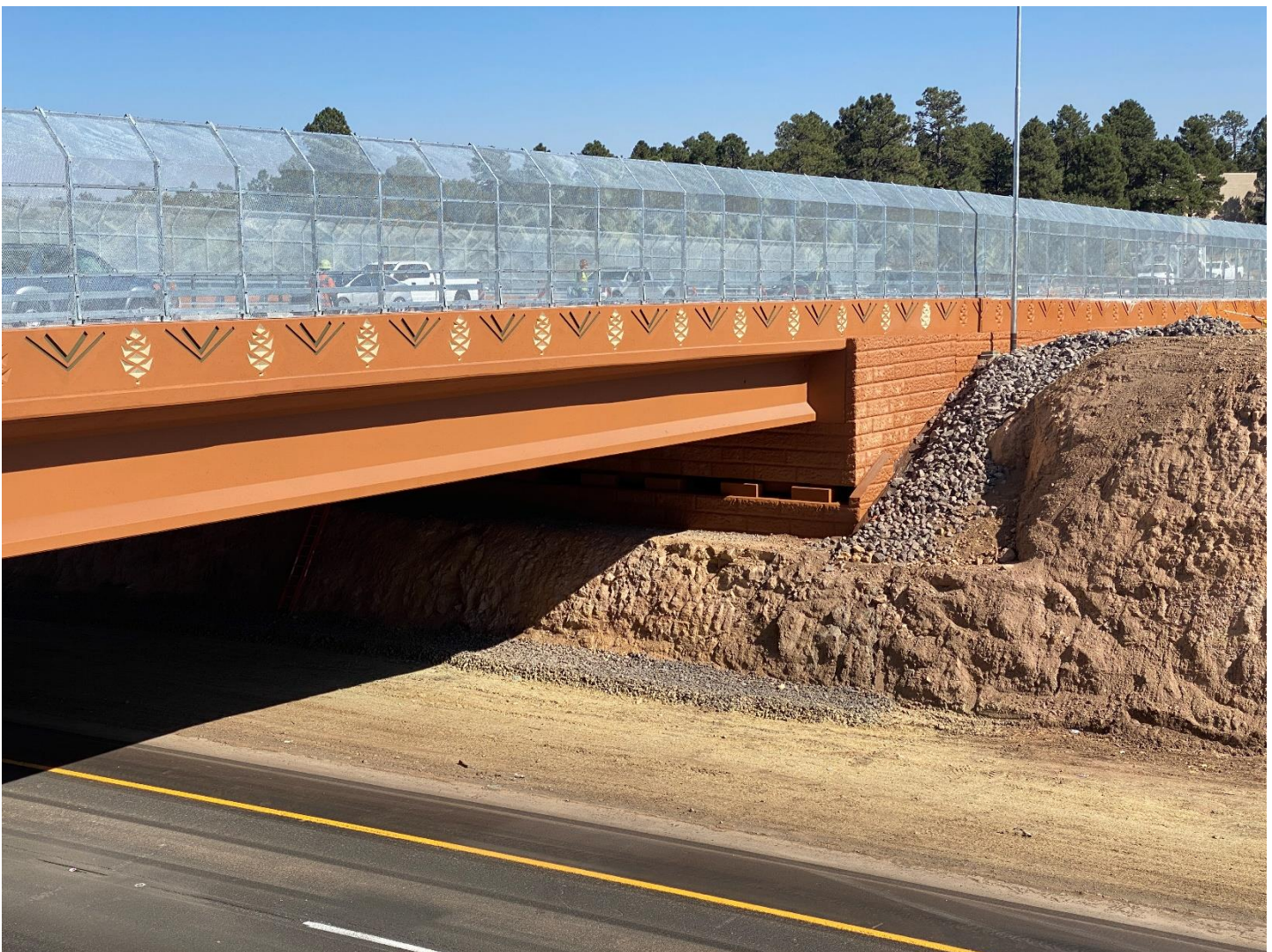
Fourth St. Bridge – Construction continues
