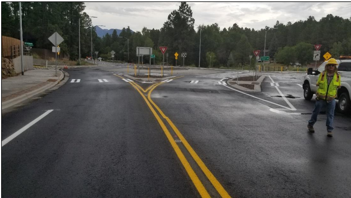
Corrected pavement looking north
