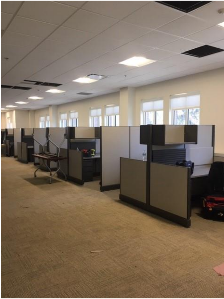
Furniture being installed in the Court Customer Service staff area
