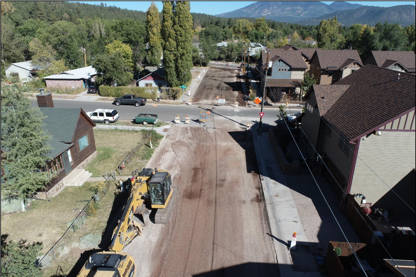
Summit Water Project-Pavement removal on Walnut Street
