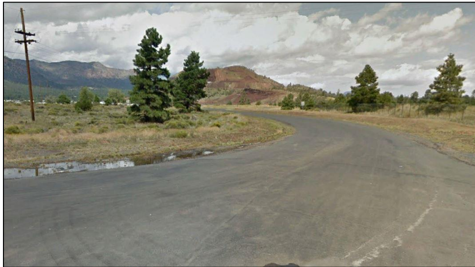
Intersection of Rt. 66 and El Paso Flagstaff Road looking north towards the Wildcat plant where the waterline will extend to
