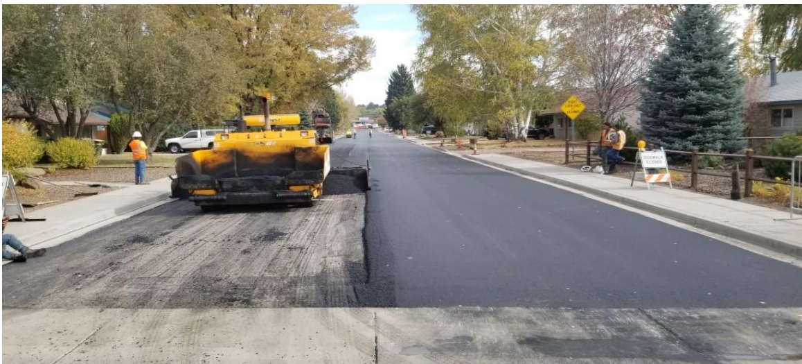
Pavement correction operations looking east on Navajo Road
