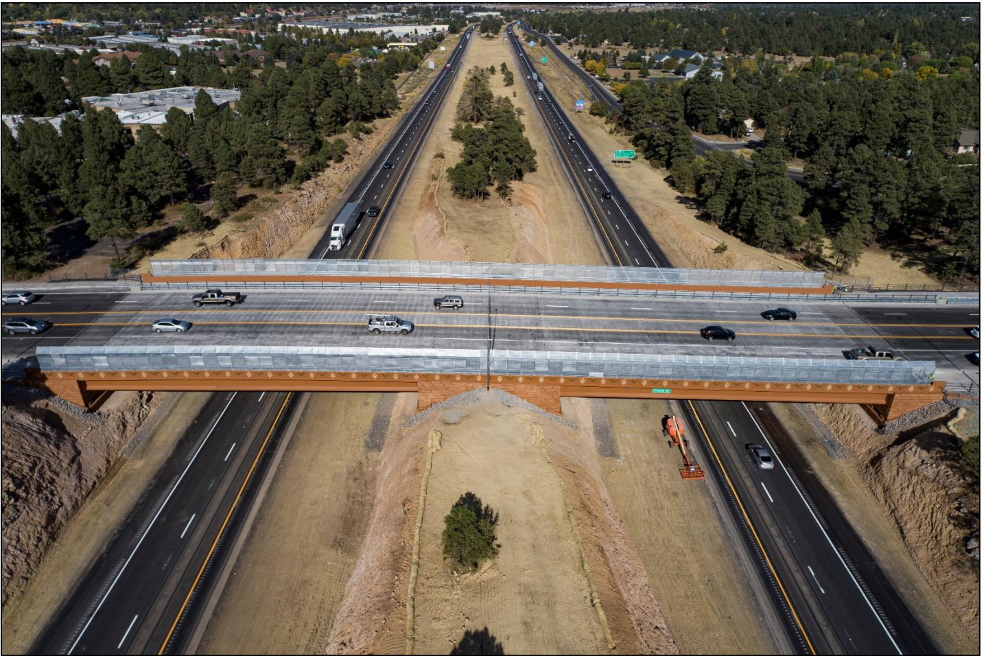
Fourth St. Bridge – Construction approaches completion
