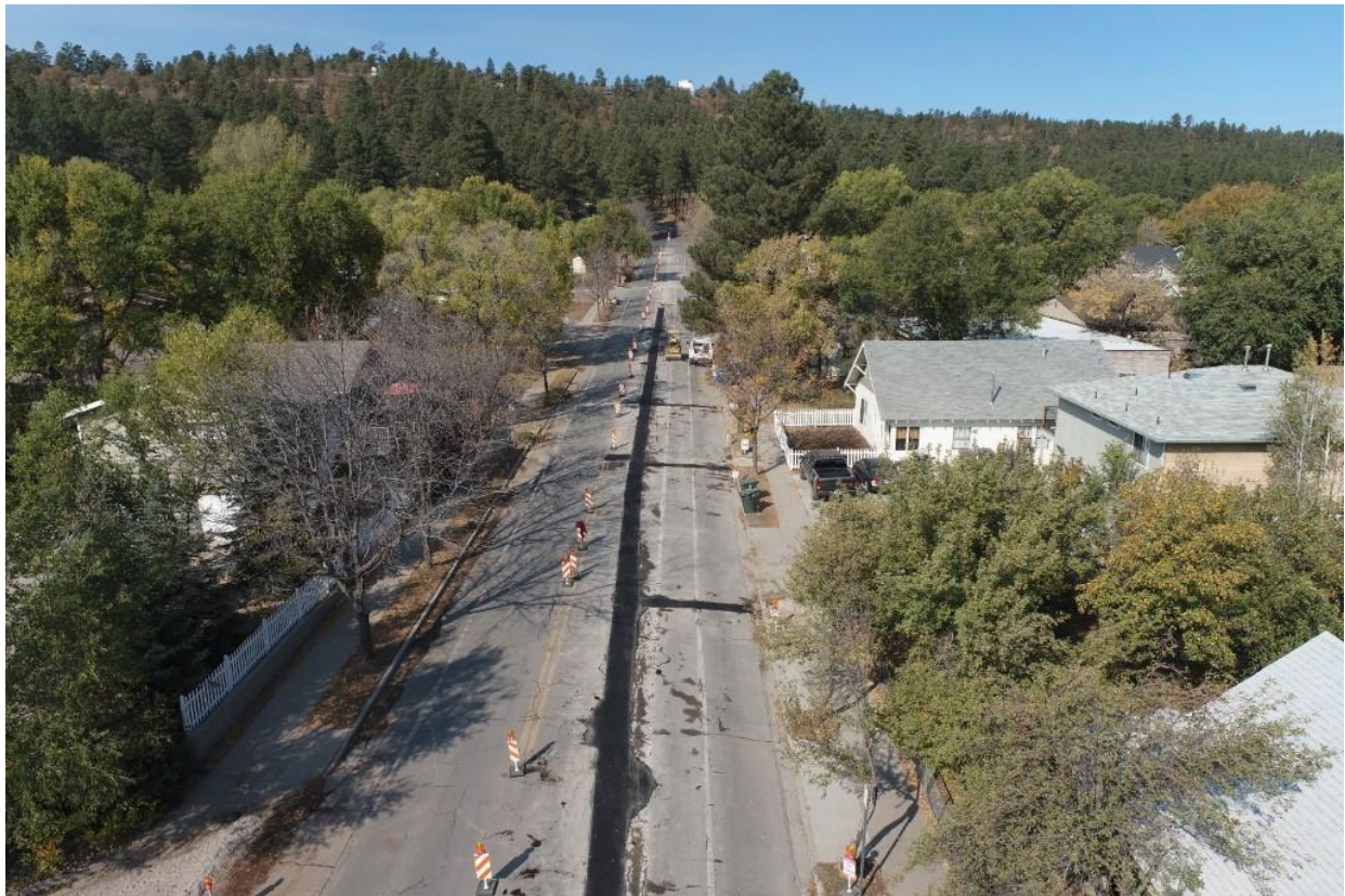
Summit Water Project-Trench patching on Santa Fe Avenue
