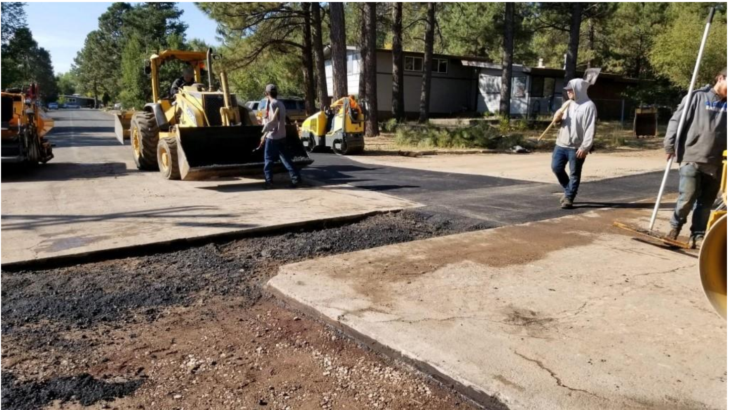
Pavement replacement at Marion Drive and Fir Avenue
