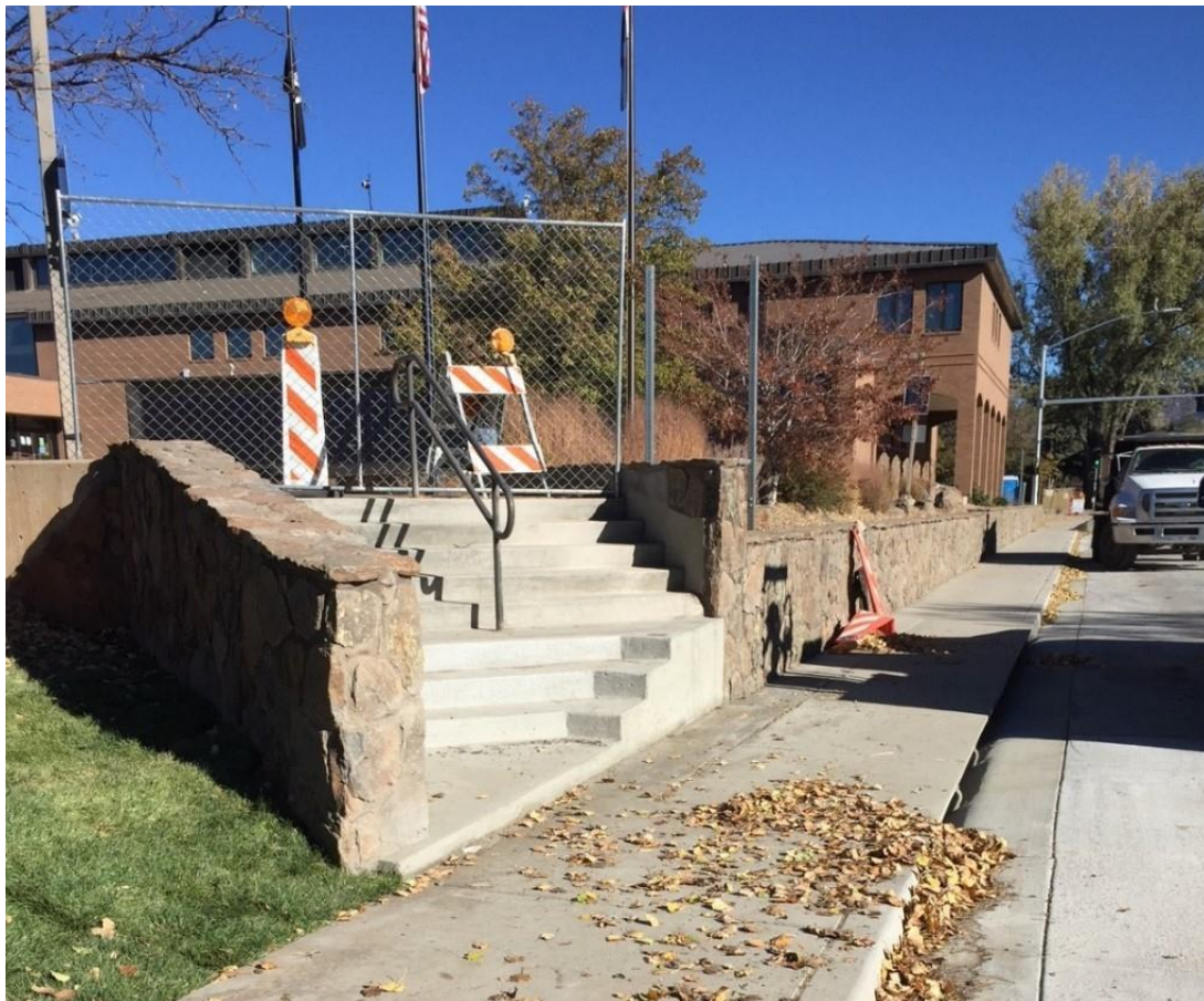
New stairs at southeast corner of City Hall (handrail forthcoming)
