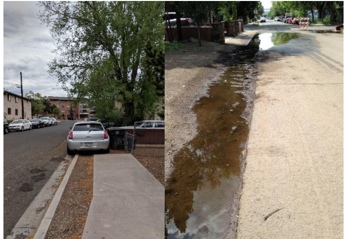
Figure 16: Incomplete street infrastructure in the Southside contributes to parking issues
