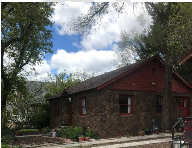
Figure 9: Vernacular malpais house on Cottage Avenue
