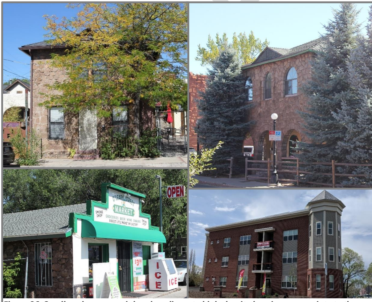
Figure 36: Small-scale commercial and medium- to high-density housing appropriate to the Live/Work Neighborhood subarea
