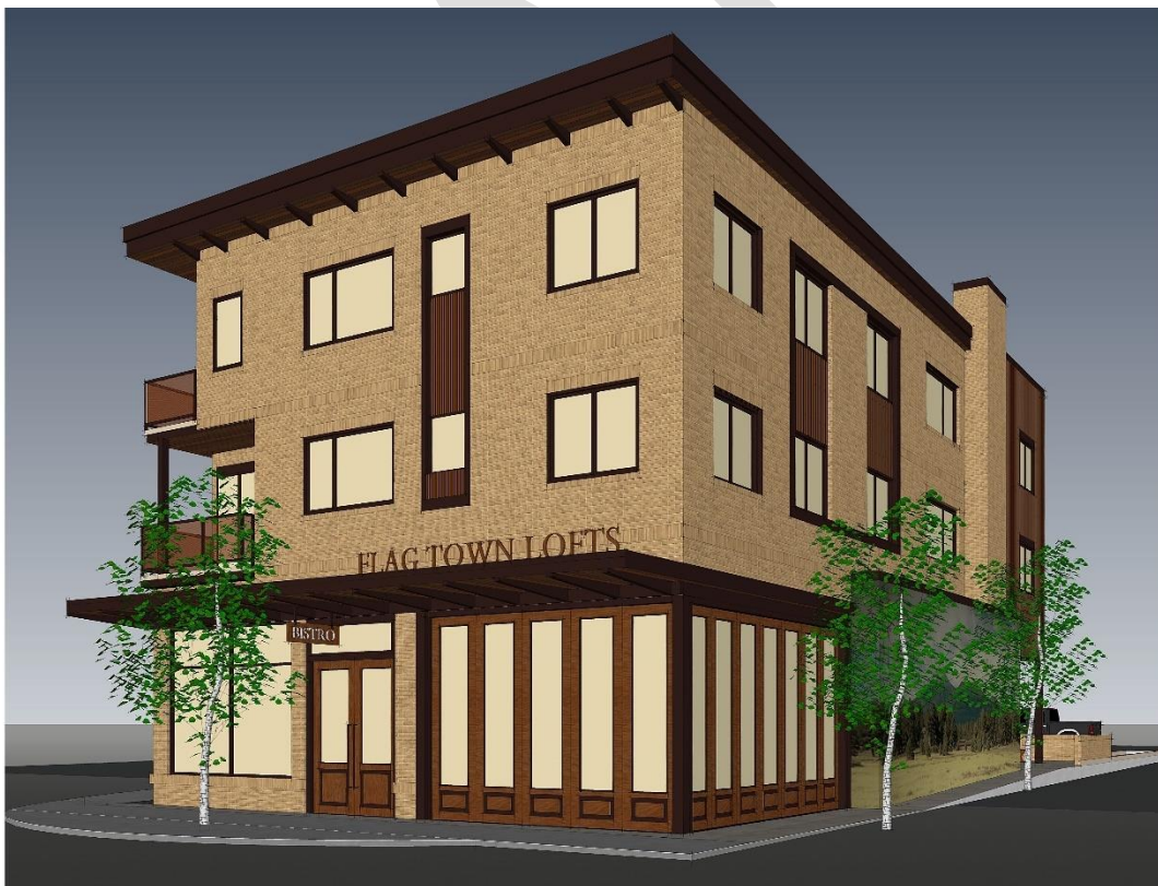
Figure 31: Building elevation for Flag Town Lofts, a new mixed-use building under construction at East Benton Avenue and South San Francisco Street (Designed by Updesign Studio)
