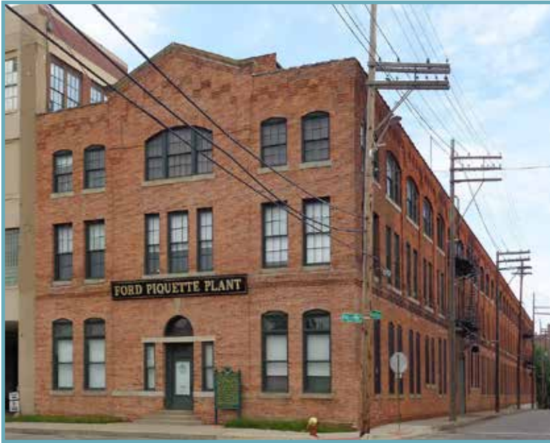
Old Ford Motors factory (photo credit: Jackdude101 via Creative Commons, creativecommons.org/licenses/by-sa/4.0/deed.en , no alterations were made)
