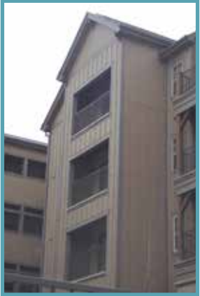
Wood siding (or a wood composite pre-primed and painted siding) placed horizontally and lapped vertically with batton joints
