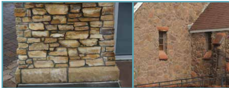
Rustic stone, Malpais basalt and stacked stone, “Flagstaff Vernacular”
