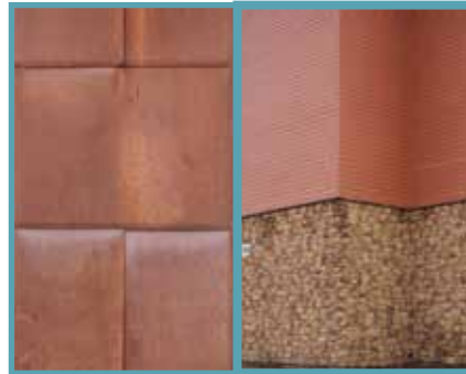
Metal shall be panels of 6" plus face with folded or standing seams. Corrugated galvanized metal is not allowed.
