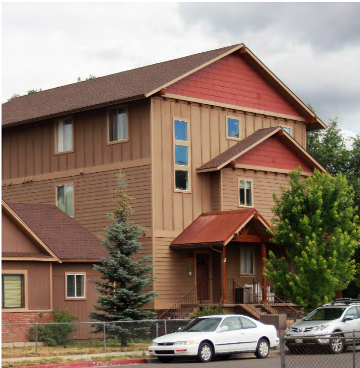
Figure 7: New duplex on South Leroux Street
