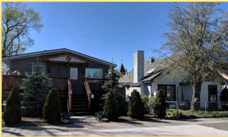
A conforming (left) and nonconforming structure (right) on South Humphreys Street
