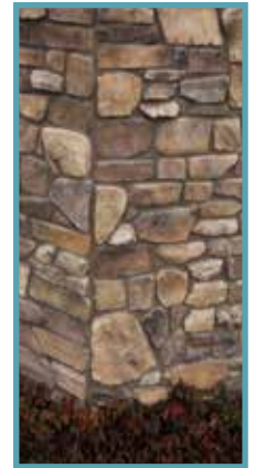
Cultured stone or fake stone (replicated stone that simulates a stone’s quality and durability)
