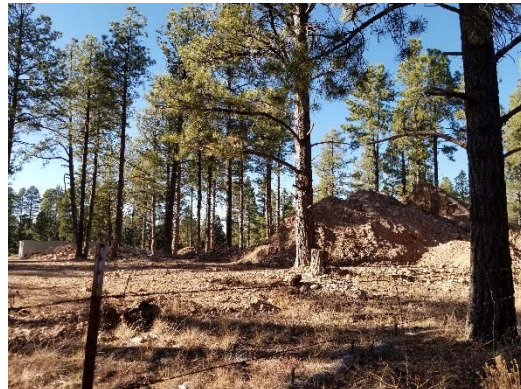
Picture 40 - West-adjacent building materials near corner 6 of Property, along western edge
