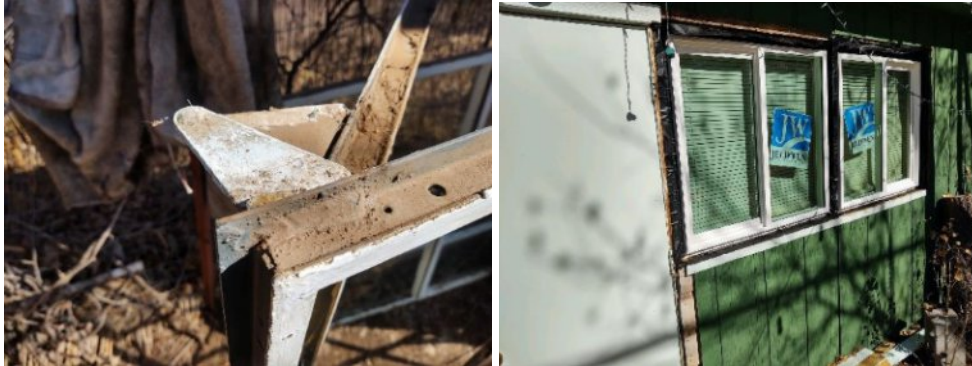
Original metal window hardware detail out-swing casement
