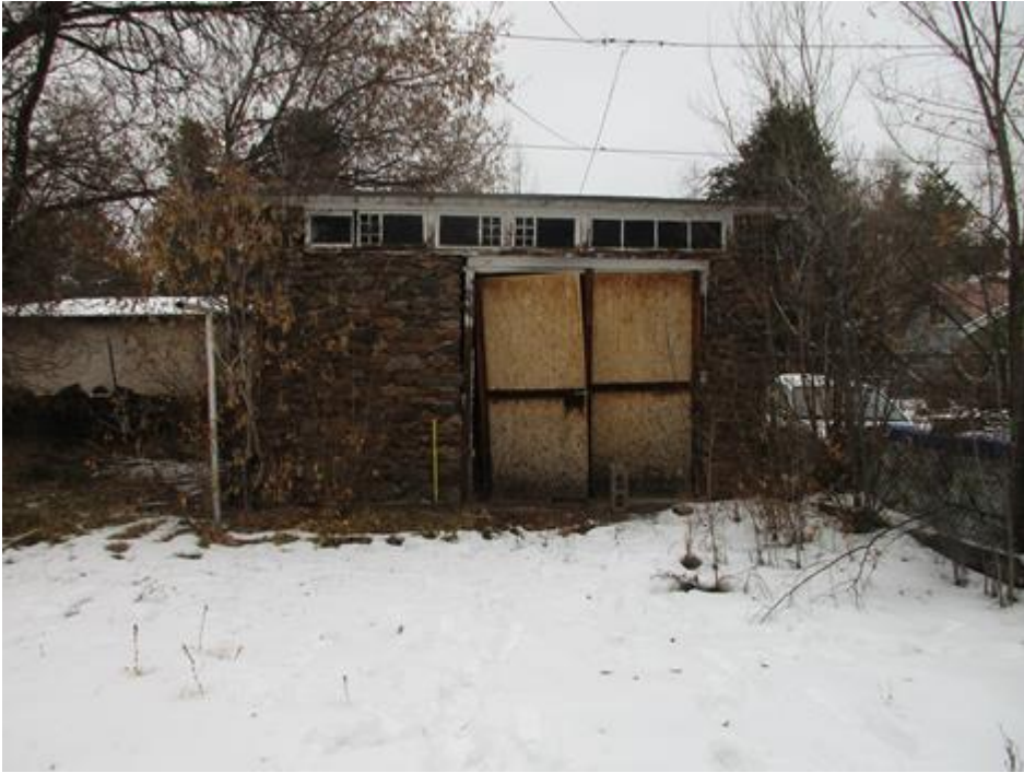
Garage - current conditions
