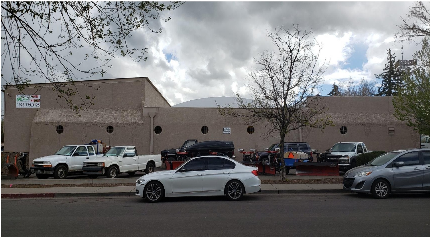
14 S Leroux St south façade overview from Cottage Avenue, May 2019.
