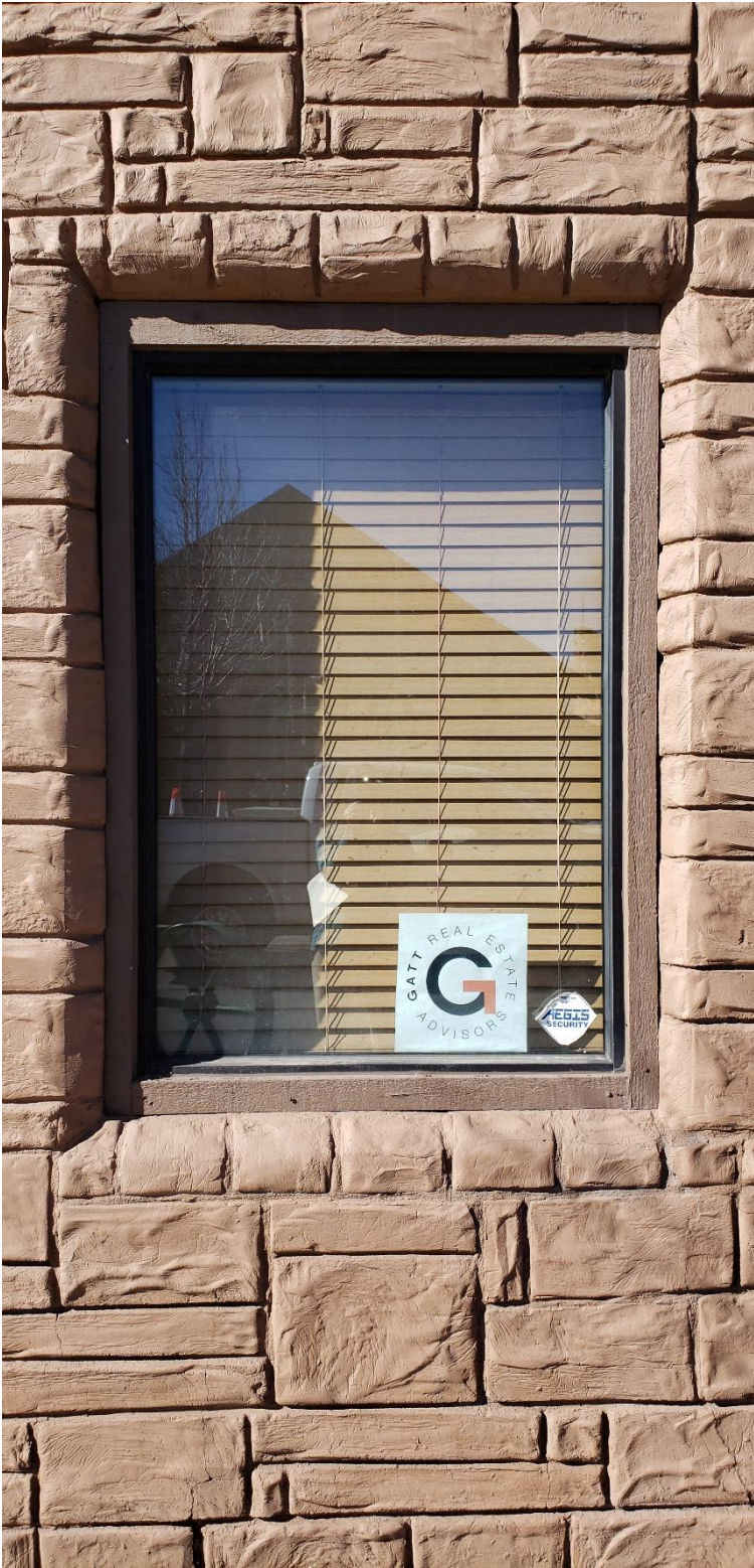
Example of concrete plaster sheathing on 43 S San Francisco's front/E façade (left) & at NE corner (right), December & May 2019.
