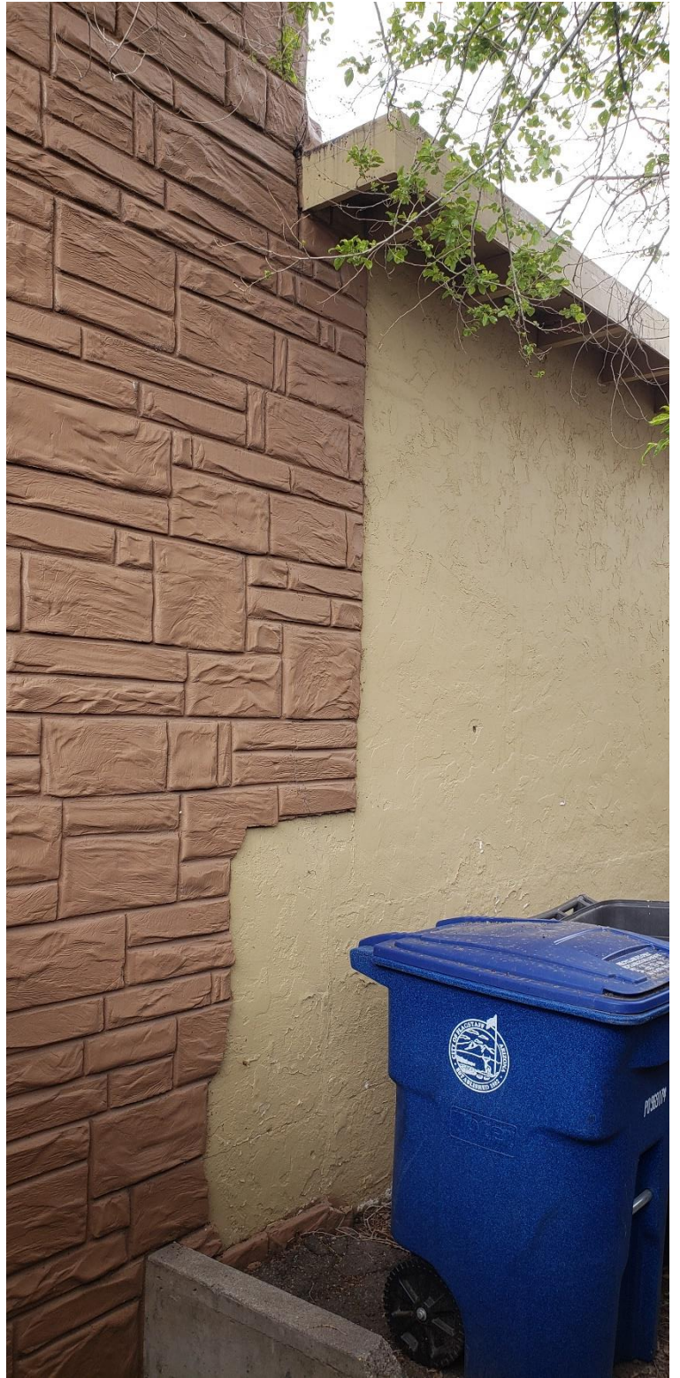
Example of concrete plaster sheathing on 43 S San Francisco's front/E façade (left) & at NE corner (right), December & May 2019.
