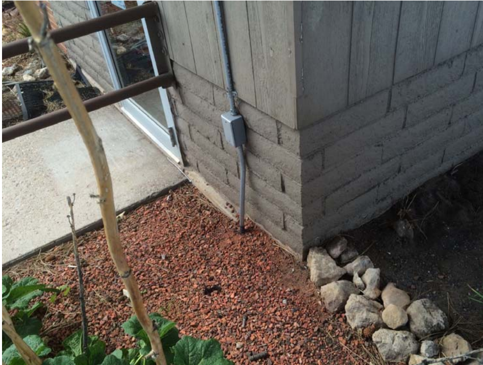
Figure 12. Detail photograph of the southeast corner cinderblock brick dado and concrete continuous spread foundation of the ADOT Flagstaff District Office.
