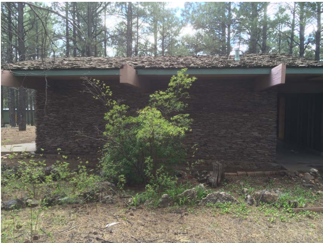
View of schist-walled eastern elevation of the garage on southern end of property, facing west.
