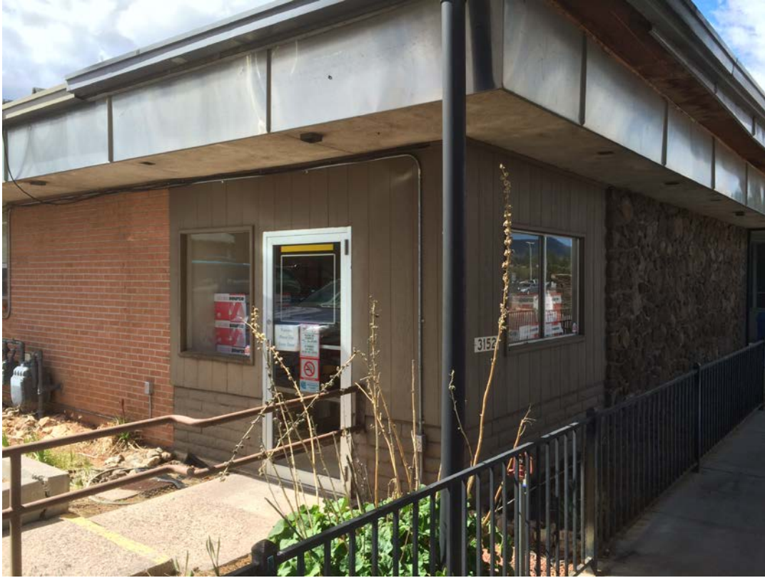
Photo of the remodeled southeastern corner of property, facing northwest.
