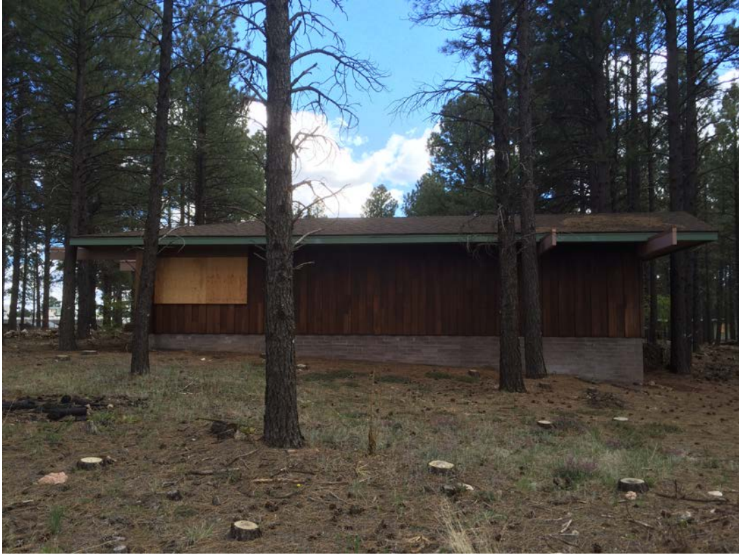
View of the northern elevation of the property, facing south.
