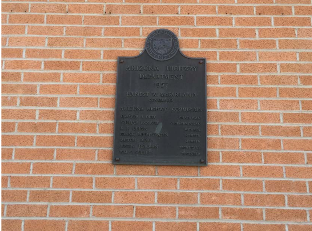
View of the plaque on the eastern elevation north of the public entrance.
