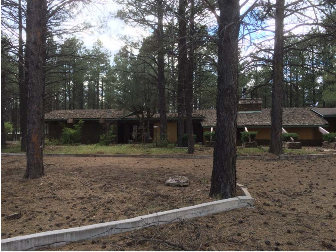
View of the southern portion of the eastern elevation of the property, facing west.
