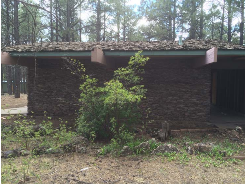
Figure 28. Photograph of the east elevation of the garage showing the masonry schist wall, facing west.
