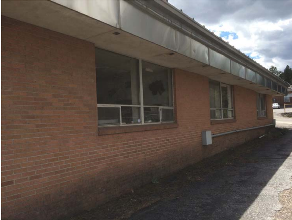
Figure 15. Photograph of the northern elevation showing the fascia, soffit, wall, and windows.
