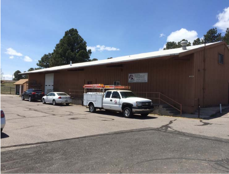
Figure 22. Overview of the facilities office/maintenance building, facing southwest.
