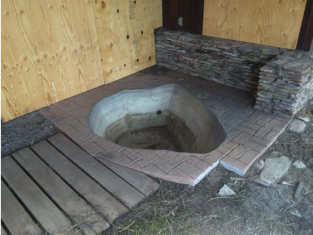
View of an outdoor concrete tub on the eastern side, south of the central living area, facing northwest.
