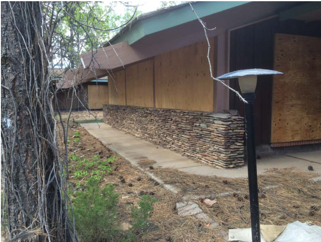
View of central portion of the western elevation of property, facing north-northeast.
