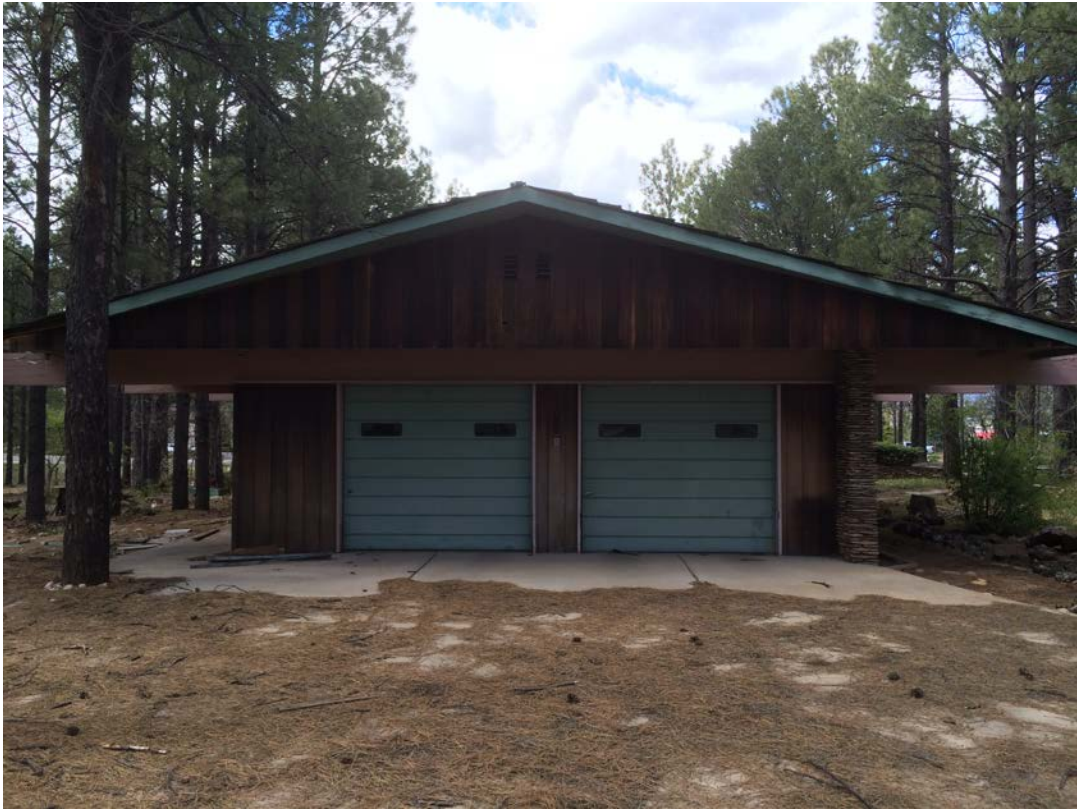
View of the southern elevation of the property (garage doors), facing north.
