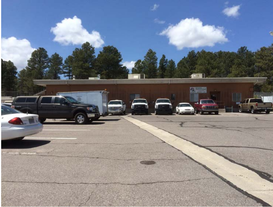
Figure 21. Overview of the materials lab, facing west.
