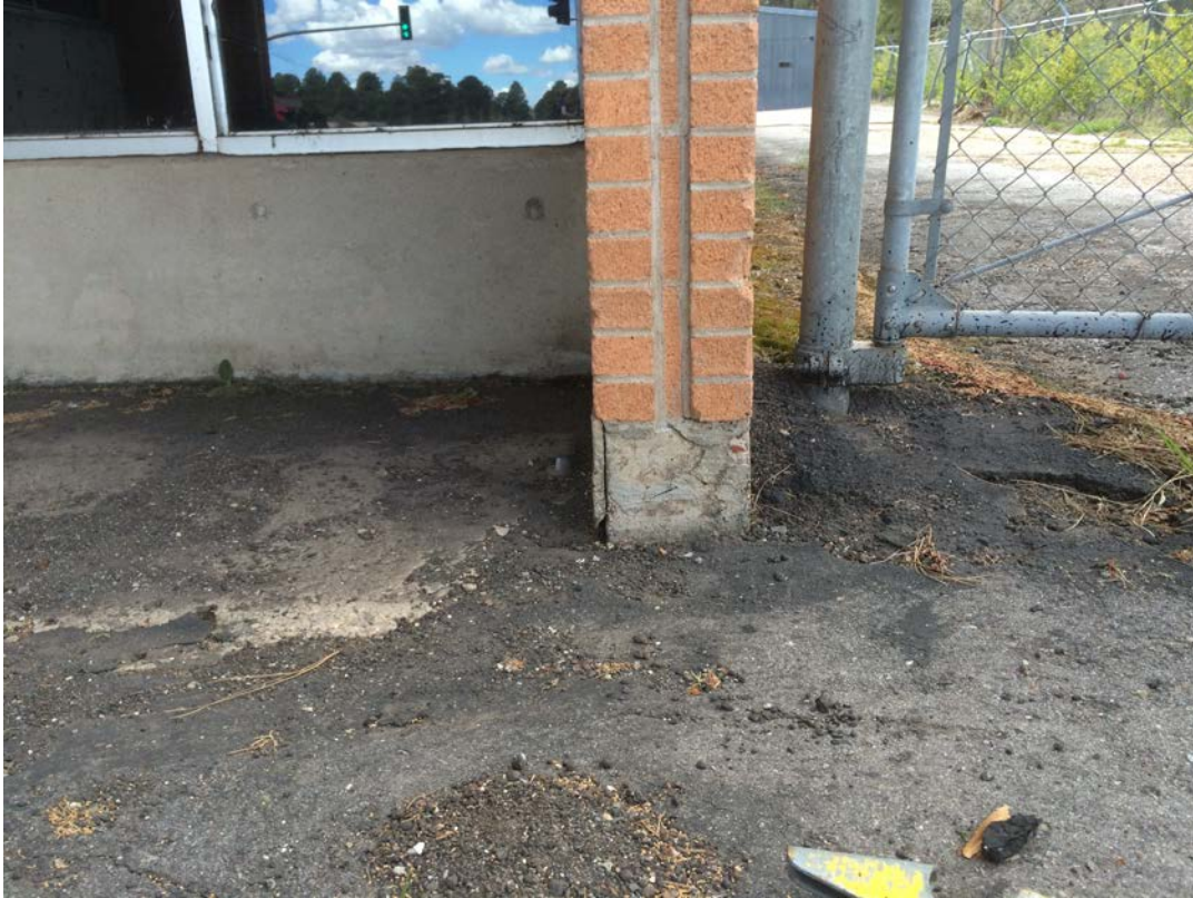
View of continuous spread concrete foundation on north wall, facing west.
