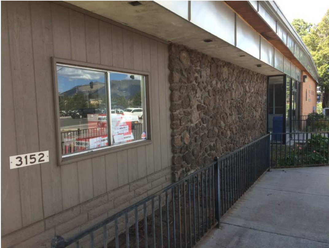
View of the eastern elevation of the property, facing north-northwest.
