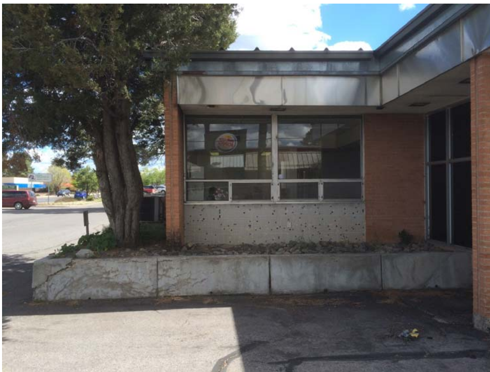
Figure 14. Photograph of the recess on the northeastern corner of the building showing the tile mosaic.
