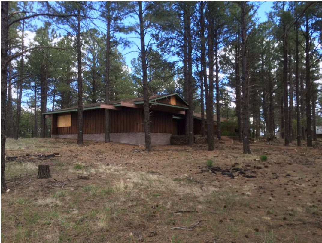
View of the northern and western elevations of the property, facing southeast.
