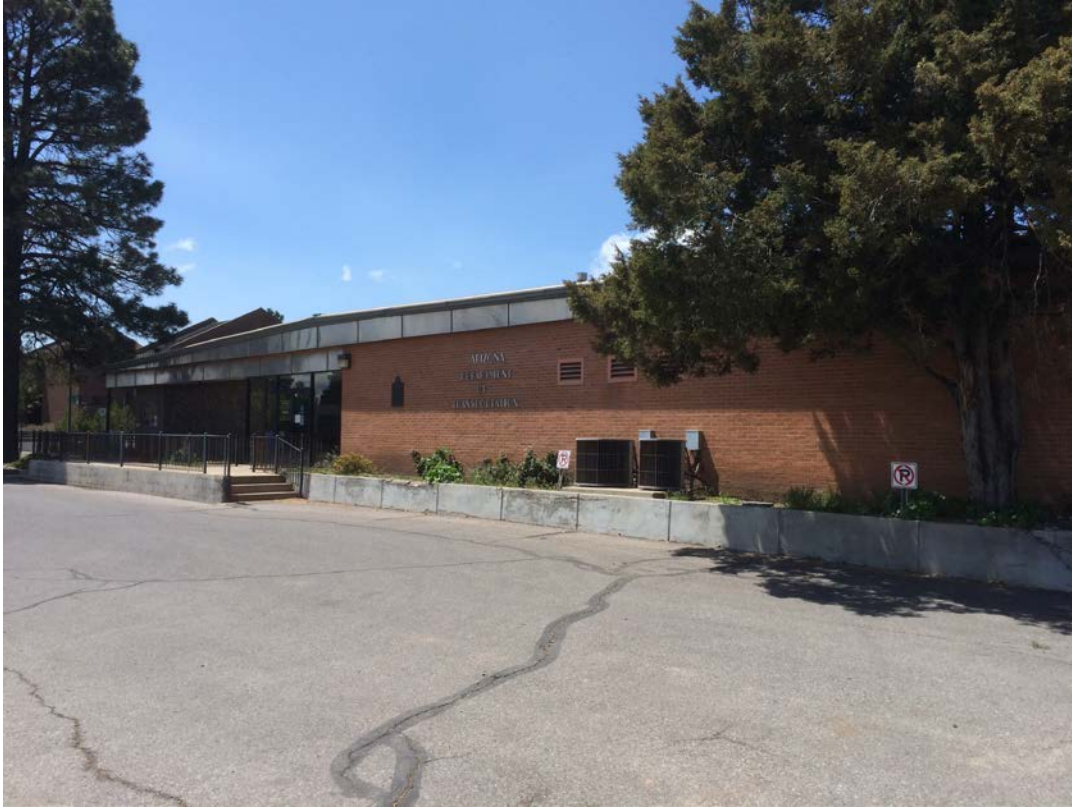
View of eastern elevation of the property at 1801 South Milton Road, photo facing southwest.
