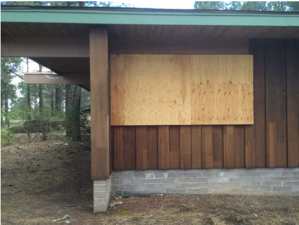
Figure 32. Photograph of the northern elevation of the residence showing the cinderblock brick foundation, facing south.
