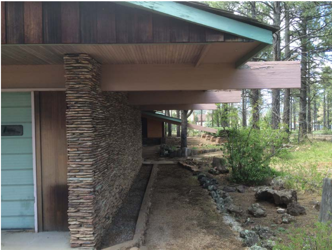
View of eastern elevation of property, facing north.
