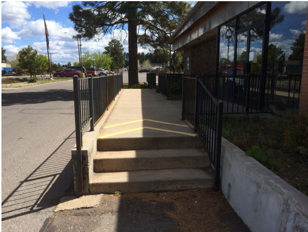
View of the front entrance to the property including steps and ramp, facing south.
