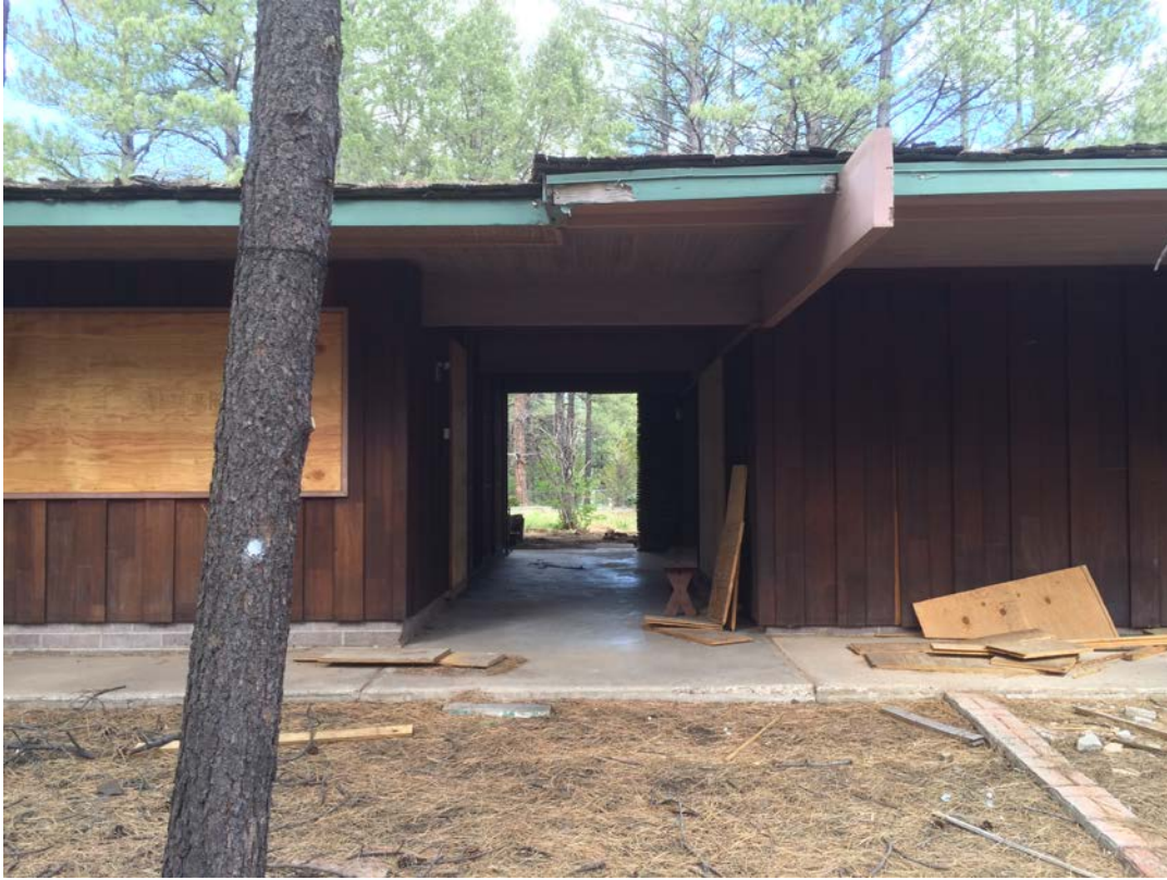
View of the breezeway, facing east.
