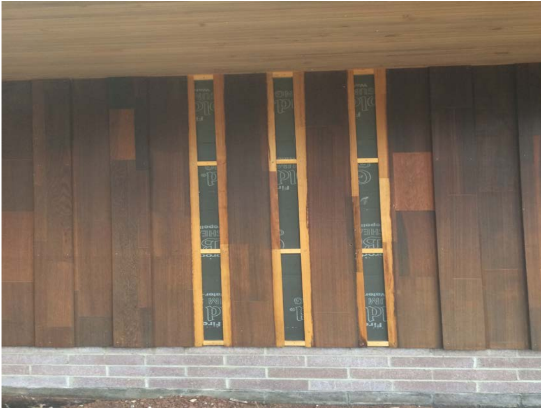
Detail of wall construction along northern end of eastern elevation, photo facing west.
