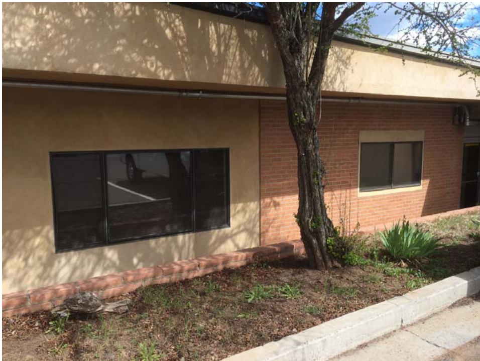
Figure 18. Photograph of the western elevation showing the original brick wall on the right and the later stucco wall on the left.
