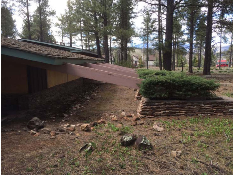
Figure 29. Photograph of the beams and planters on the east side of the residence, facing north.
