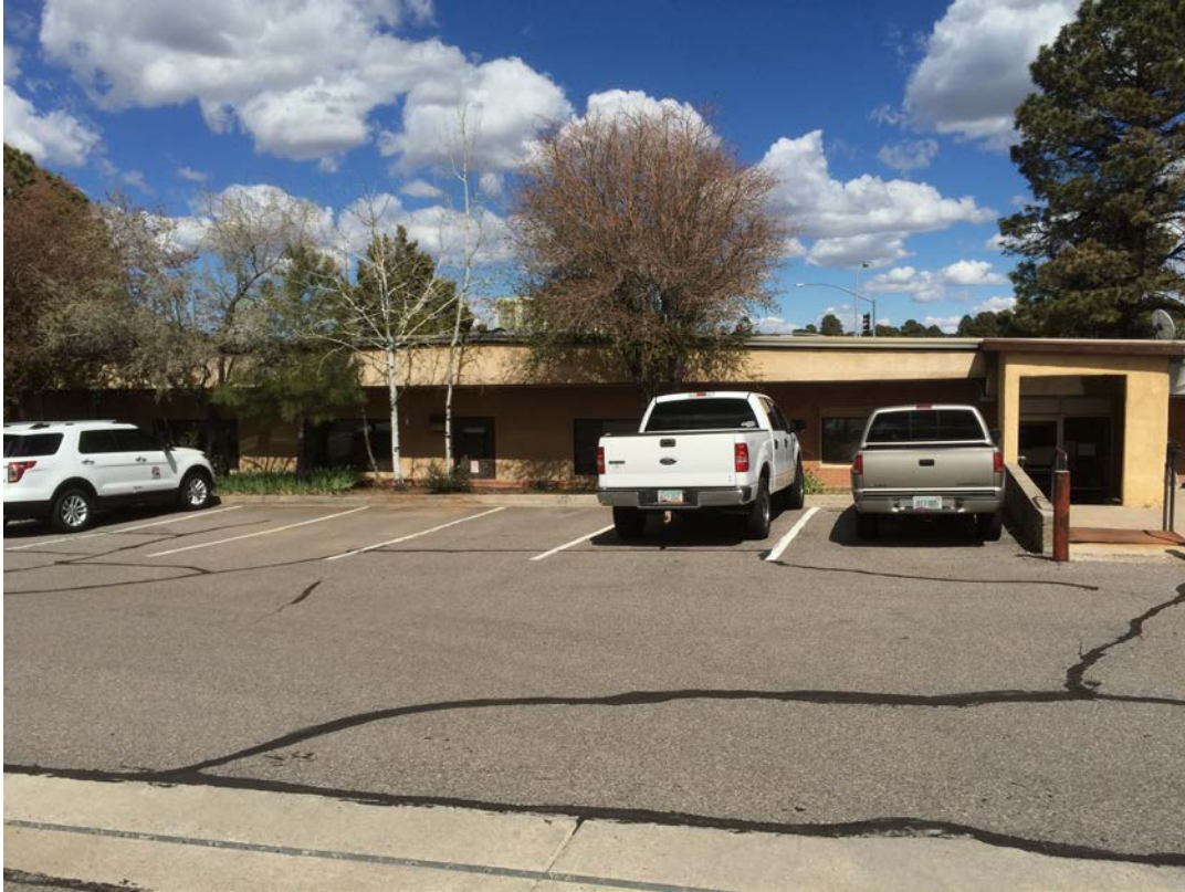
View of western elevation of property including remodeled area, photo facing east.
