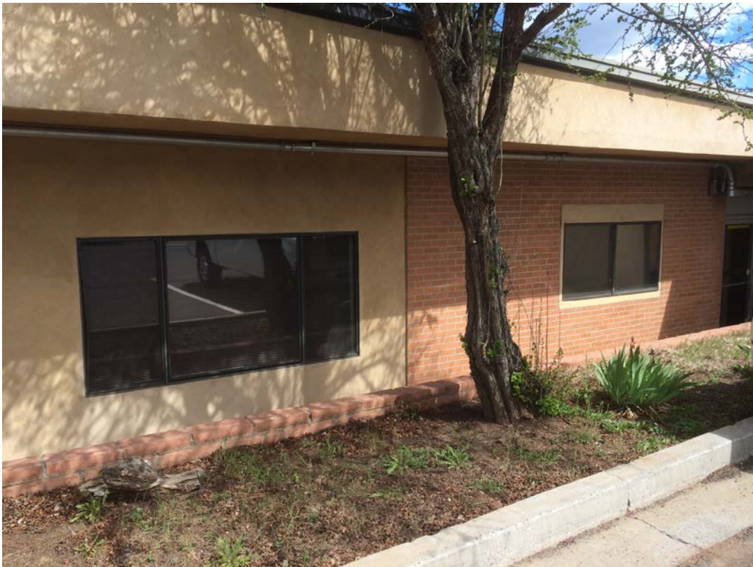
View of southern portion of the western elevation showing differential walls, facing southeast.
