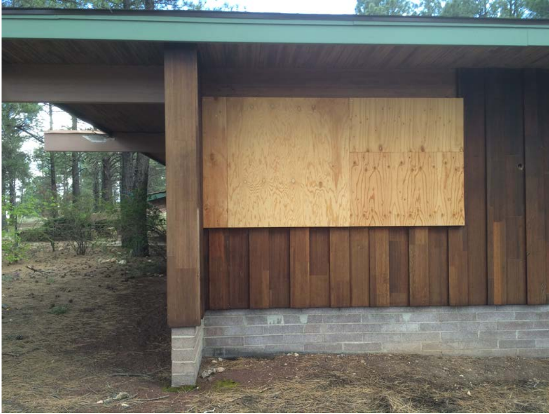
Detail of the foundation, walls, windows, and fascia on east end of north elevation, facing south.
