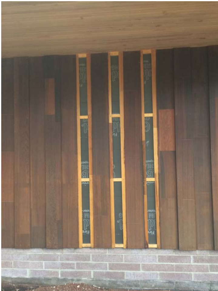
Figure 27. Photograph of a wall section of the primary residence (east elevation), facing west.
