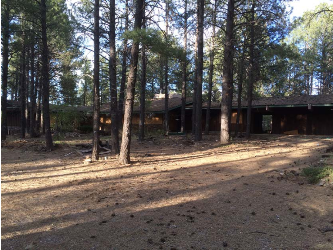
View of the western elevation of the property partially obscured by trees, facing east-northeast.
