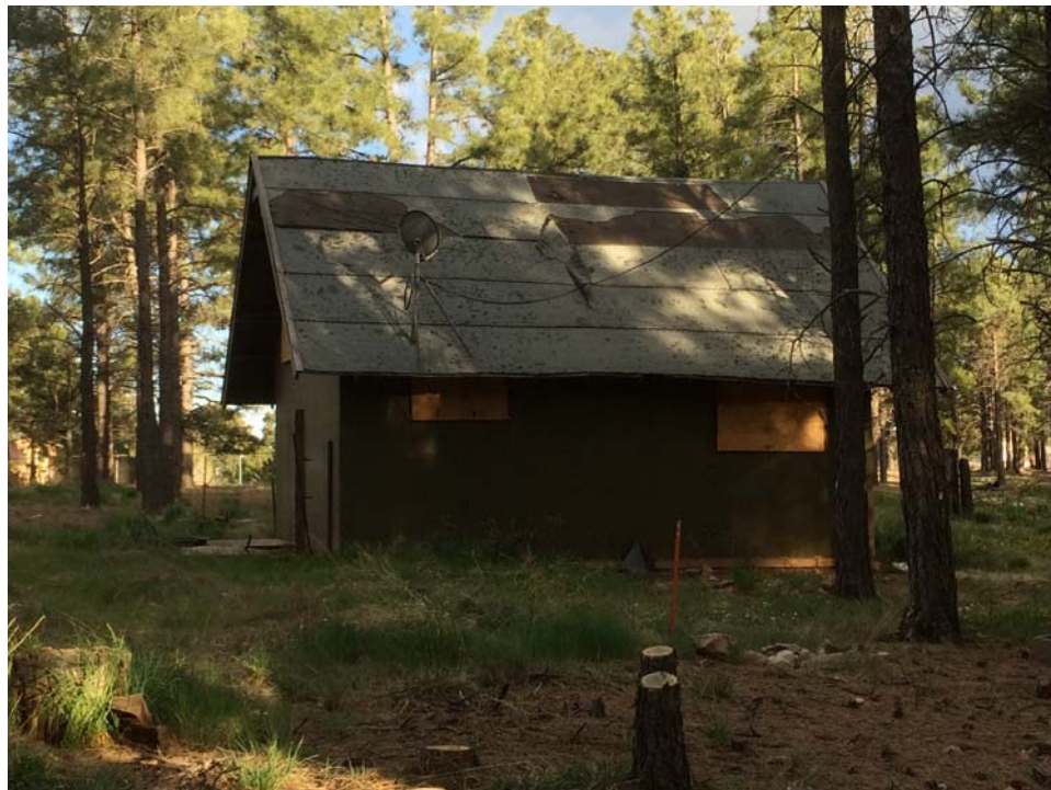
Figure 36. Overview of the barn at 701 West University Avenue, facing southeast.
