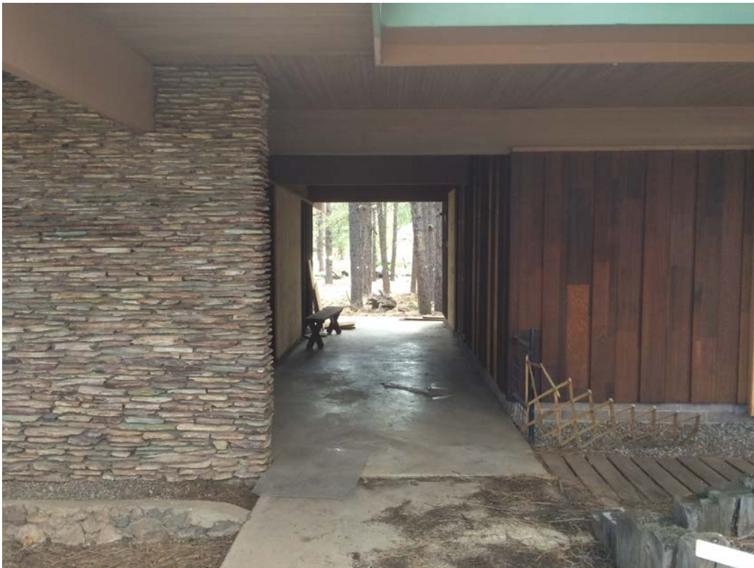
View of the breezeway, facing west.
