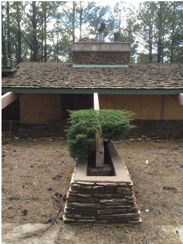
Figure 30. Detail photograph of the schist masonry-lined planters, facing west.
