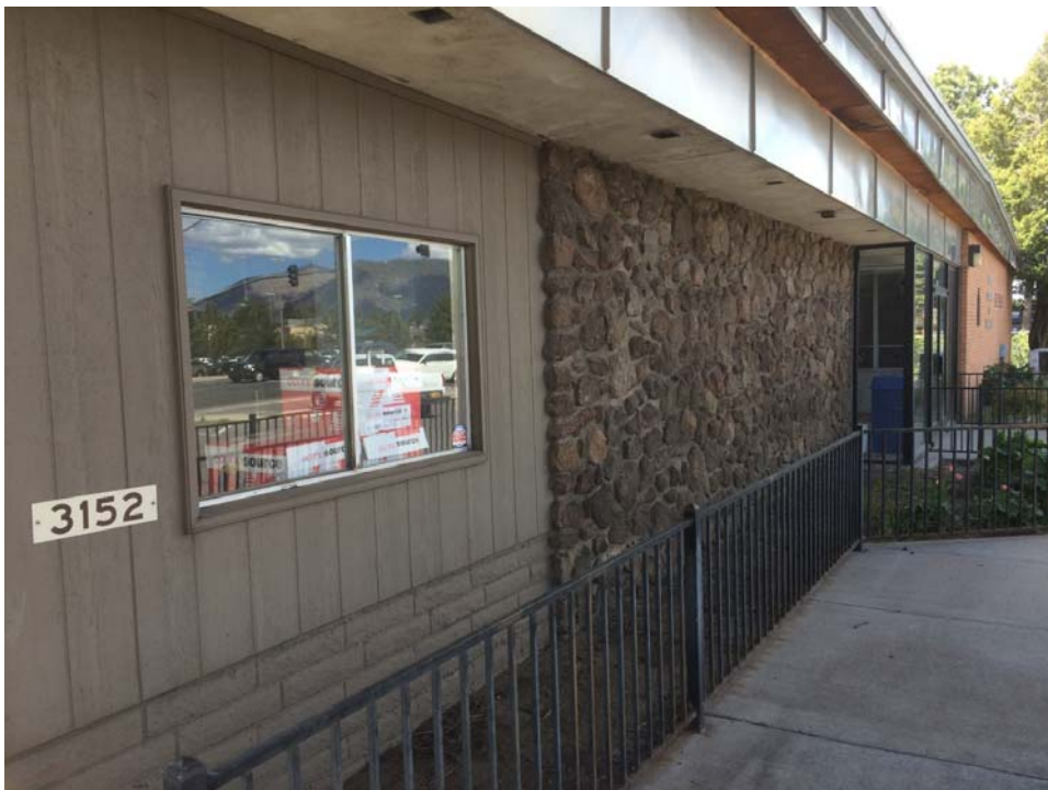
Figure 13. Photograph of the eastern elevation of the structure, facing north-northwest.
