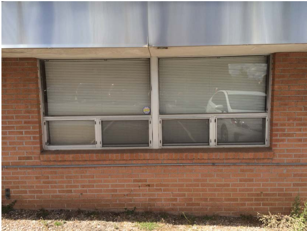
Photograph of original windows on the south elevation, photo facing north.
