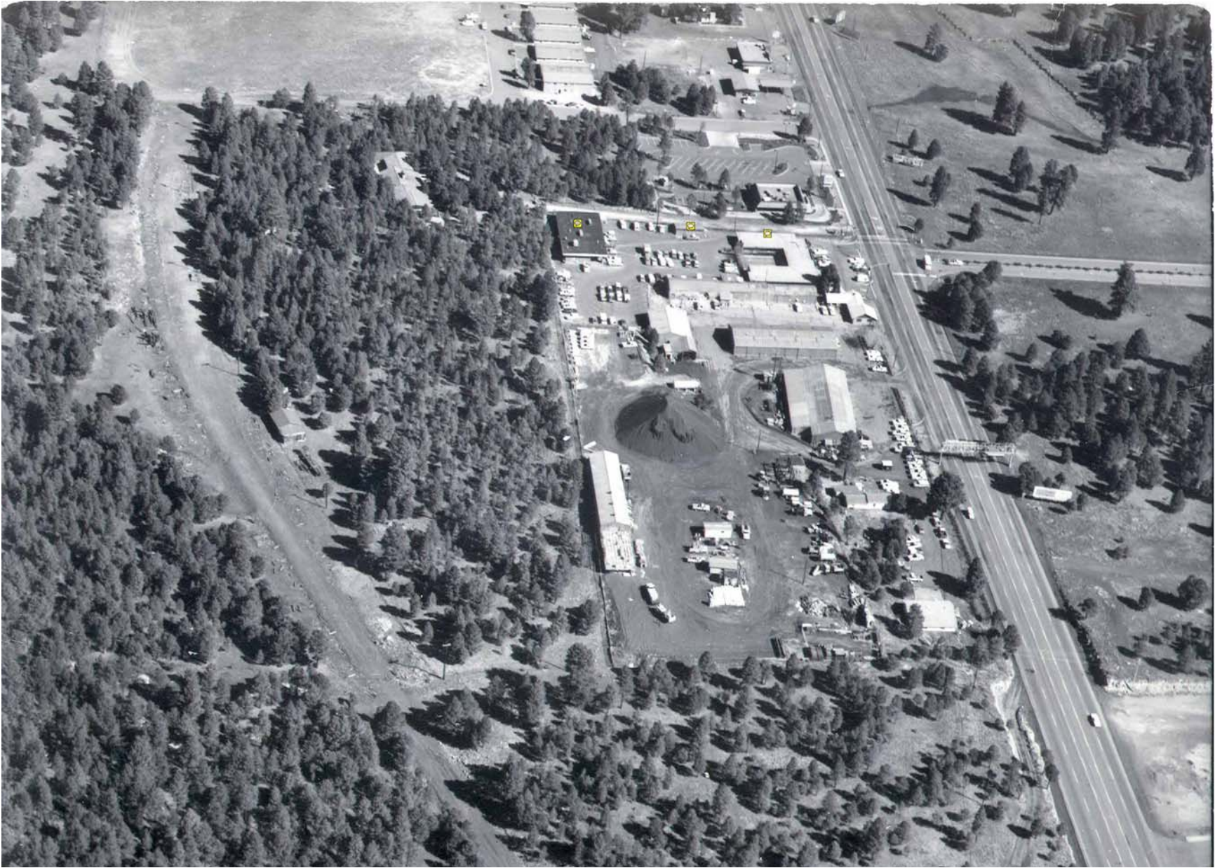
Figure 9. Aerial photo (ca. 1975) showing the project area and ADOT buildings.
