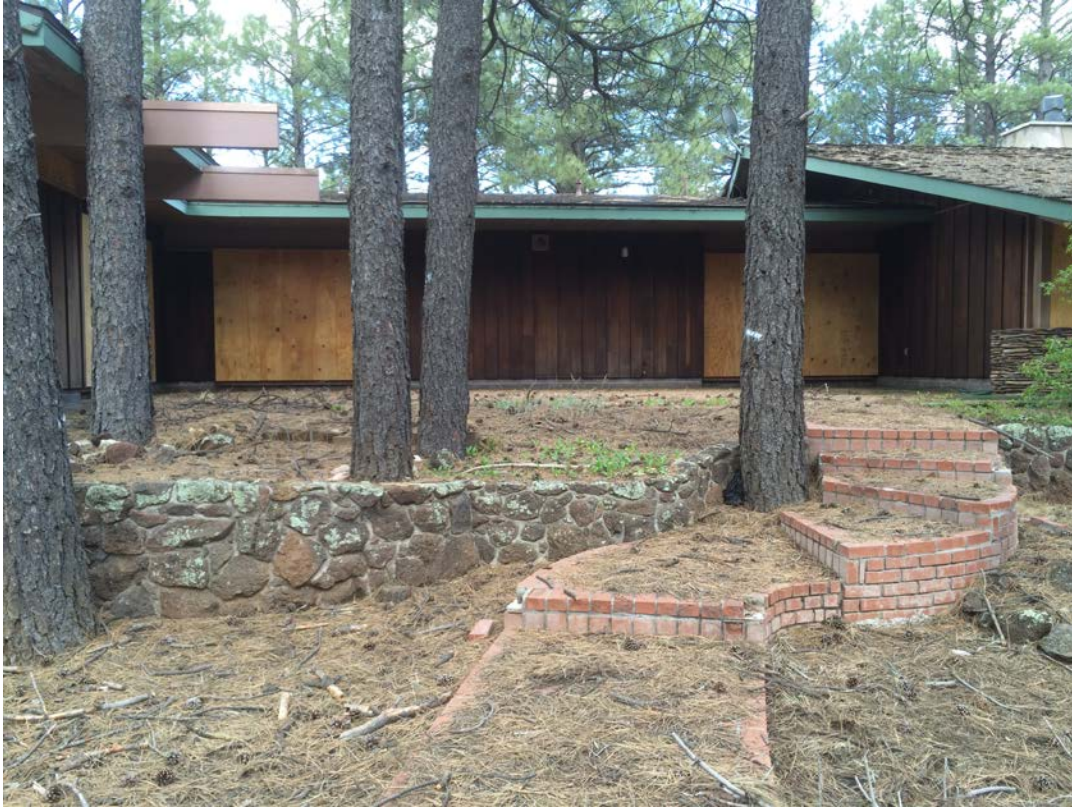
View of the central portion of the north wing on the west elevation, facing east.
