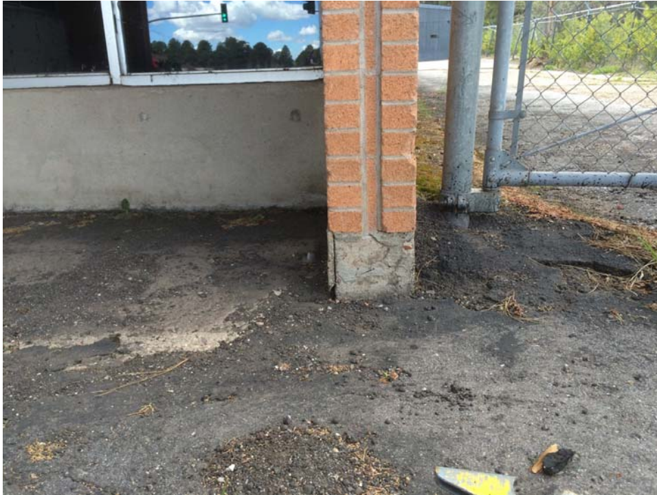
Figure 17. Photograph of concrete foundation and brick wall of the northeast corner of the structure (eastern elevation), facing west.
