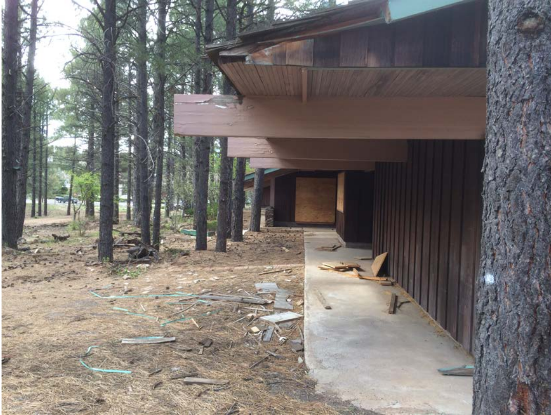
View of western elevation of property, facing north.
