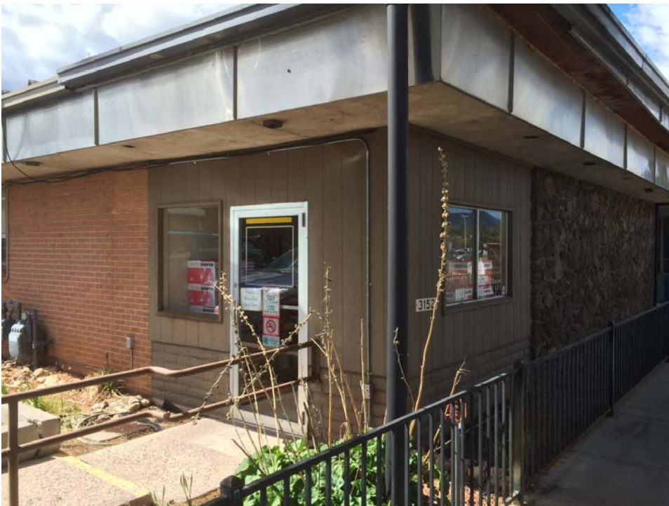
Figure 11. Photograph of the southeast corner of the ADOT Flagstaff District Office.
