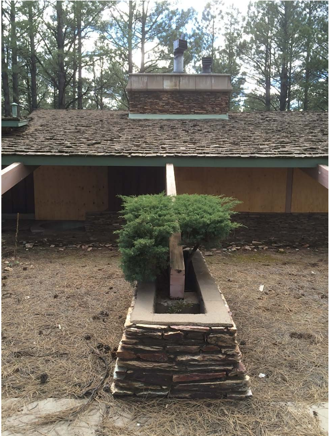
Detail of a roof beam and schist-walled planter on the east side of the house.
