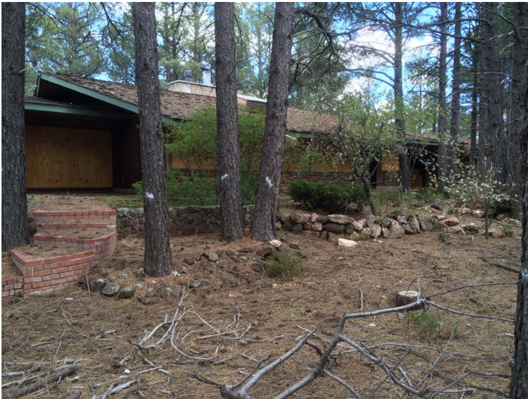
View of the western elevation of the property, facing southeast.
