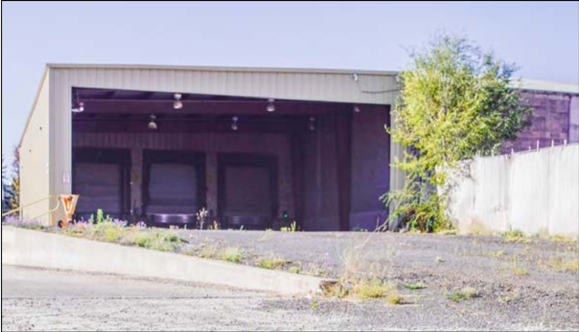
Figure 90. Photo of Building 1 truck bay, facing south.
