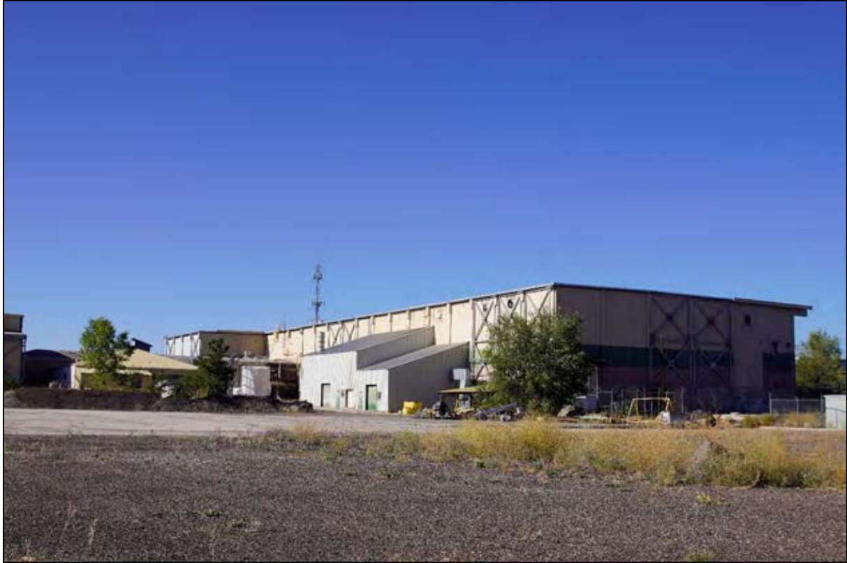
Figure 69. Photo of Building 3, facing southwest.
