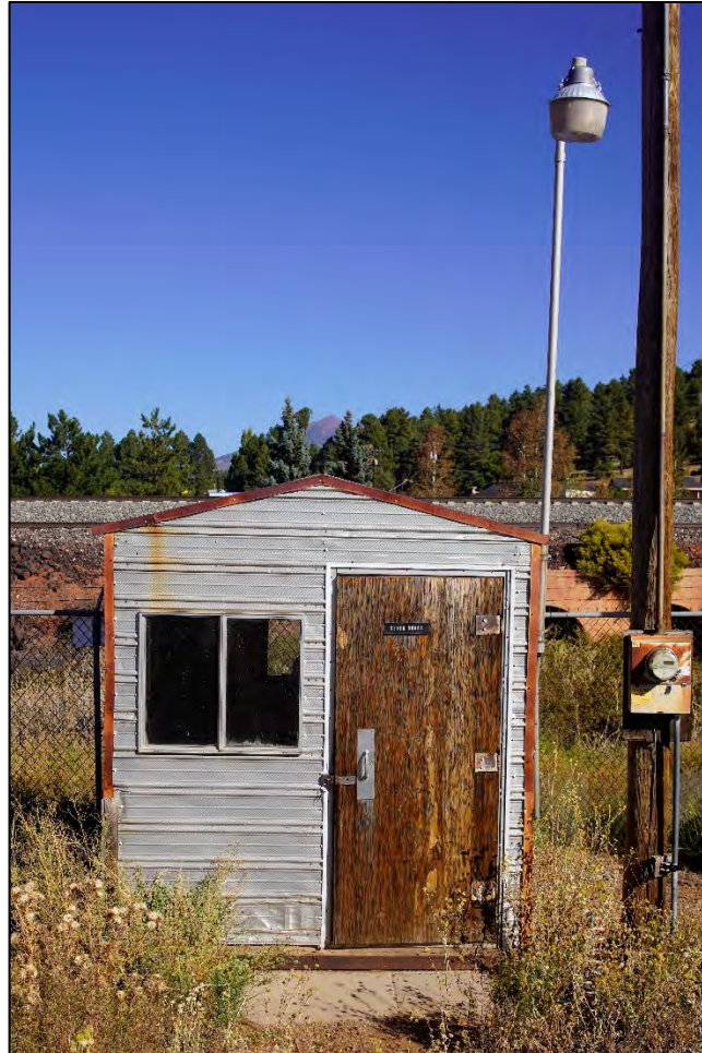
Figure 81. Photo of the Sewer Shack, facing north.
