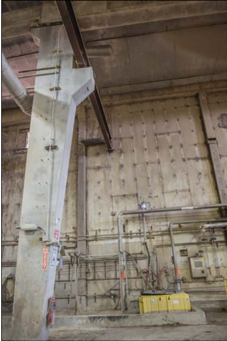
Figure 111. Building 3, tapered column detail.
