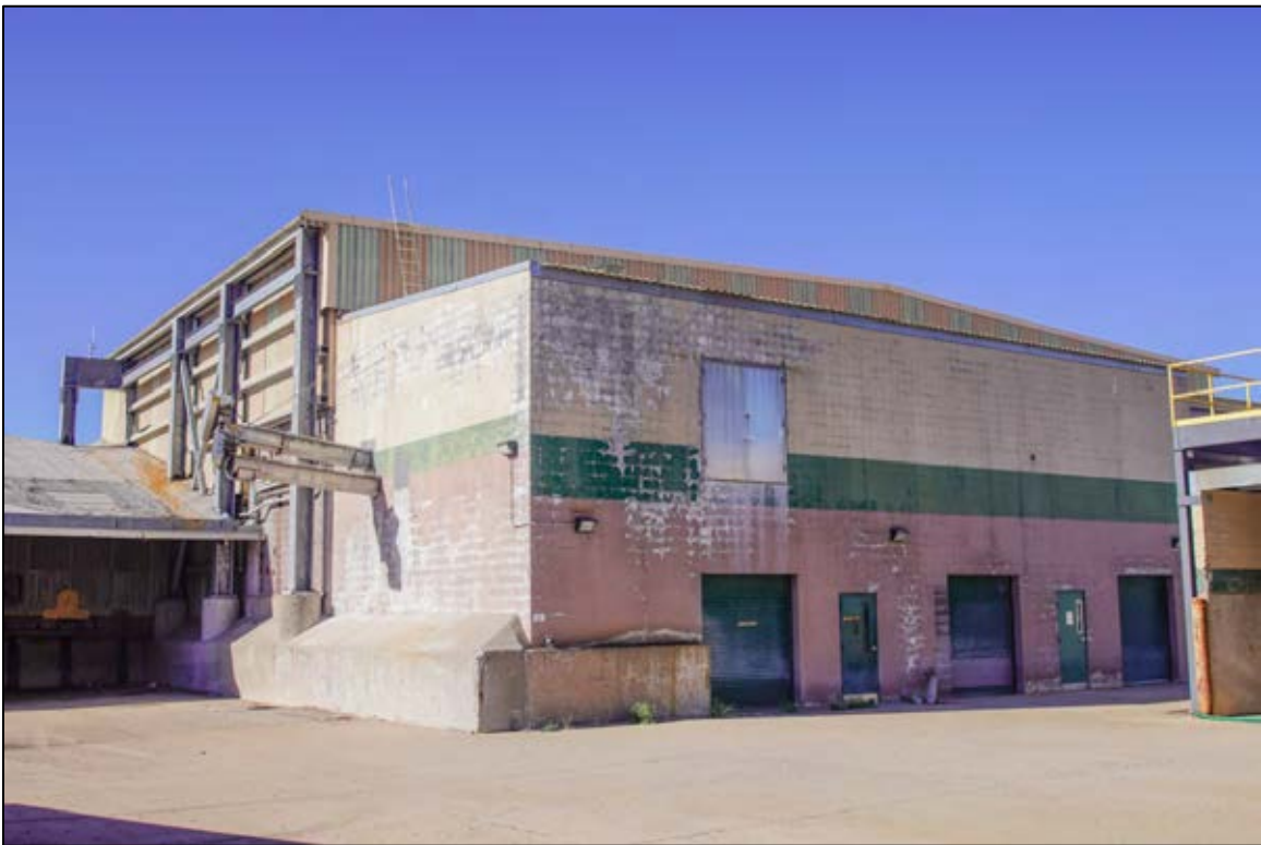
Figure 124. Building 6, north elevation.
