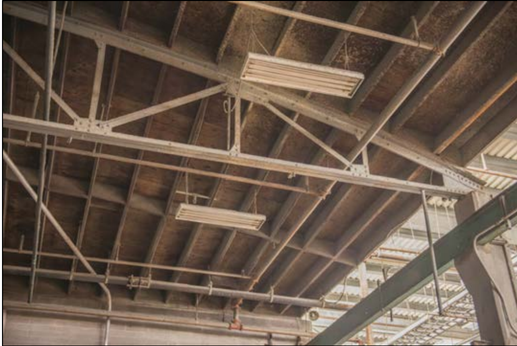
Figure 125. Building 6, bow truss detail.
