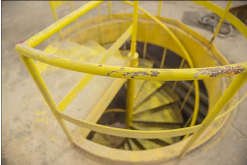
Figure 117. Building 3, circular stairs to basement.
