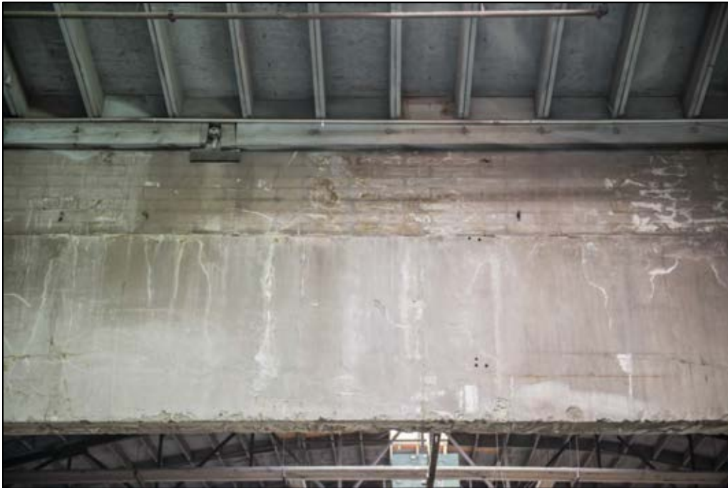
Figure 93. Building 1 CMU above concrete shear wall.
