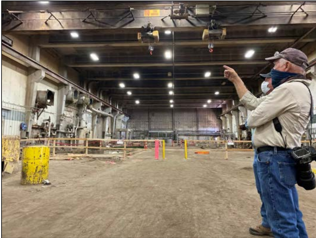
Figure 70. Photo of Building 3 interior, facing north-northeast.
