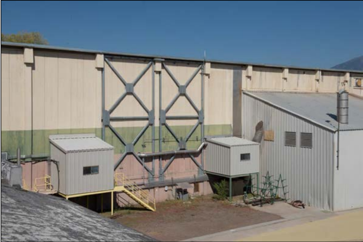
Figure 113. Building 3 braced frames, facing northwest.
