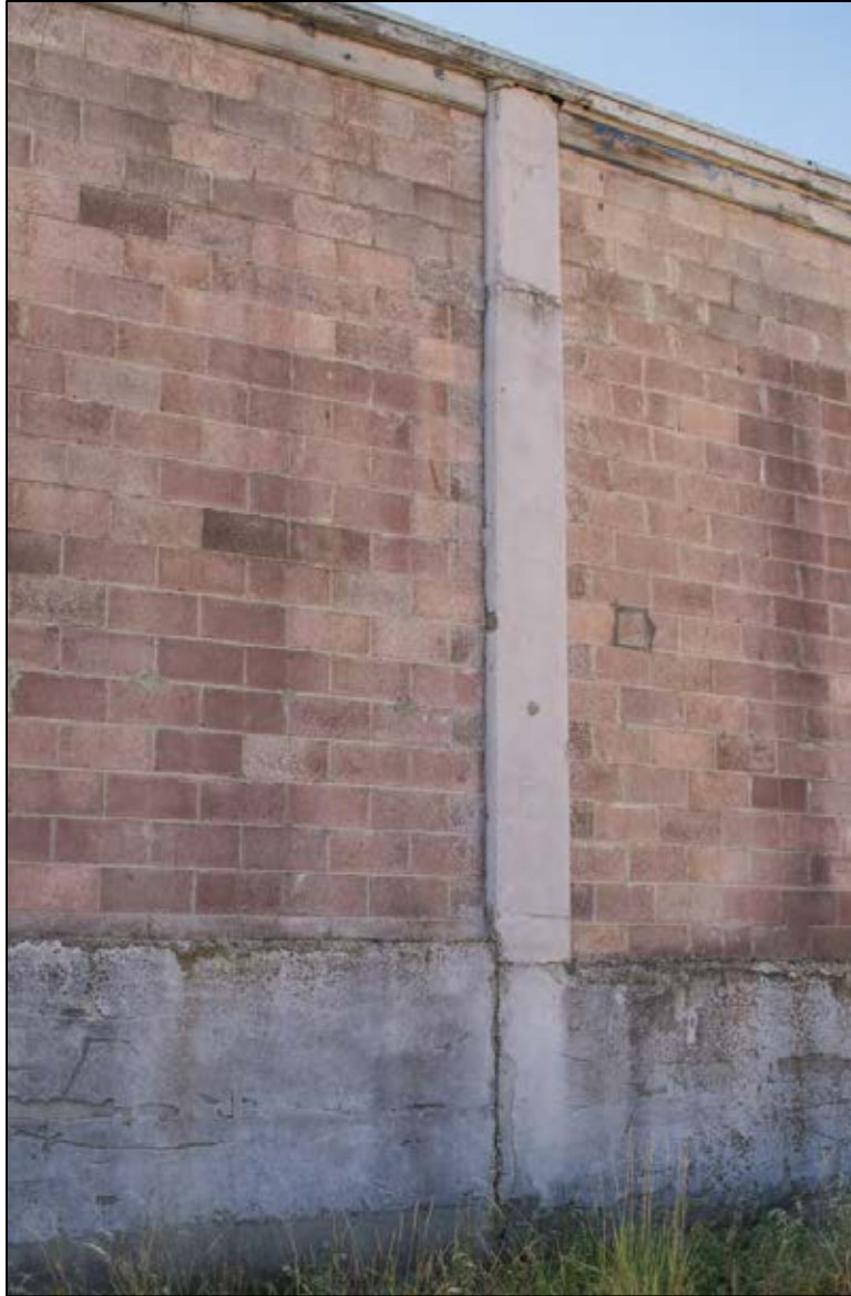
Figure 99. Building 1 exterior detail.
