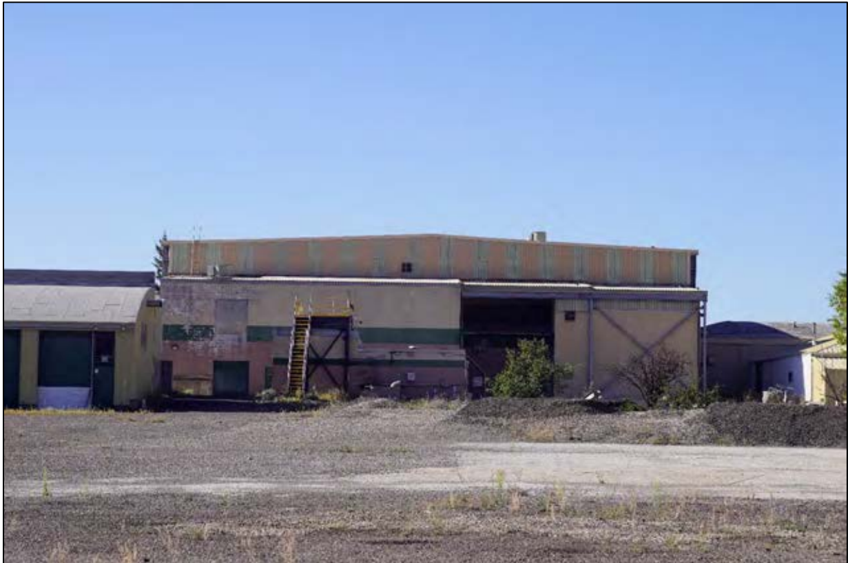
Figure 76. Photo of Building 6, facing south-southwest.
