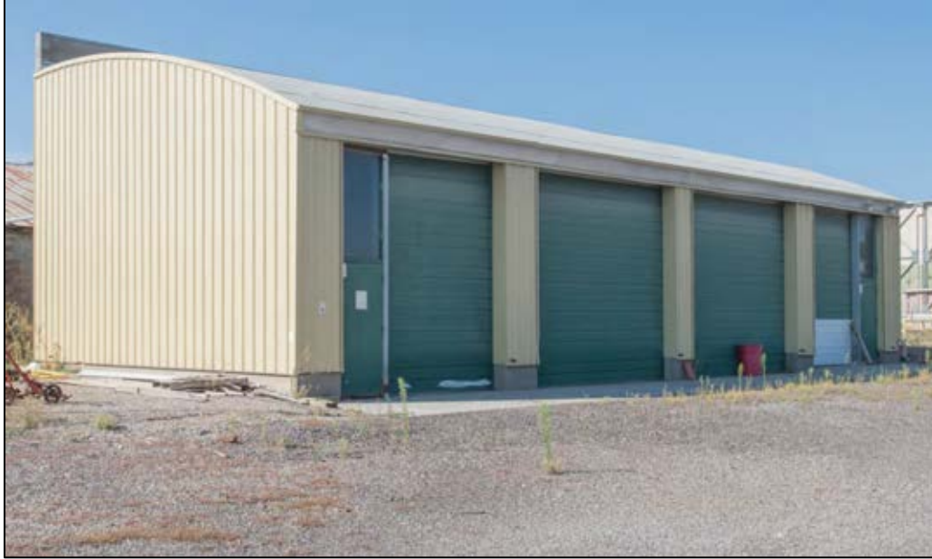
Figure 133. Building 10, facing west.
