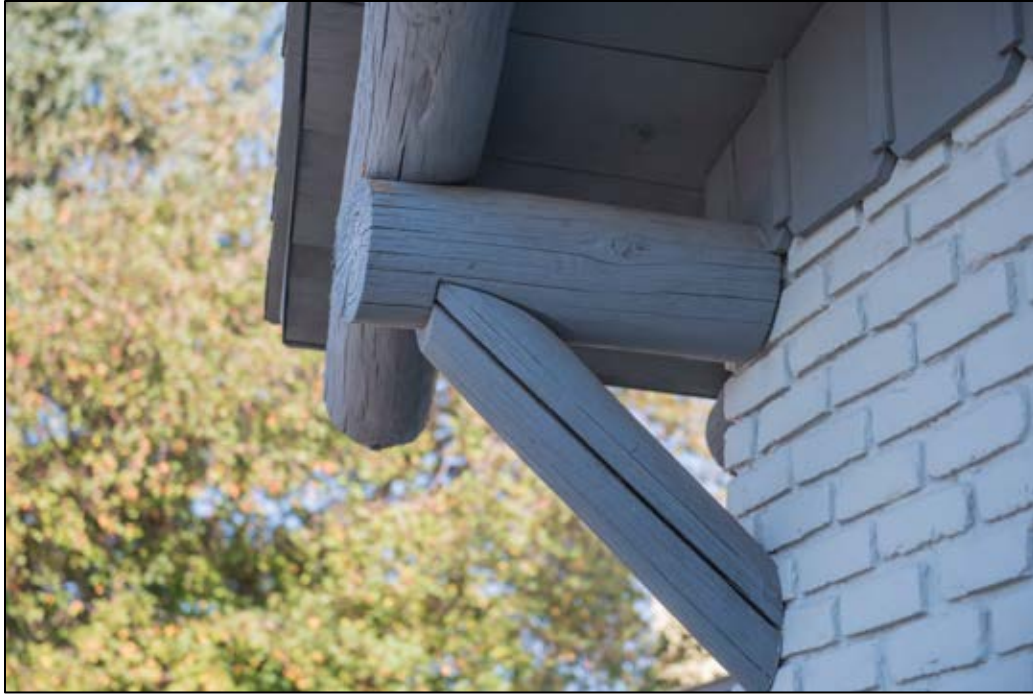
Figure 120. Building 4 roof detail.
