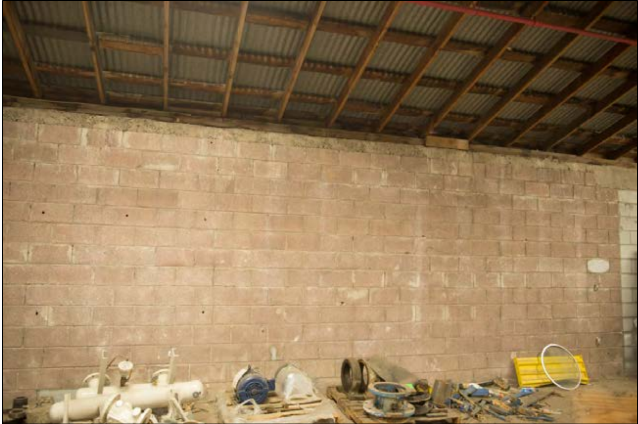
Figure 132. Building 8 interior bays.
