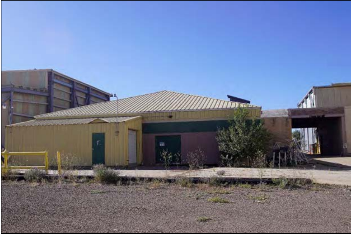
Figure 74. Photo of Building 5, facing south-southwest.
