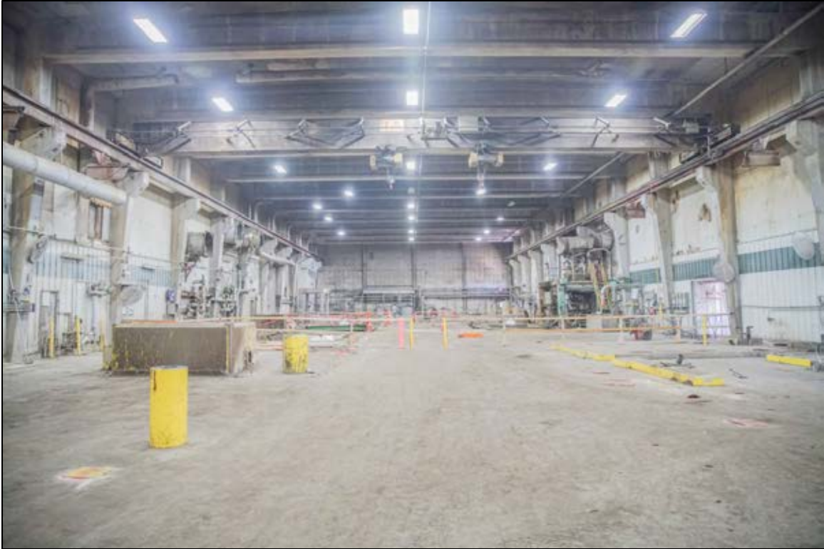
Figure 110. Building 3, north paper production room interior, facing north-northwest.
