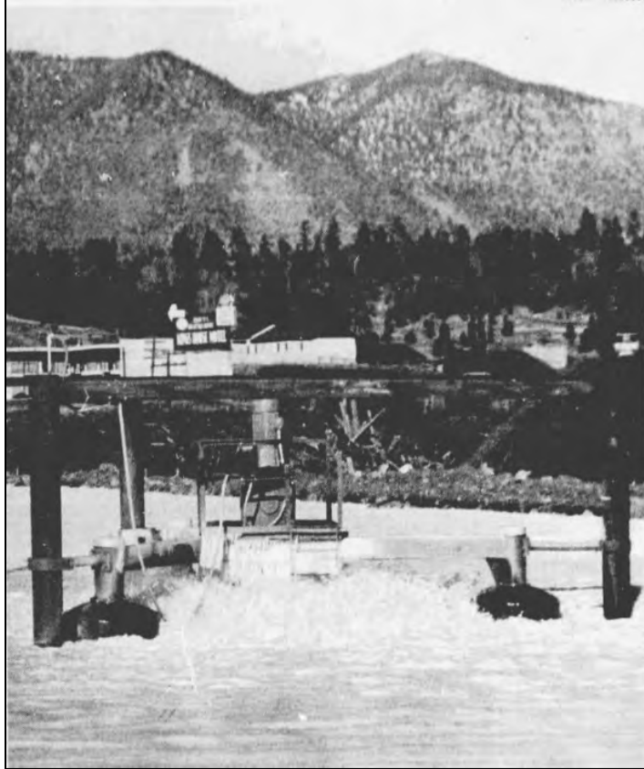
Figure 39. An aerator in the City's new water recycling lagoon (ADS January 5, 1972).
