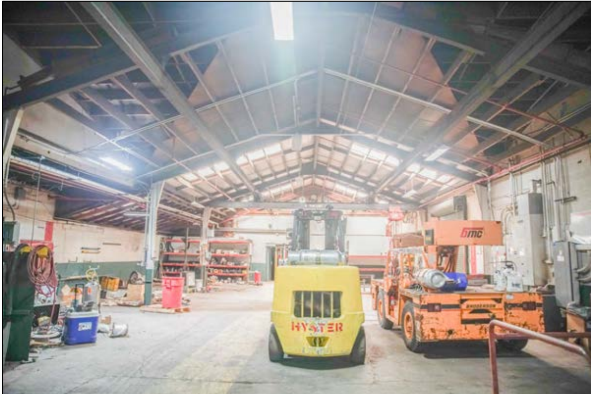
Figure 129. Building 7 interior, facing north toward Building 5.
