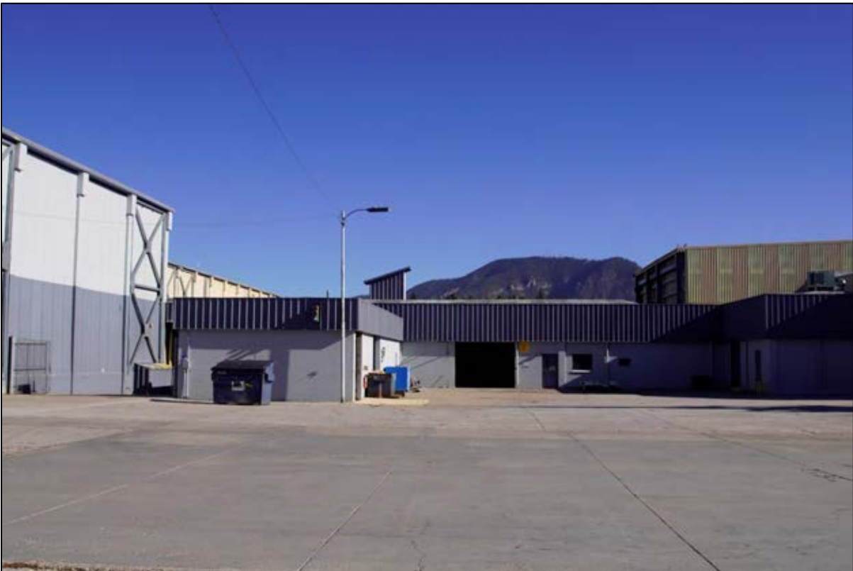
Figure 75. Photo of Buildings 7 and 8, facing north-northeast.
