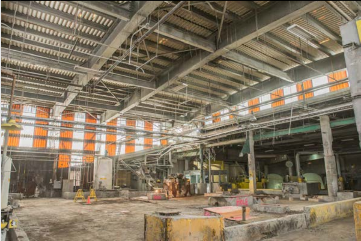
Figure 123. Building 6 interior, facing southeast.
