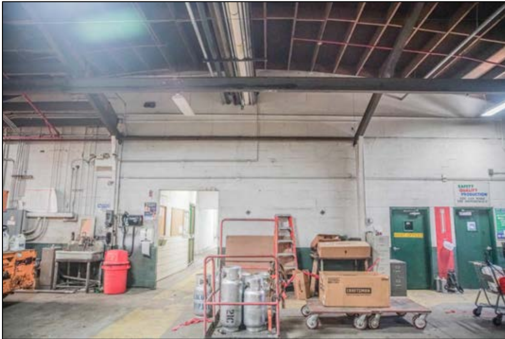
Figure 127. Building 7 interior, facing east.
