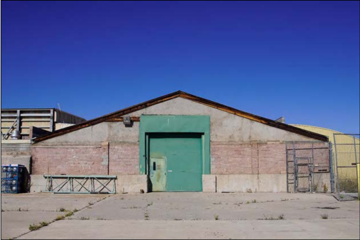
Figure 65. Photo of Building 2, facing west-northwest.
