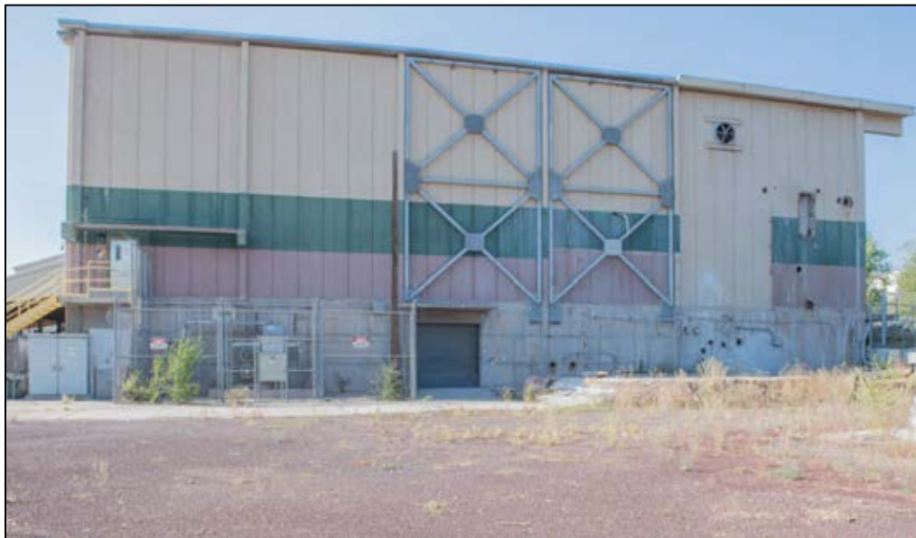
Figure 118. Building 3, north end door to basement.
