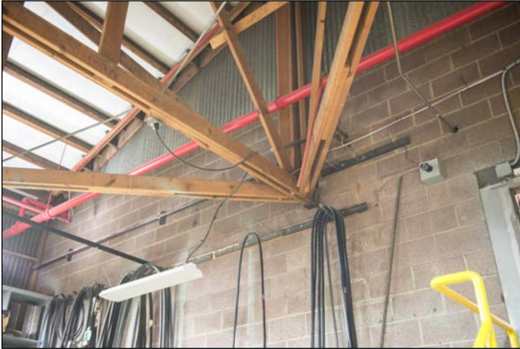
Figure 121. Building 5, interior trusses.
