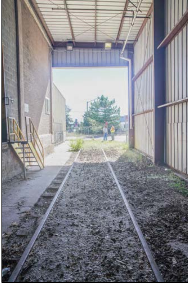
Figure 100. Building 1, southside rail spur and shed, facing east-northeast.
