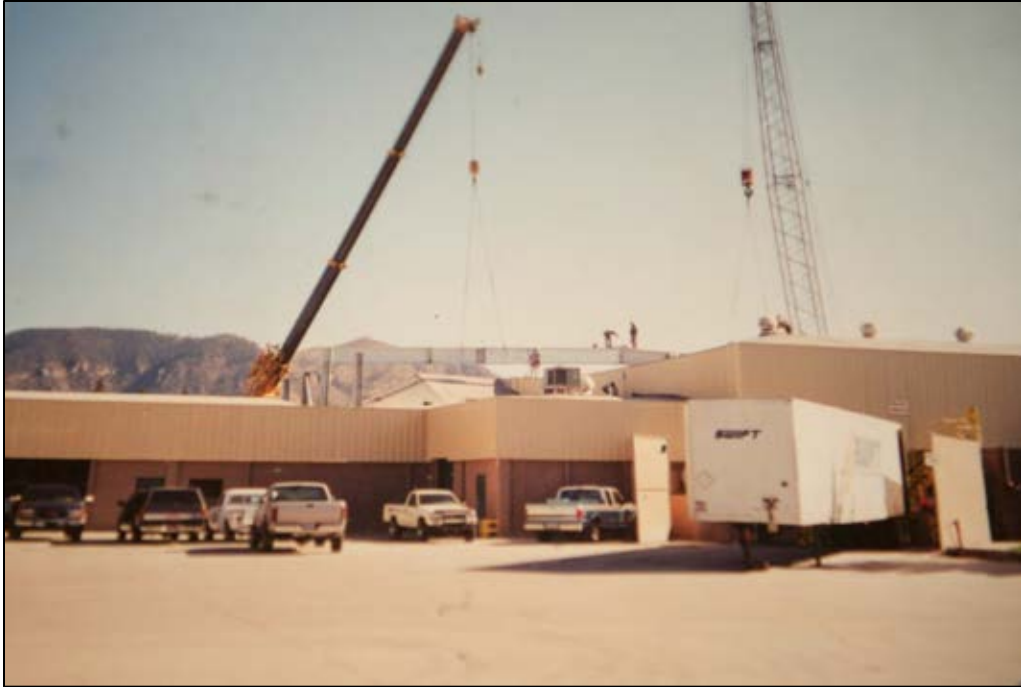
Figure 122. Building 6, roof repair.
