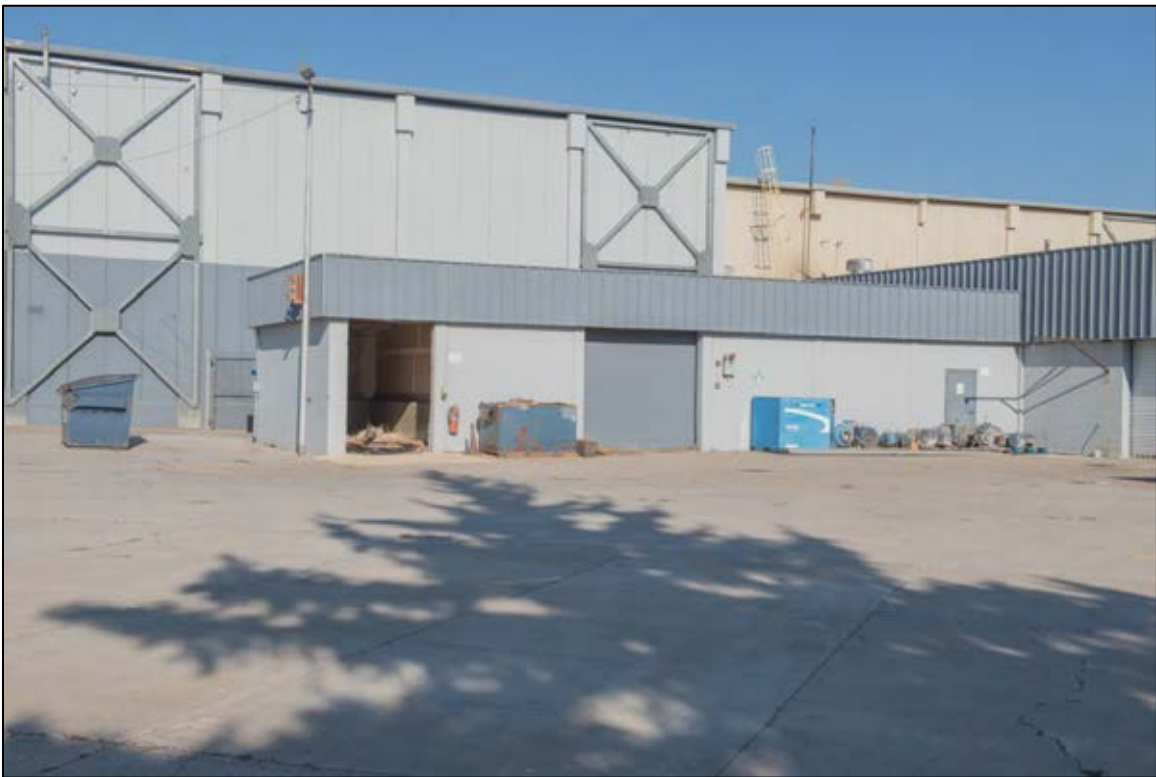
Figure 131. Building 8, facing west.
