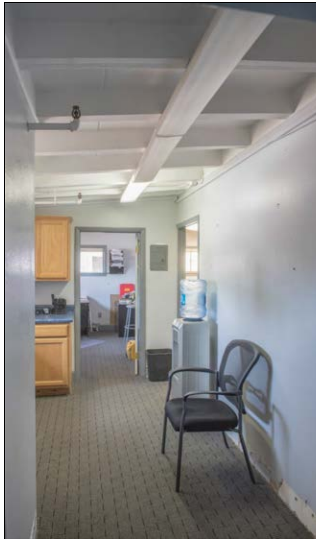
Figure 119. Building 4 interior showing open beam ceiling.
