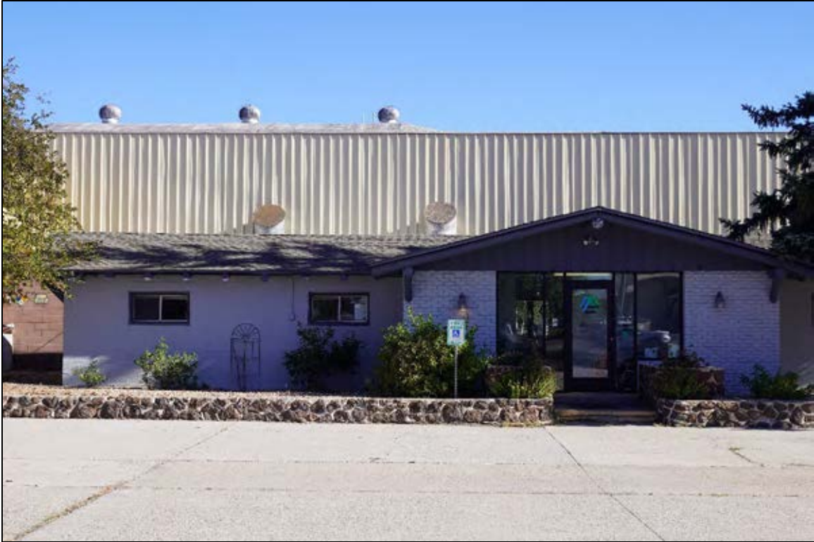
Figure 73. Photo of Building 4, facing north-northeast.
