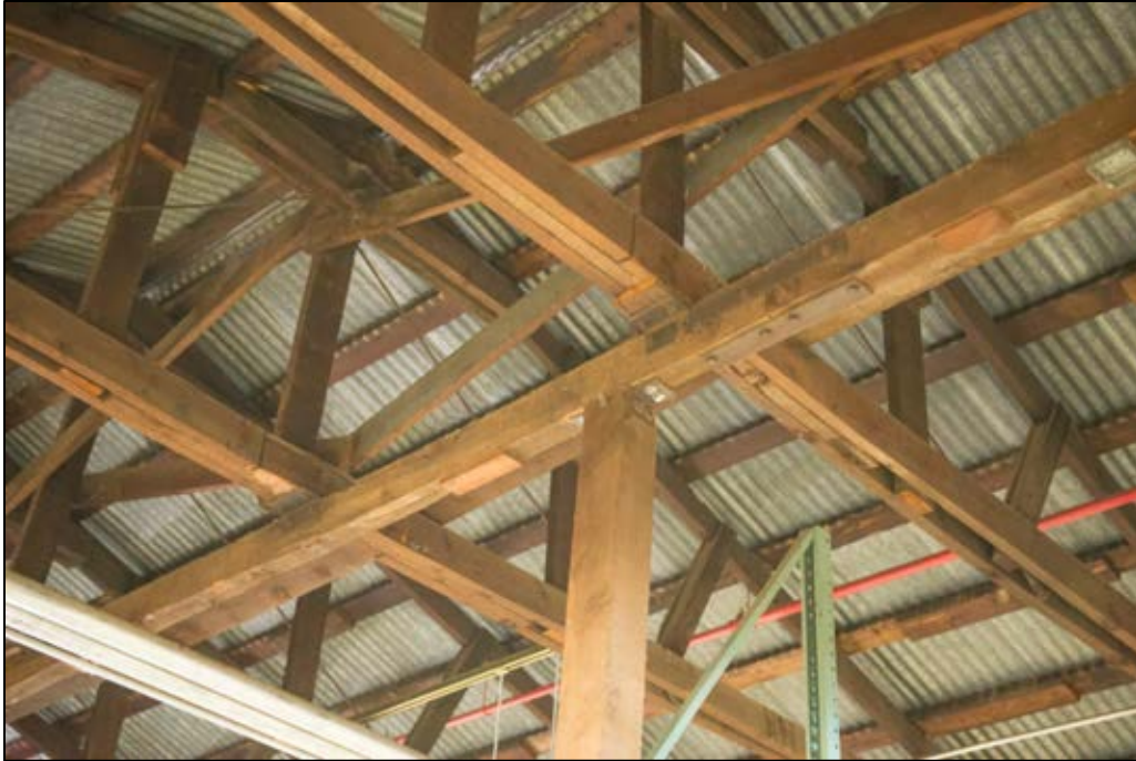
Figure 102. Building 2 roof trusses above post and beam construction.
