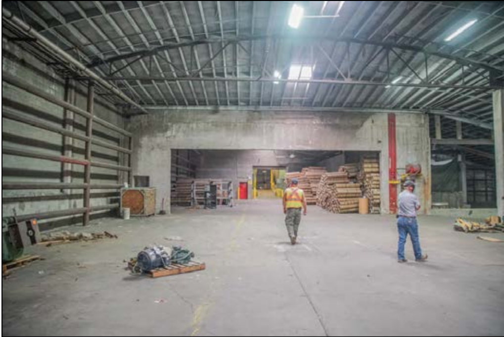
Figure 92. Photo of Building 1, eastern warehouse shear wall, facing west-northwest.
