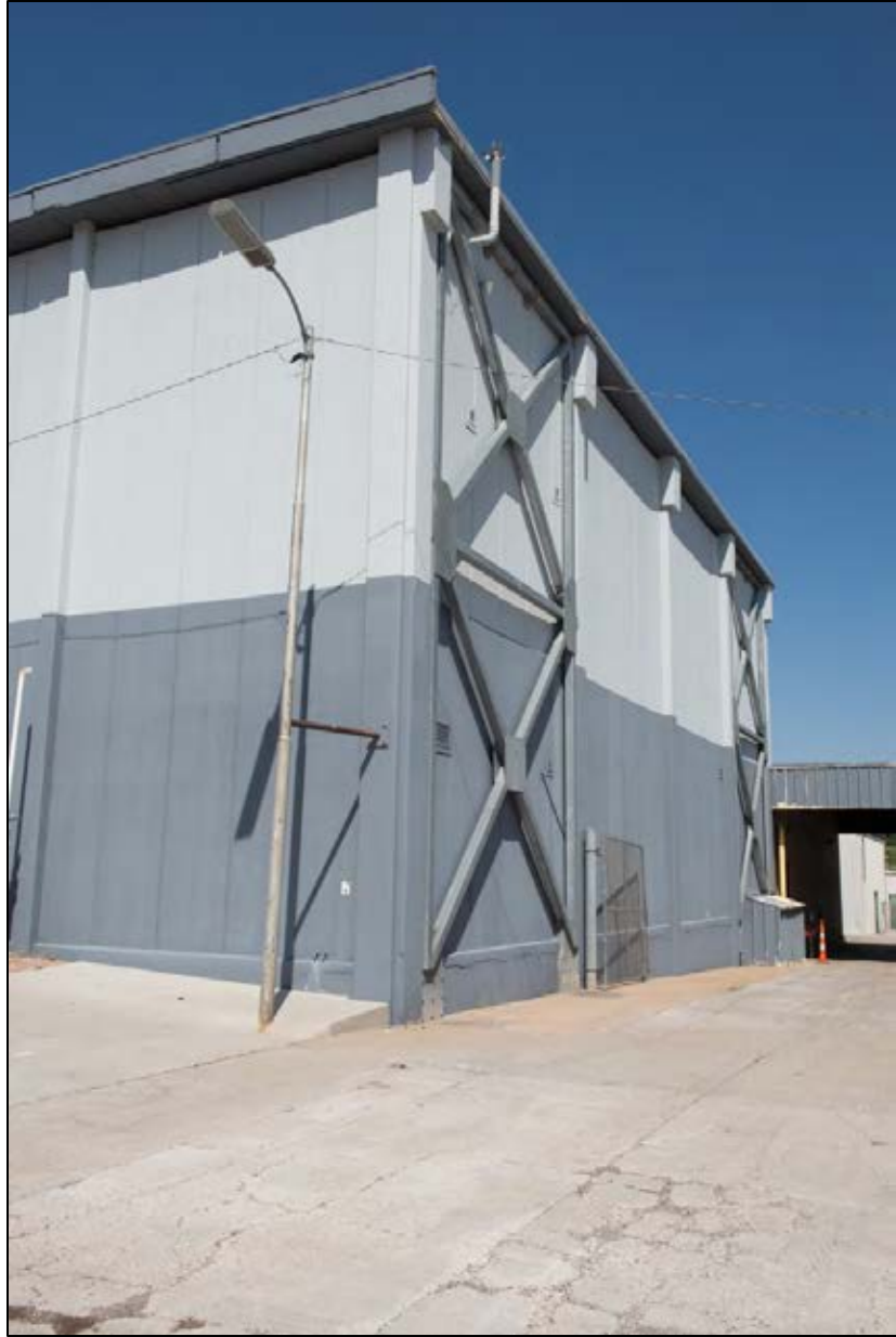
Figure 114. Building 3, braced frames, facing north-northwest.
