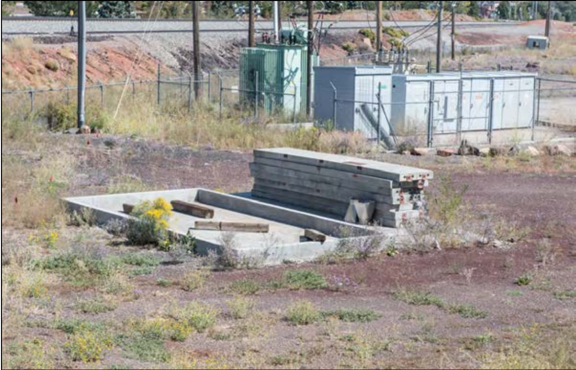
Figure 105. Building 3 pre-stressed roof replacement panels.
