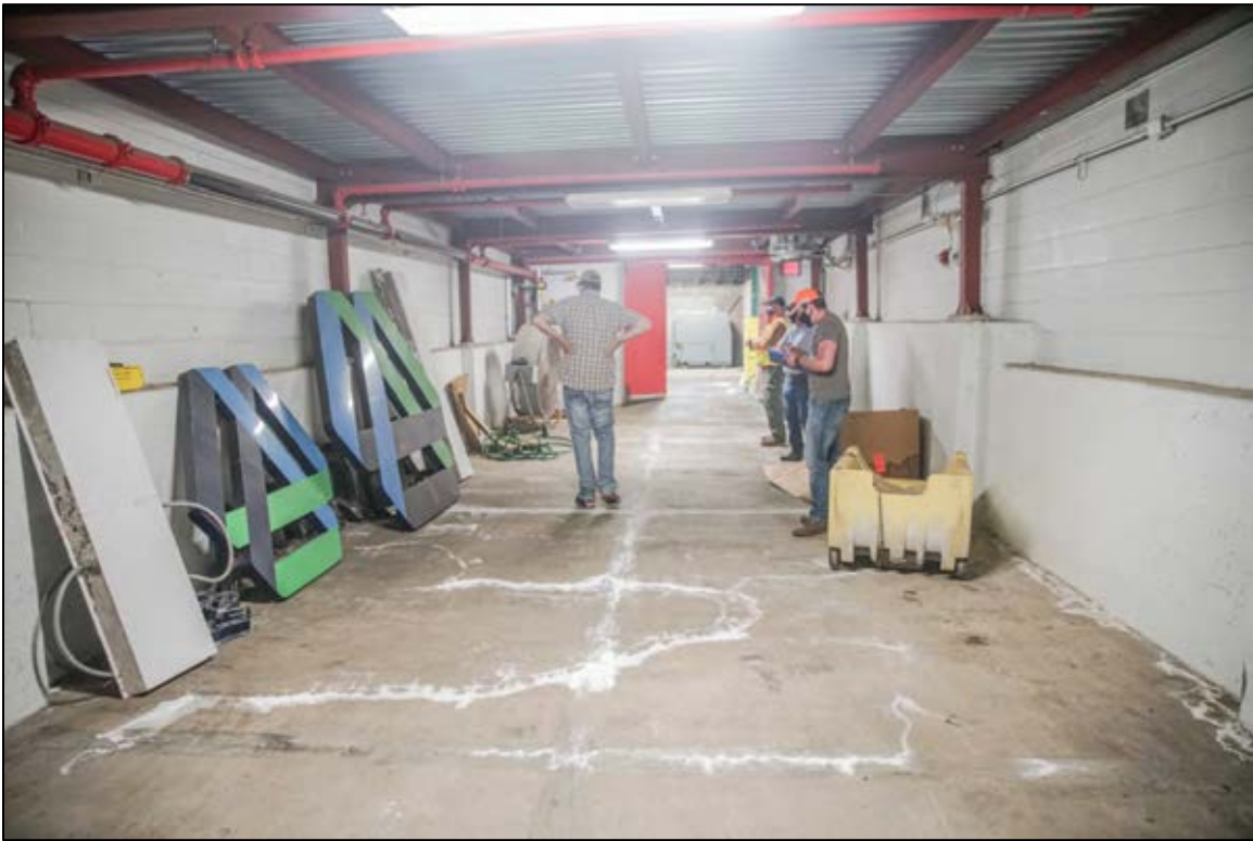
Figure 104. Building 2 connector, facing south-southwest.
