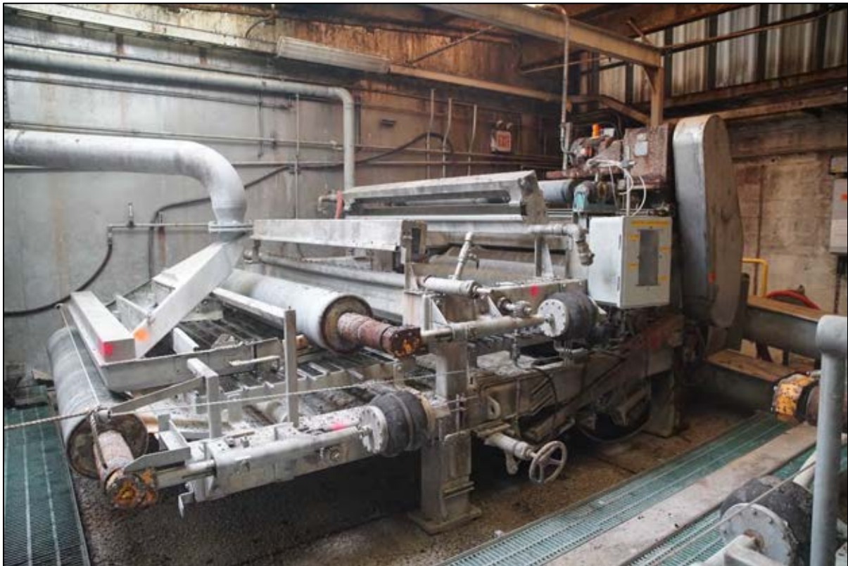
Figure 78. Photo of Building 6 interior showing fiber preparation equipment, facing southeast.
