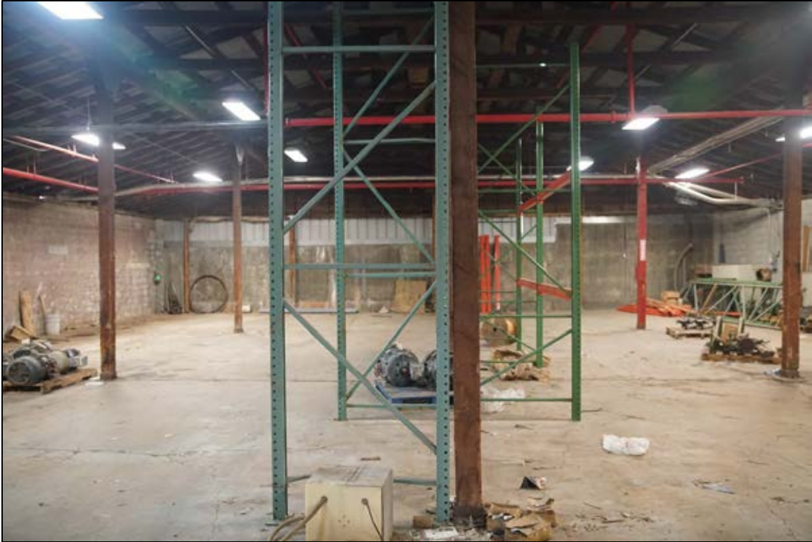
Figure 67. Building 2 interior, facing west-northwest.
