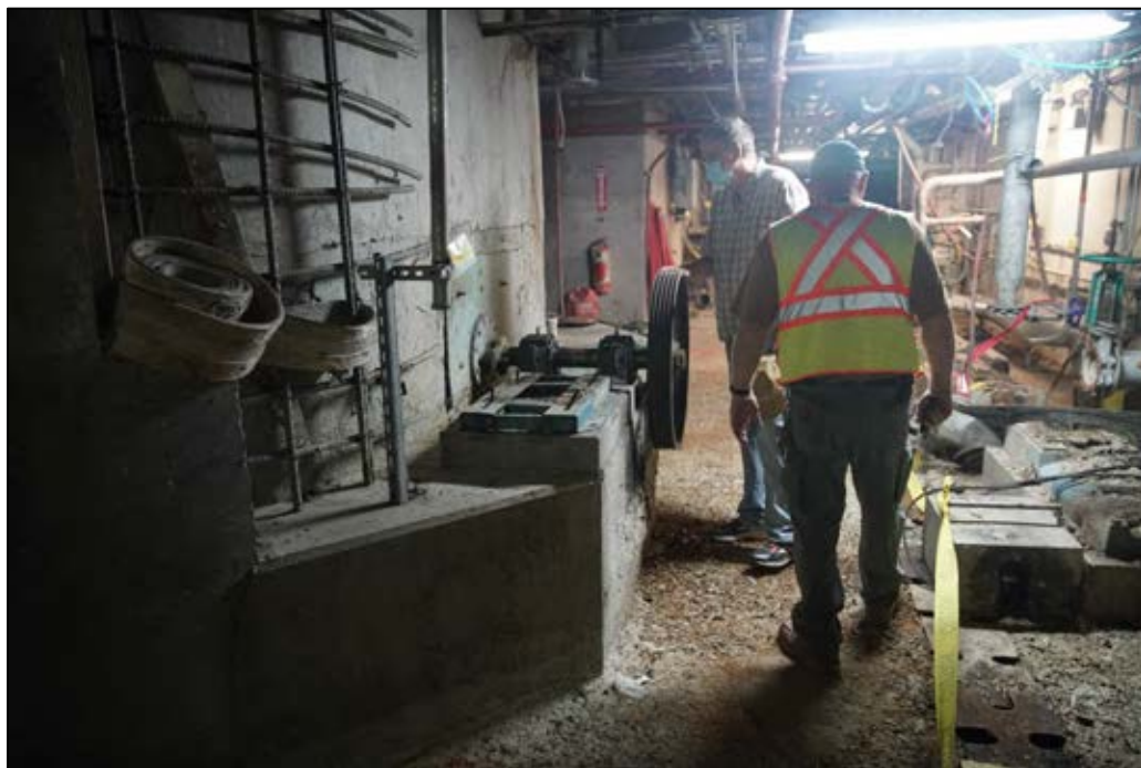
Figure 126. Building 6, basement, facing west.
