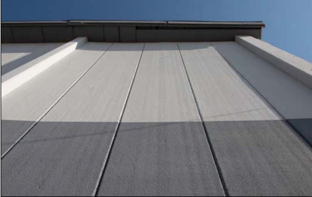
Figure 115. Building 3, exterior wall panels.
