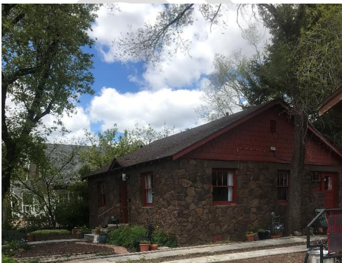
Figure 9: Vernacular malpais house on Cottage Avenue
