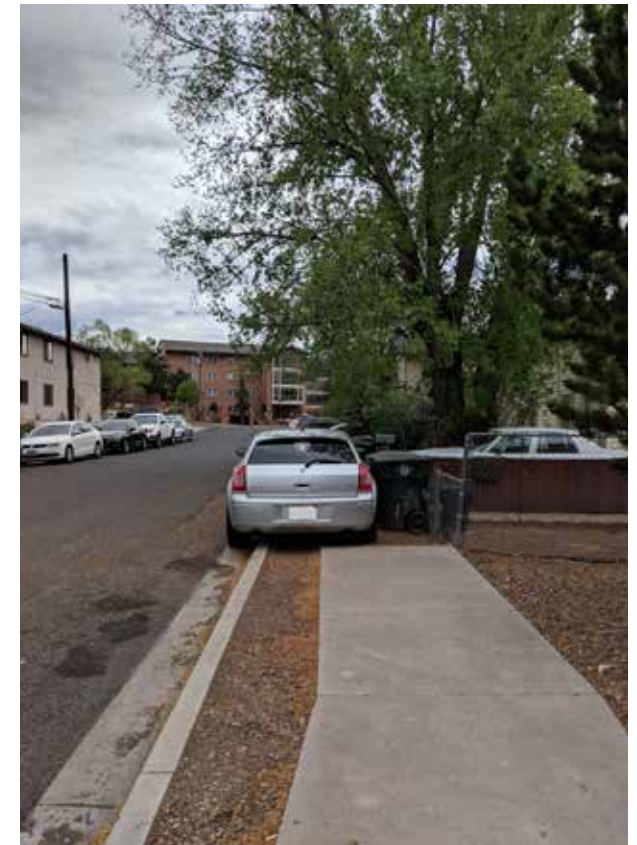
Incomplete street infrastructure in the Southside contributes to parking issues
