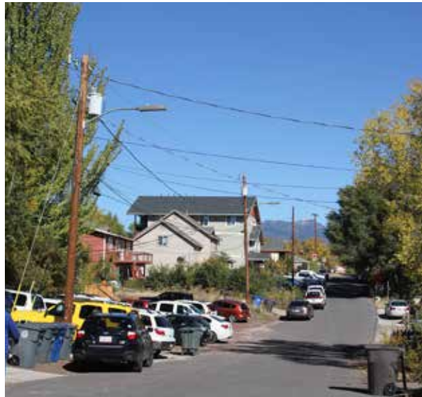
South Fontaine Avenue south of Franklin Avenue demonstrating irregular parking due to lack of curb, gutter and sidewalk
