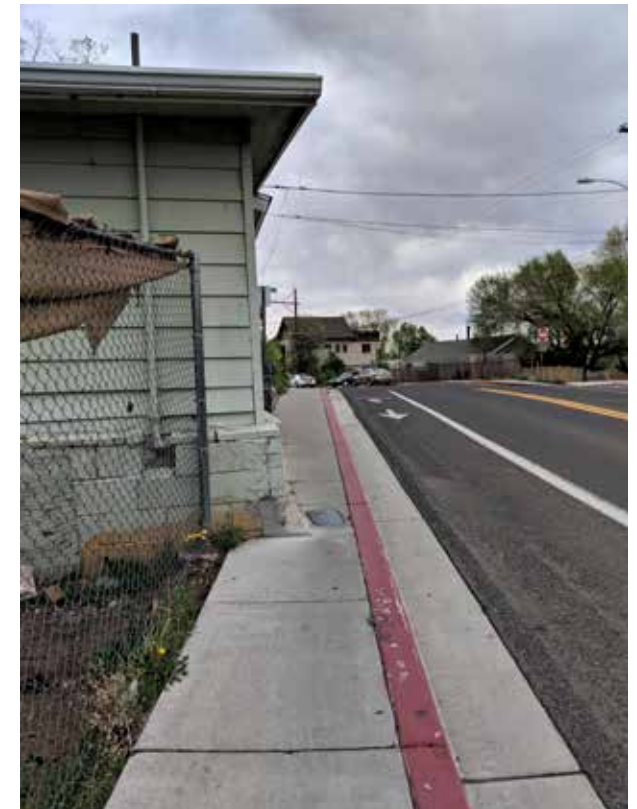
Encroachment into the City right-of-way on Franklin Avenue
