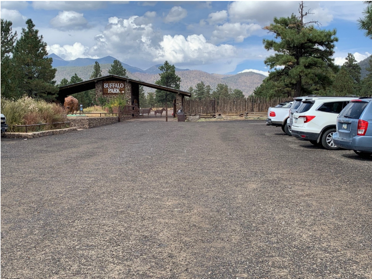
Parking lot and entryway. Accessible parking will be installed along the right side where vehicles are parked
