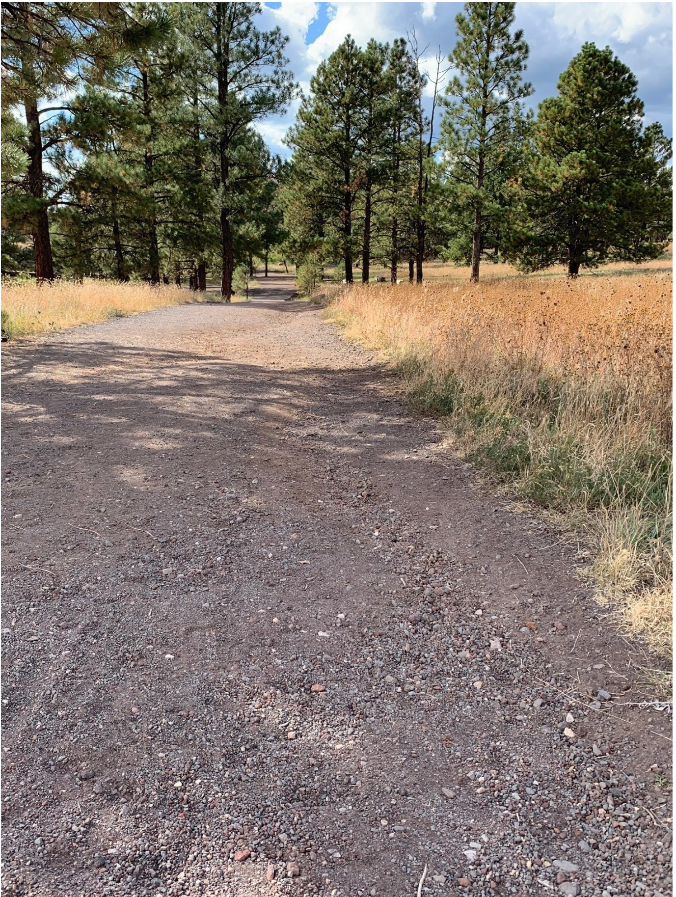
The aggregate trail surface of the Nate Avery Trail is often loose and not suitable for wheelchairs
