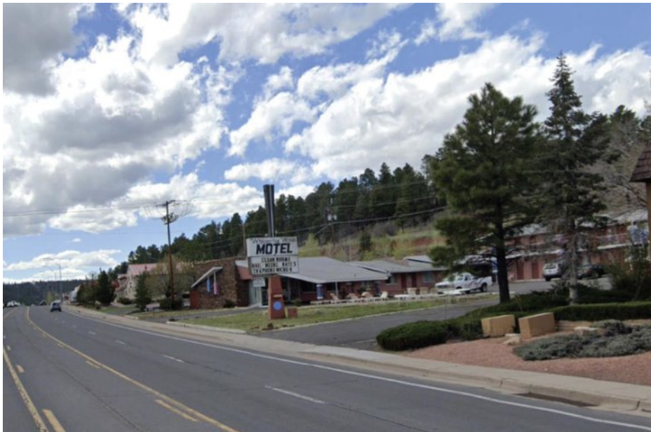
Existing Sign Condition
