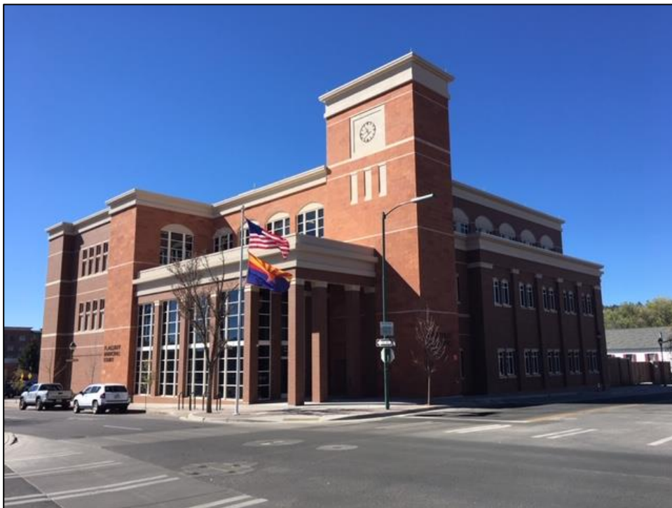
Flagstaff Municipal Court Facility, looking at the main entrance – northeast corner
