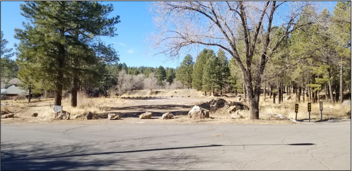
Dale Ave. / Mogollon St. intersection looking west Removed fencing and installed boulders around the southwest portion of the Thorpe Park Annex
