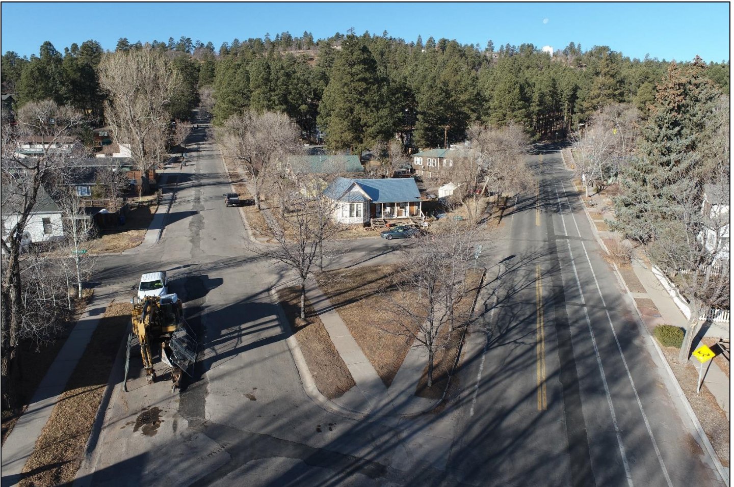
Summit Water Project-Trenches patched for winter
