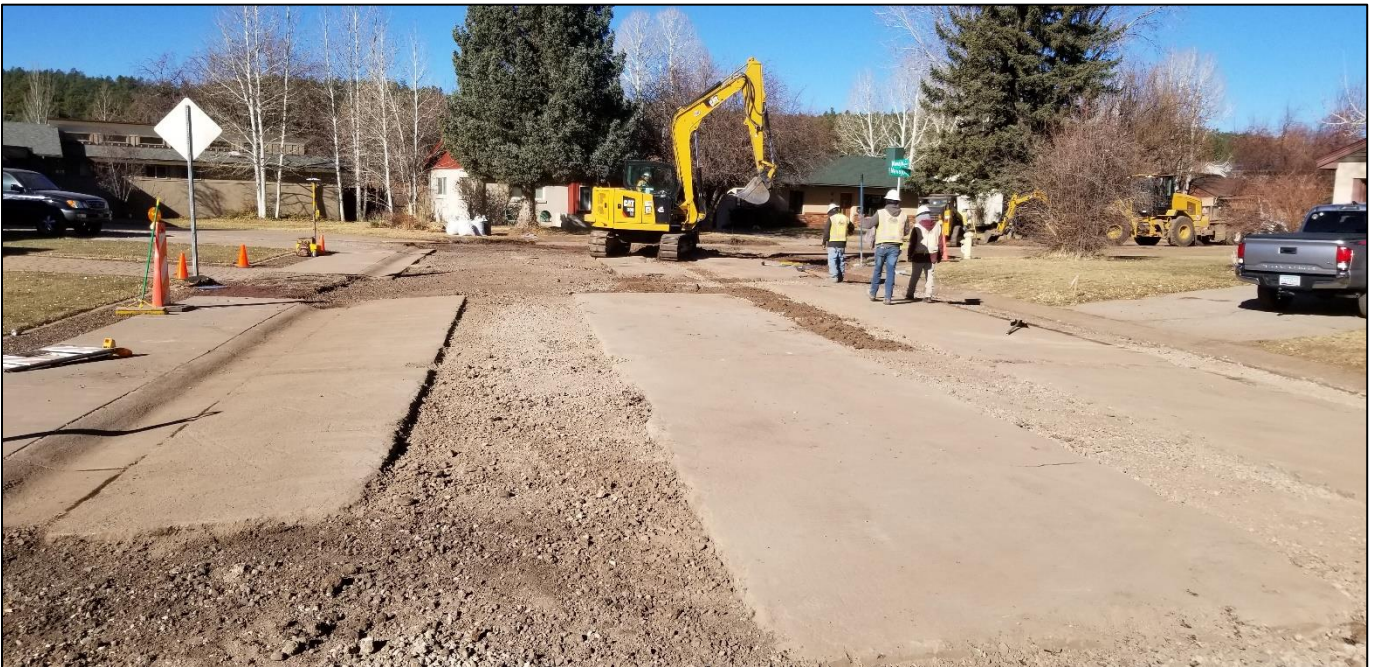
Navajo Rd. / Navajo Dr. intersection looking west Preparing the roadway for asphalt patching over trenches for a clean site prior to the Neighborhood Luminarias Event
