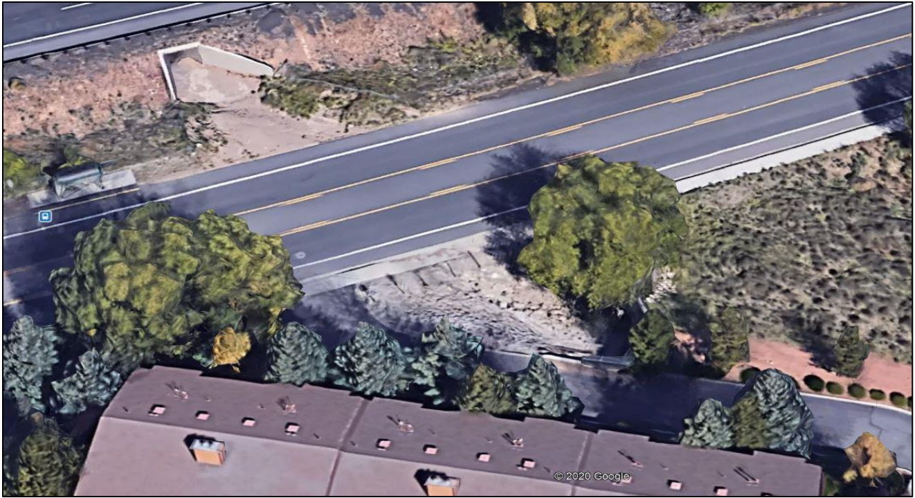
Google Earth image of existing low water crossing across Soliere Ave. Current condition allows stormwater to discharge from the box culvert and across Soliere Ave. Planned improvements will convey stormwater underneath Soliere Ave.
