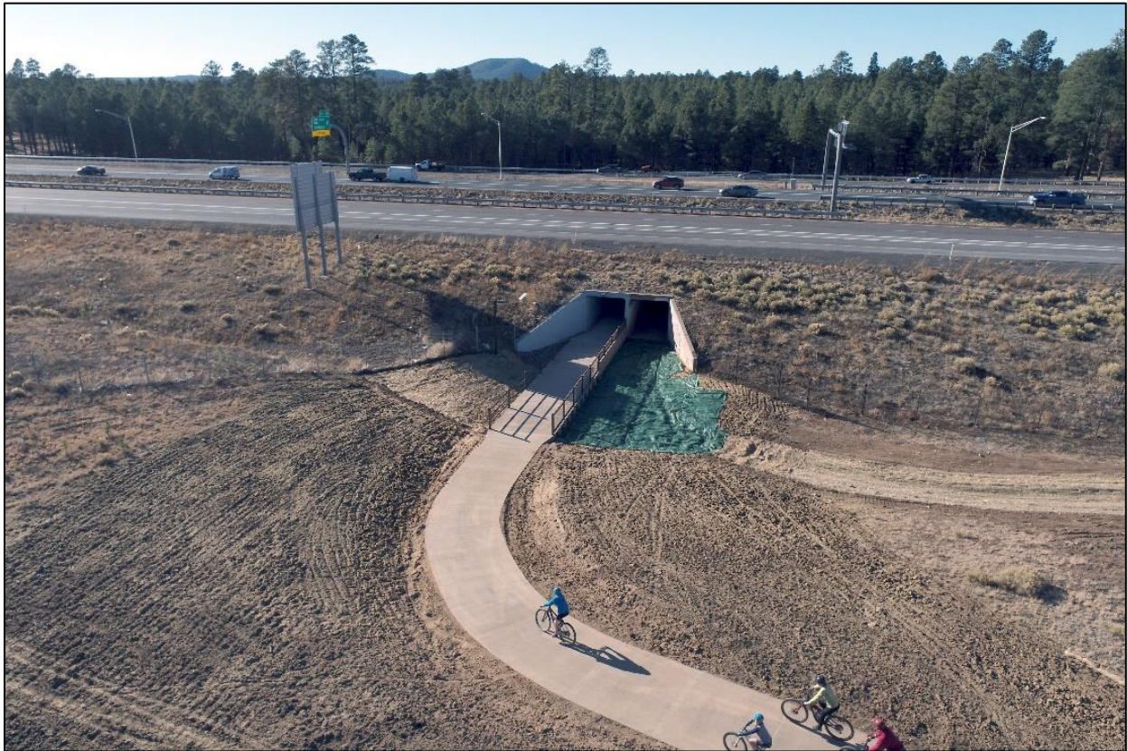
Looking west at the eastern portal. Note Interstate 17 above the tunnel and the drainage tunnel to the right of the FUTS tunnel.
