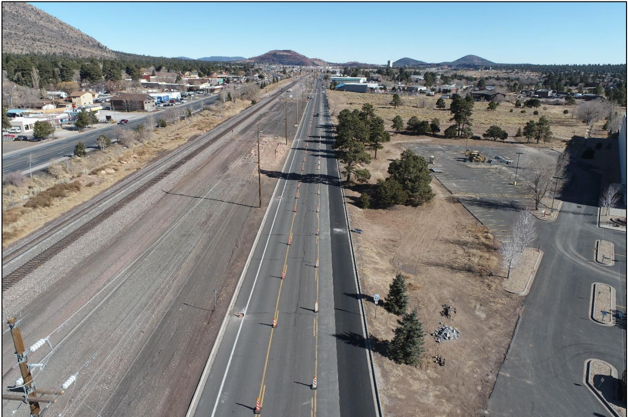
Industrial Drive ready for striping and valve adjustments, Industrial Dr. looking east
