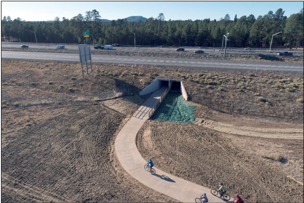
Looking west at the eastern portal. Note Interstate 17 above the tunnel and the drainage tunnel to the right of the FUTS tunnel.
