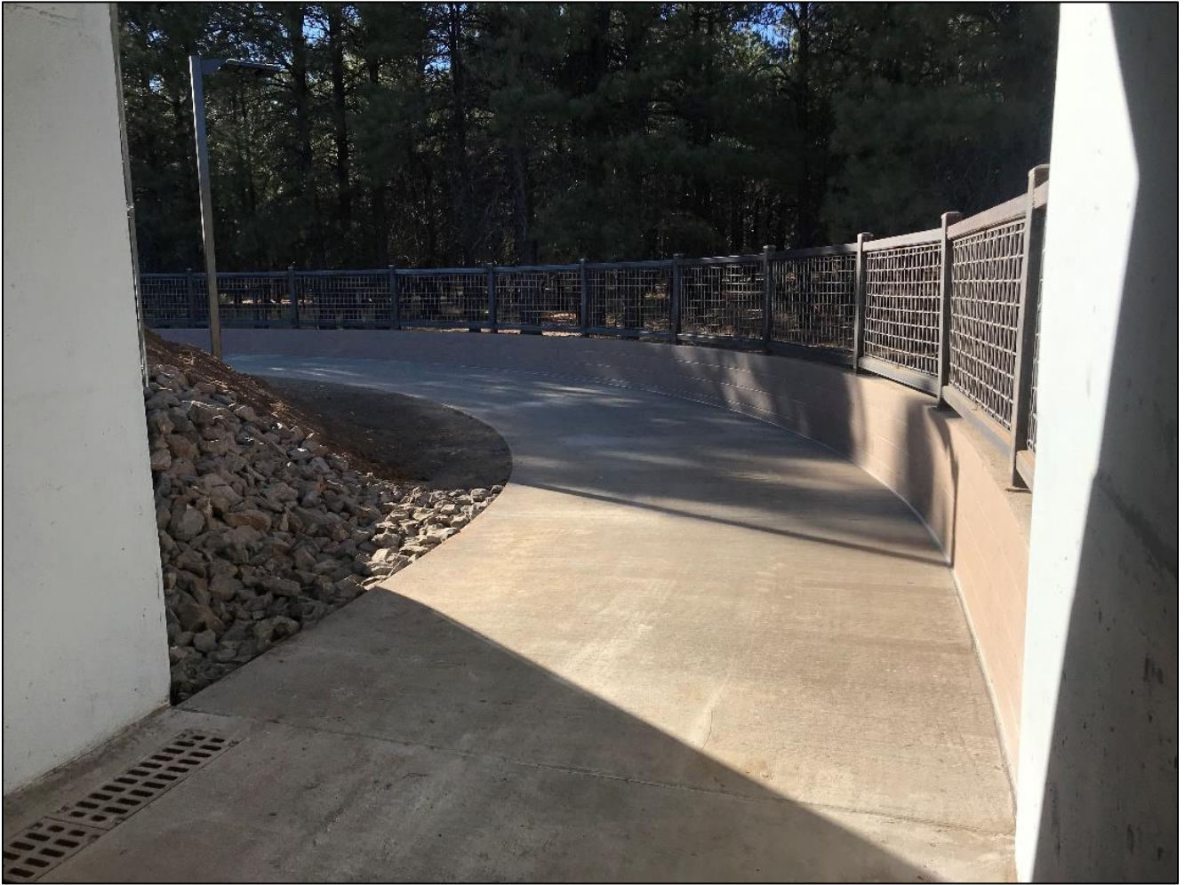
Looking west out the western portal. Note the FUTS safety fence at right and trench drain at left.
