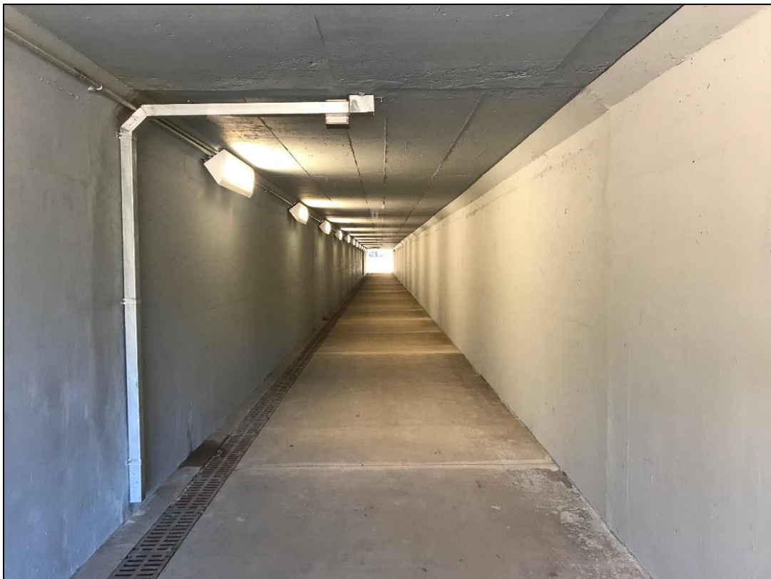
Looking west through the tunnel. Note the interior lighting and heated weep drain frost protection conduit.
