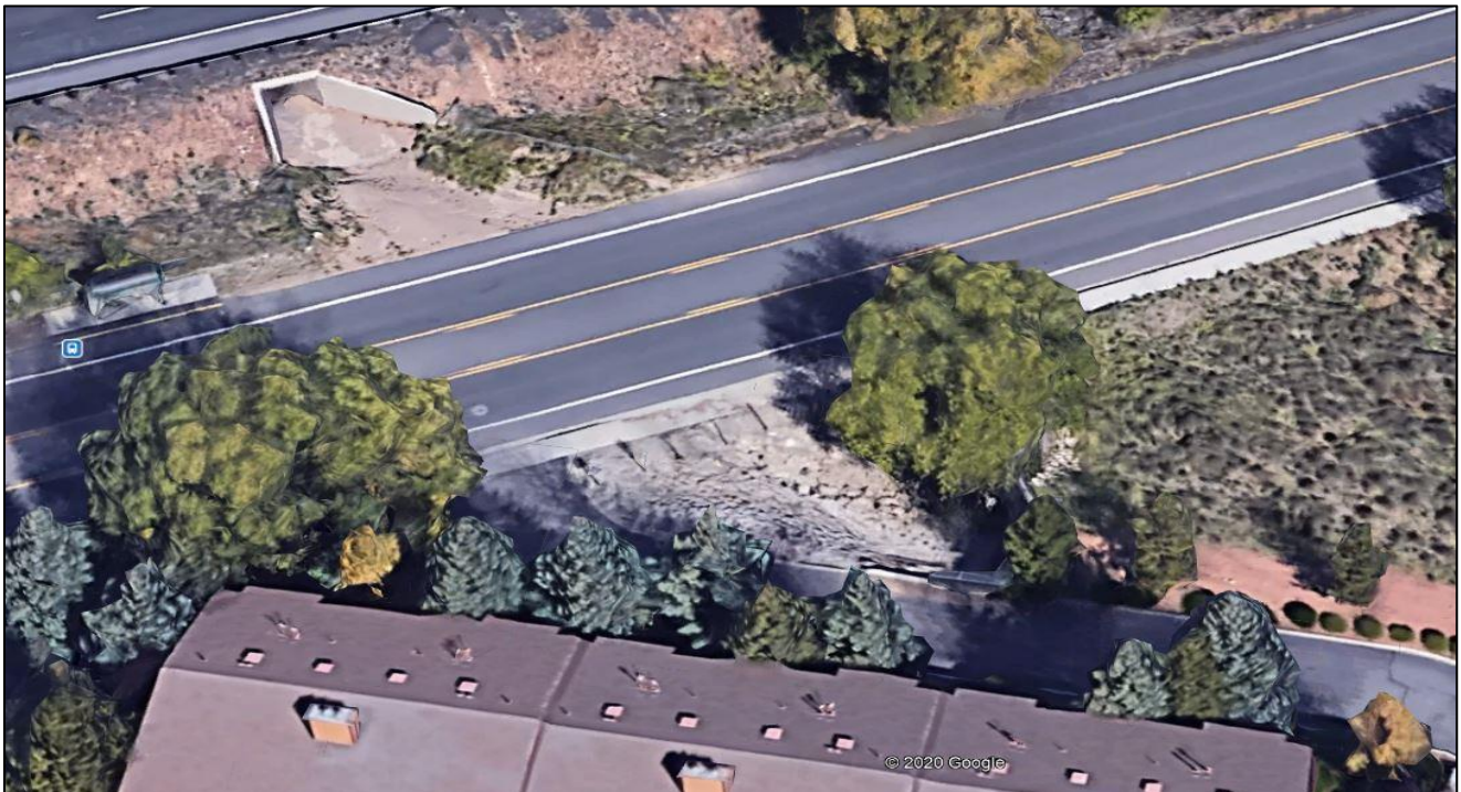
Google Earth image of existing low water crossing across Soliere Ave. Current condition allows stormwater to discharge from the box culvert and across Soliere Ave. Planned improvements will convey stormwater underneath Soliere Ave.
