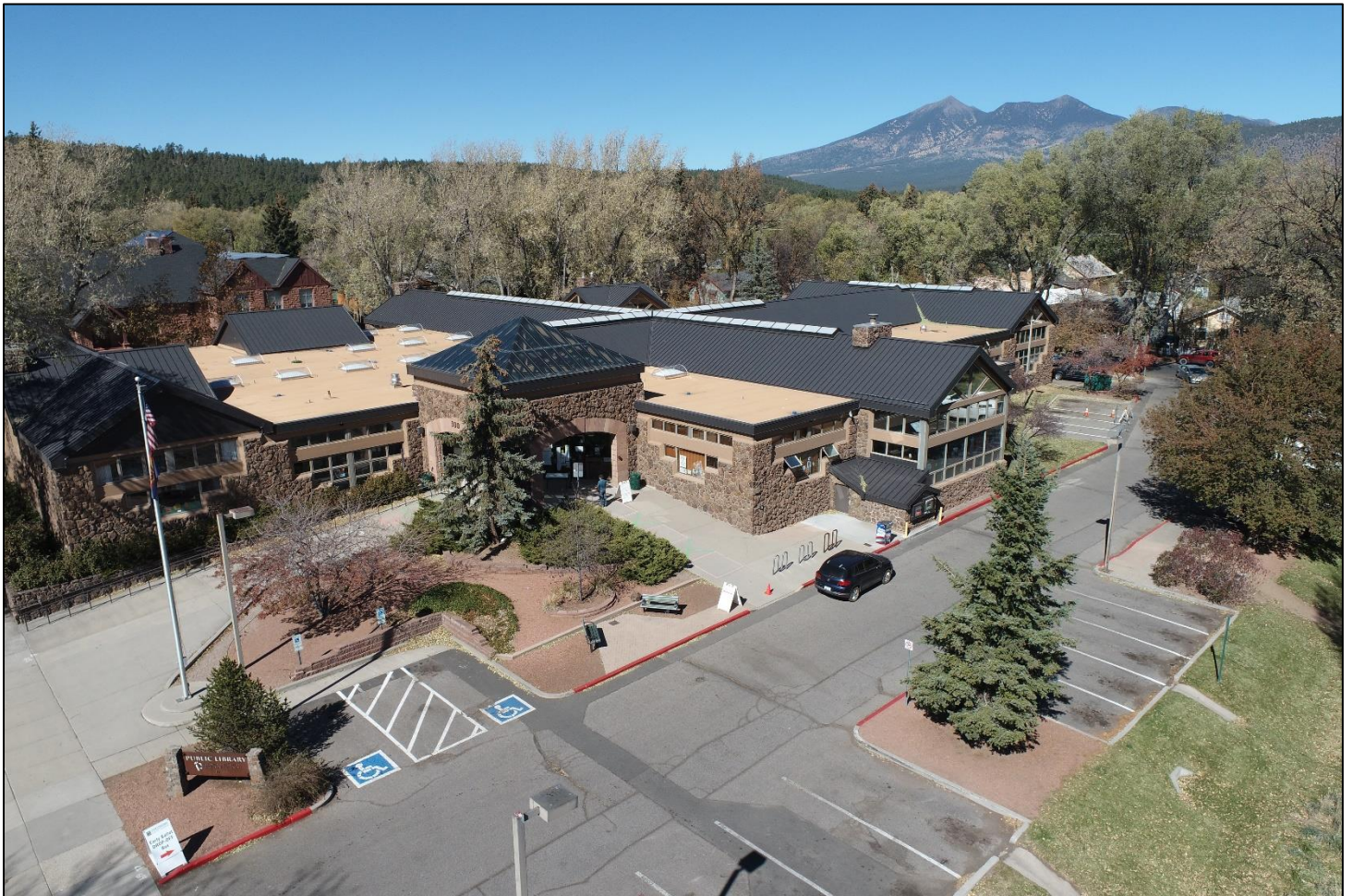
Library Entrance Project-Existing Conditions
