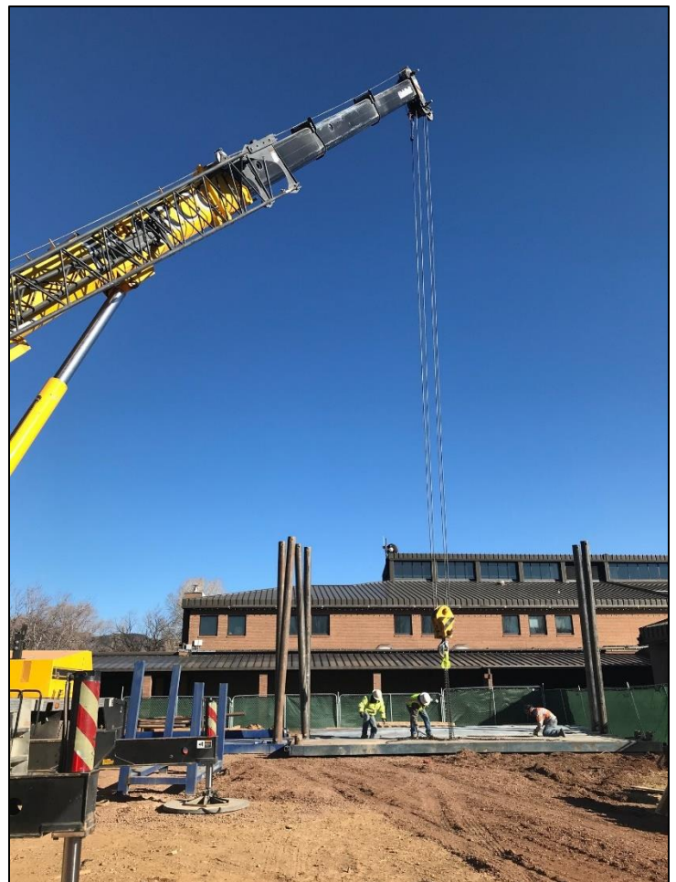
Trench shoring box preparation using a 90 ton crane
