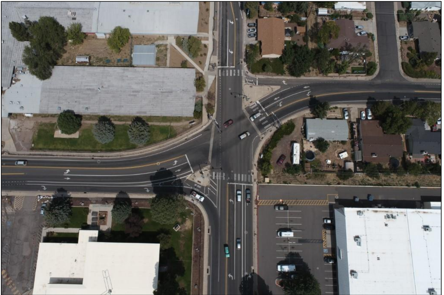
Existing Lockett-Cedar-Fourth Intersection
