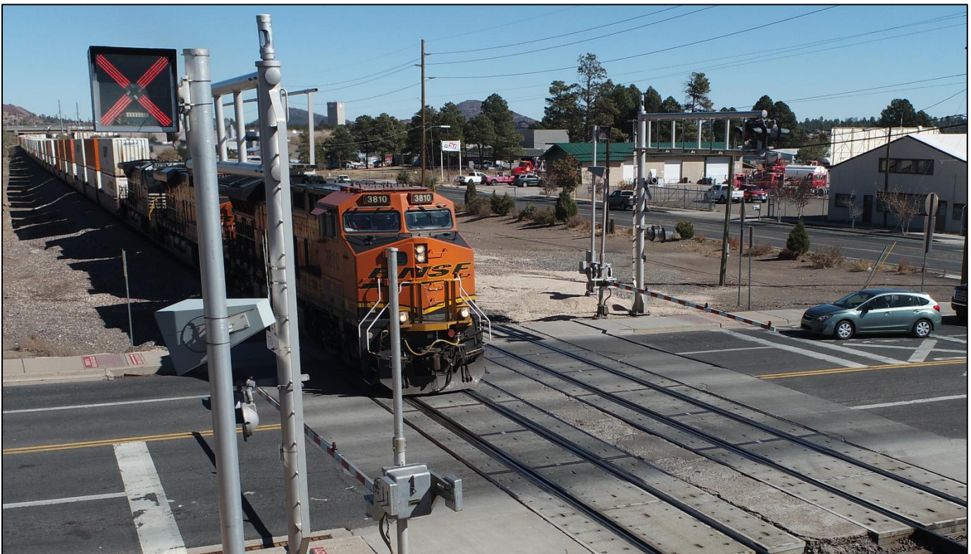
Fanning Railroad Crossing
