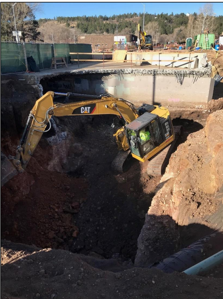
Wingwall excavation at the northeast side of the new bridge
