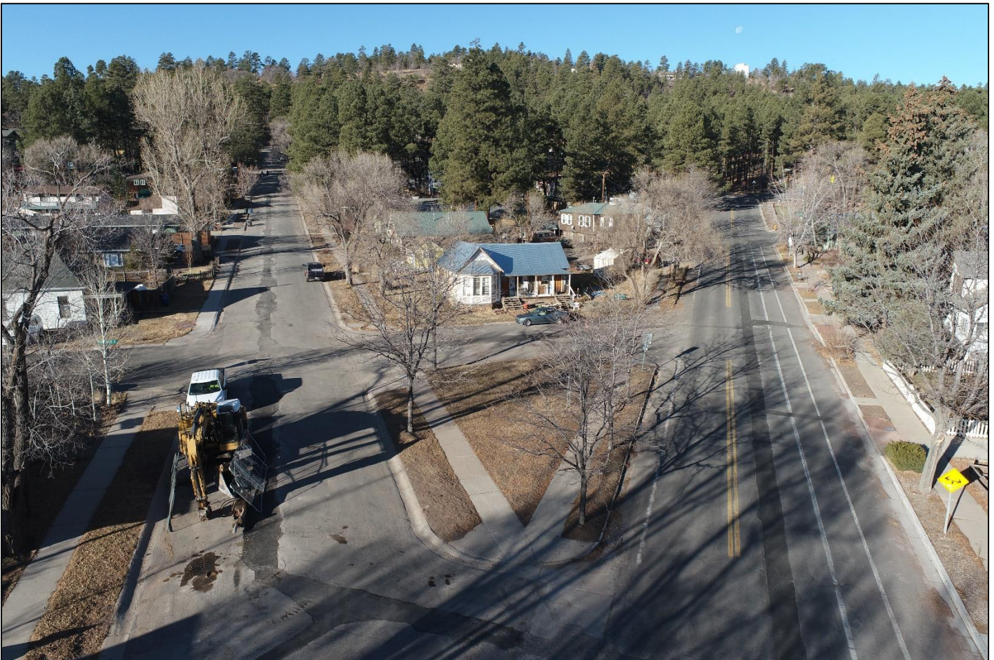
Summit Water Project-Trenches patched for winter
