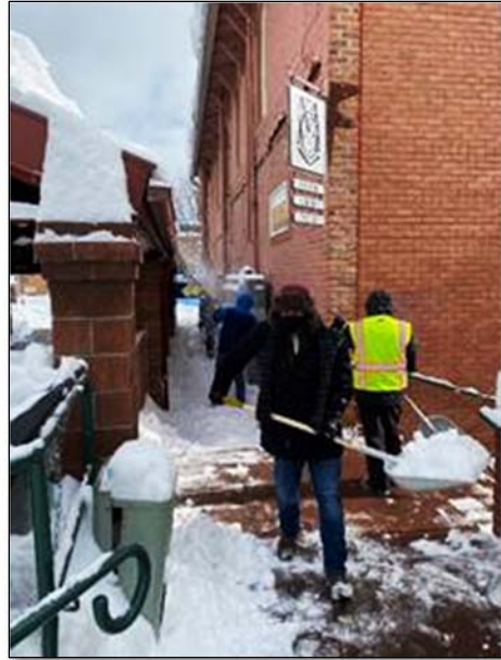
Clearing snow - parking garage canopy
