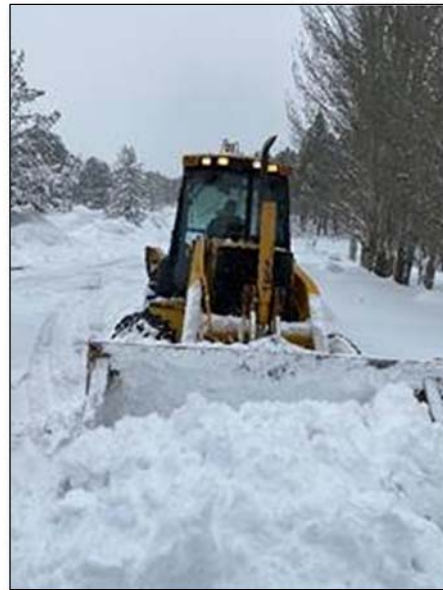
Parks Maintenance Worker Kevin Whealy along Butler
