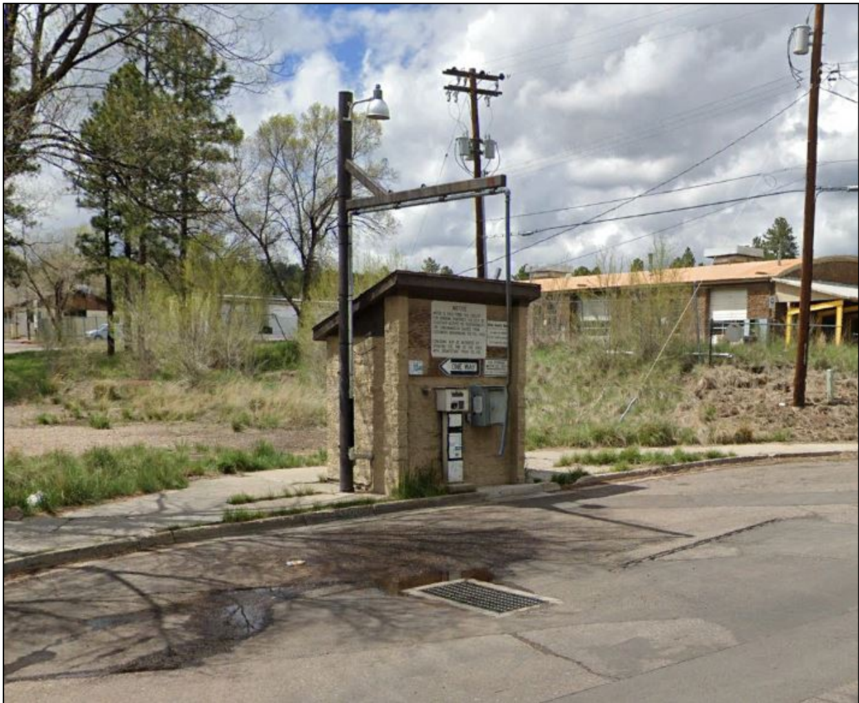
Existing potable water loadout station on Bonito Street
