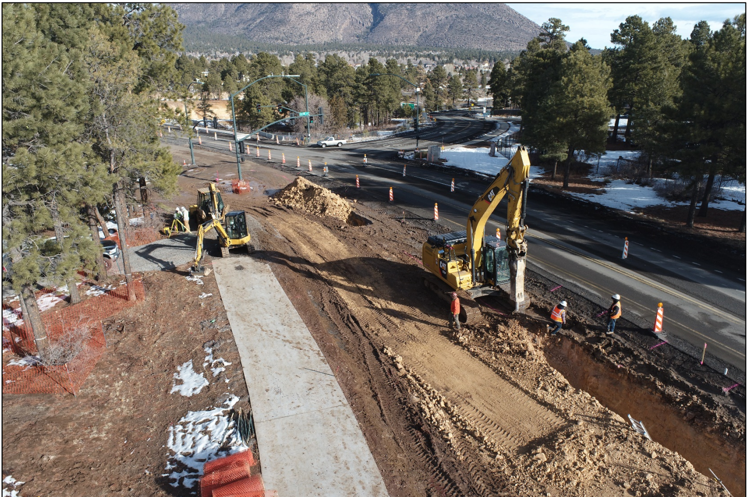
Fourth Street Reconstruction –Project underway
