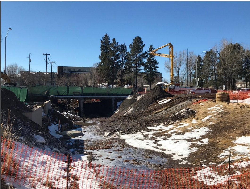
Backfill complete on the north side of the Rt. 66 and concrete placement of the southwest wingwall
