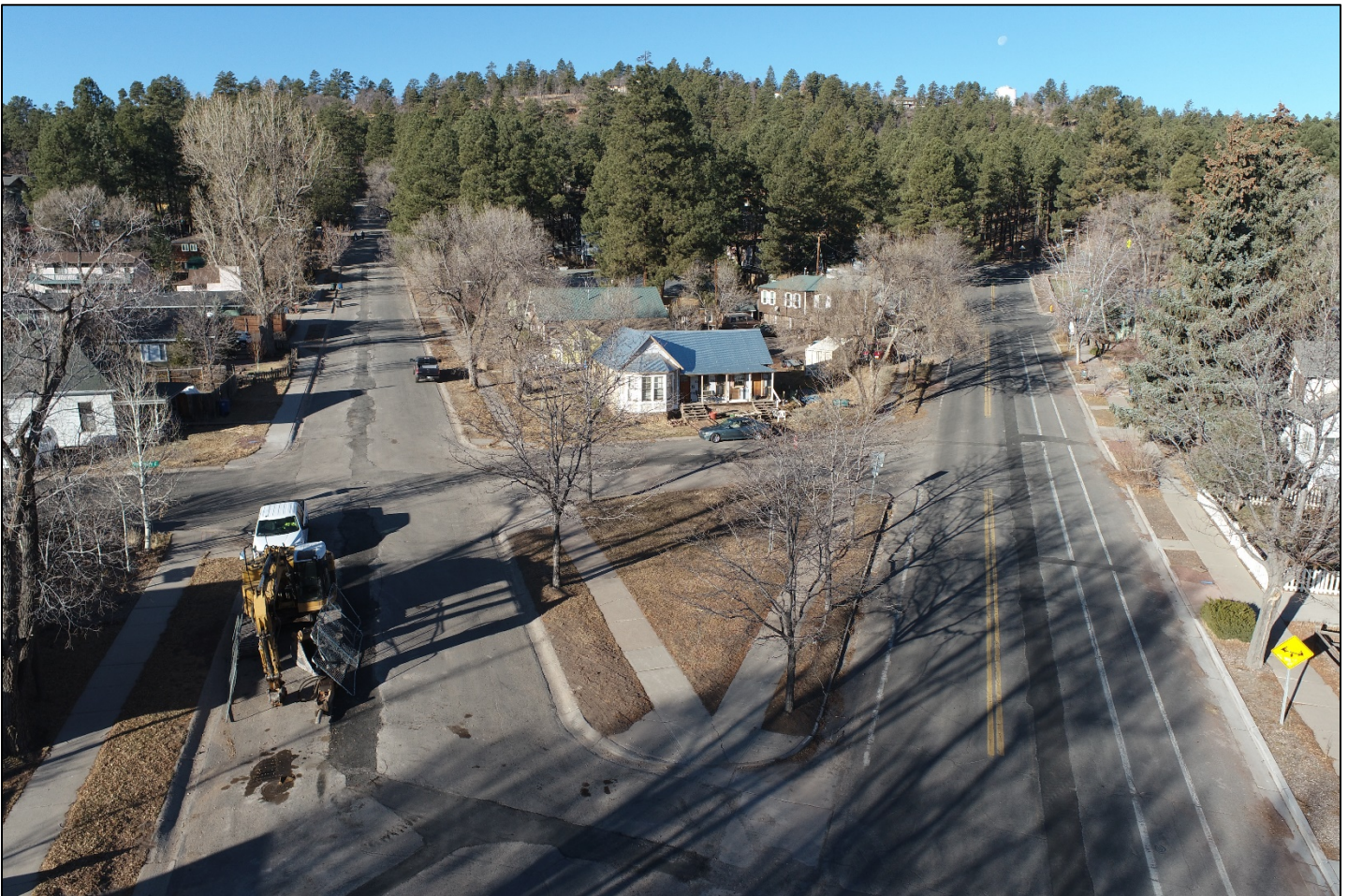
Summit Water Project-Trenches patched for winter
