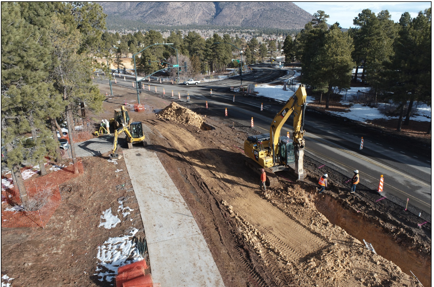
Fourth Street Reconstruction –Project underway
