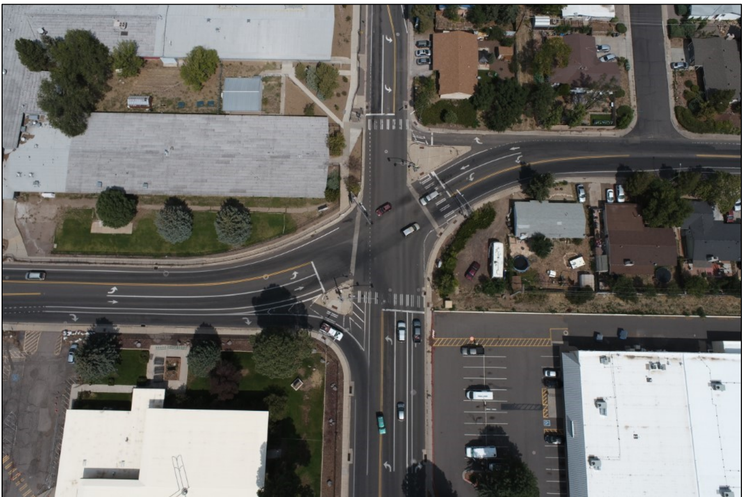
Existing Lockett-Cedar-Fourth Intersection
