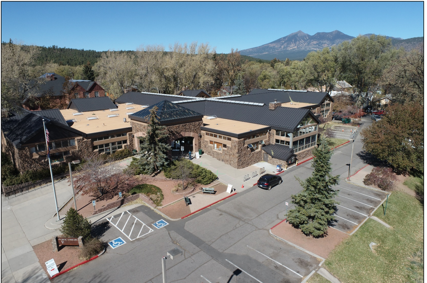
Library Entrance Project-Existing Conditions
