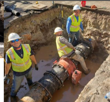
Clay Ave pipeline repairs
