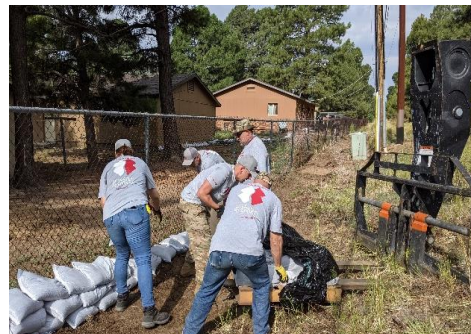
Team Rubicon placing sandbags
