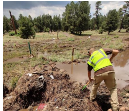
Clearing a pine needle dam
