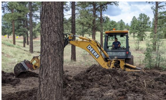
Distribution staff dredging a channel
