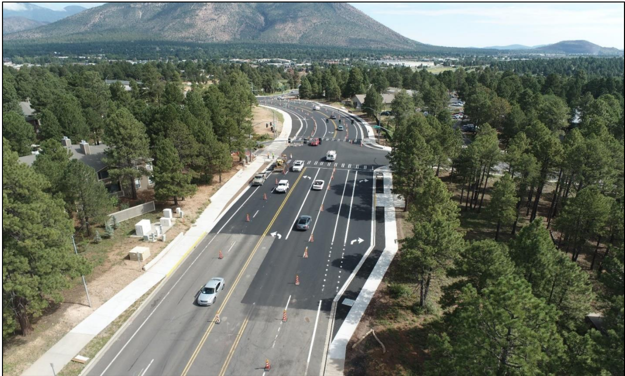
Fourth Street Reconstruction –Initial Striping installed
