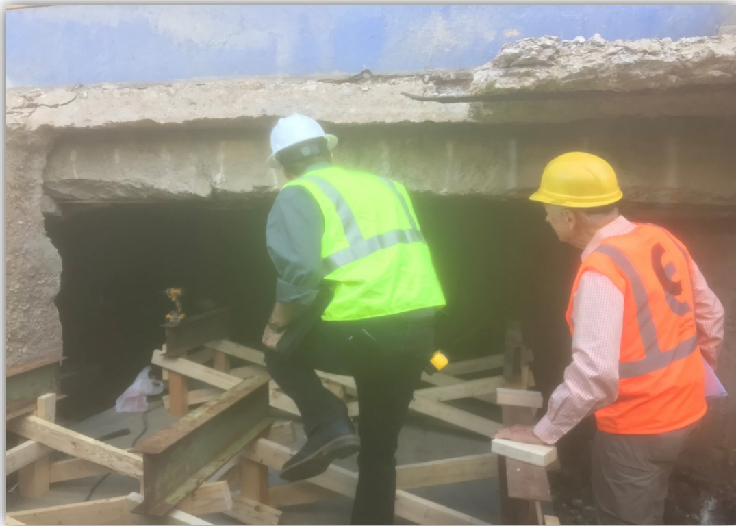
Inspection of temporary shoring for the Zani Beam
