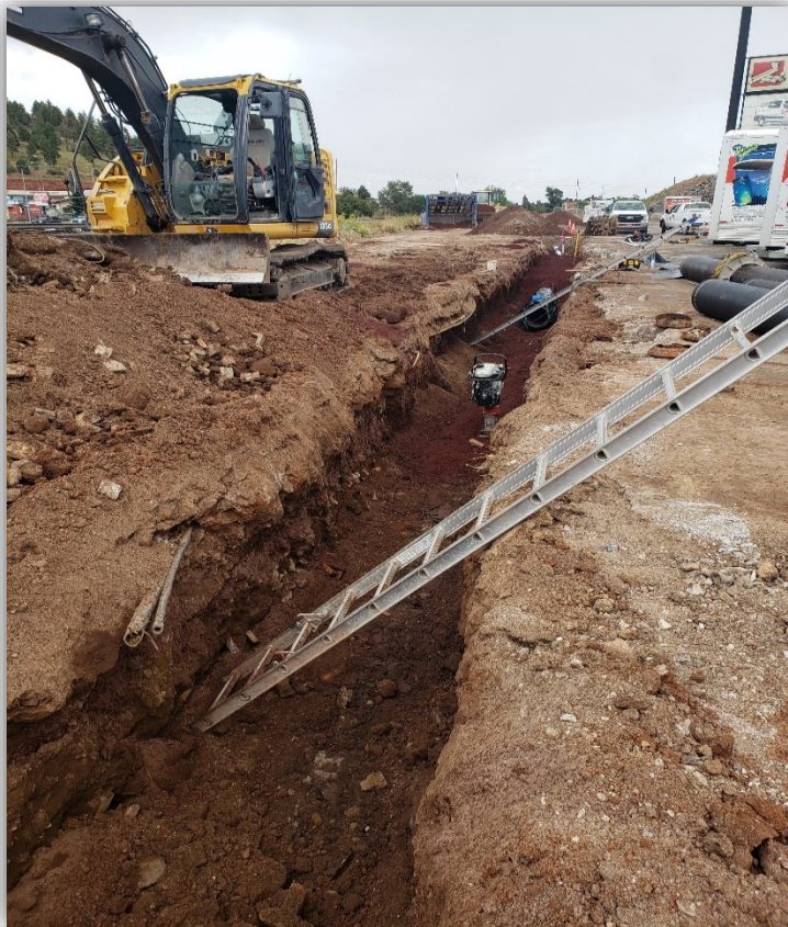
Installation of the 16" waterline
