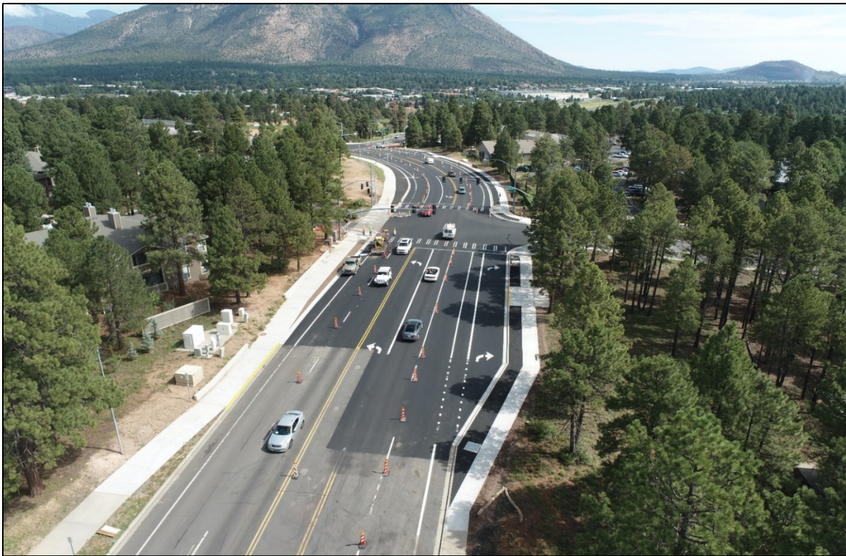
Fourth Street Reconstruction –Initial Striping installed
