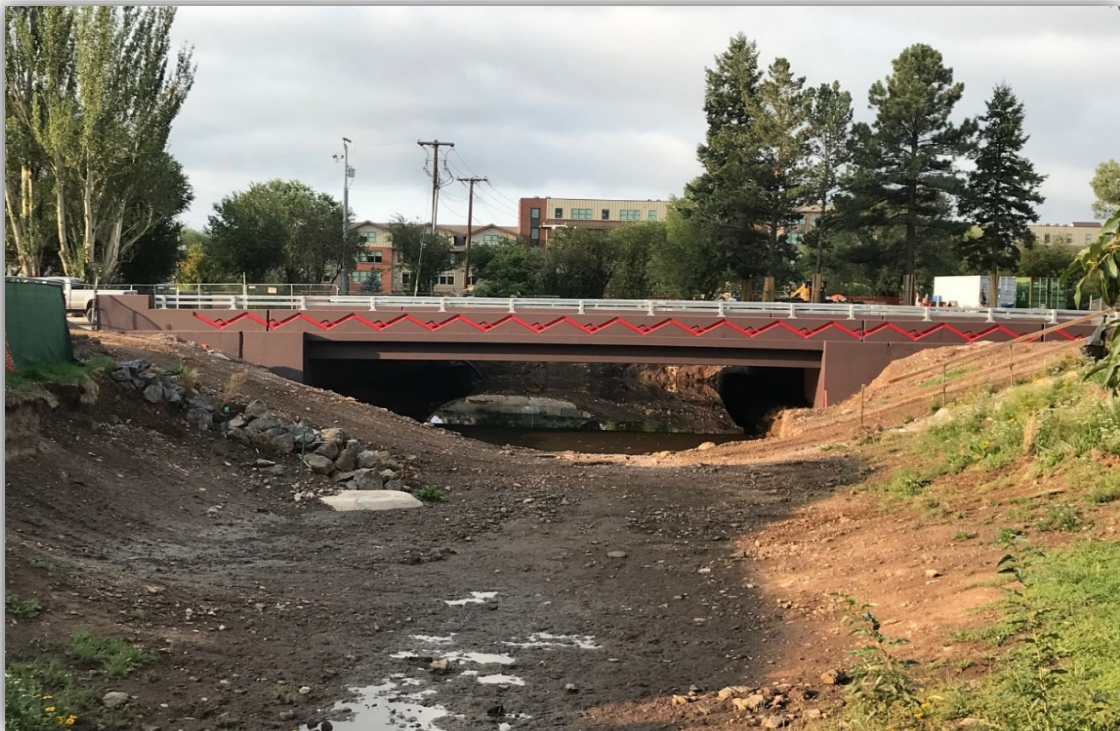
Bridge structure with new paint
