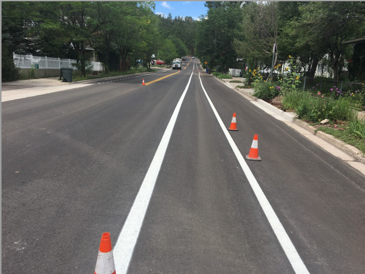
Summit Waterline Project-New striping on Santa Fe Ave installed by Streets
