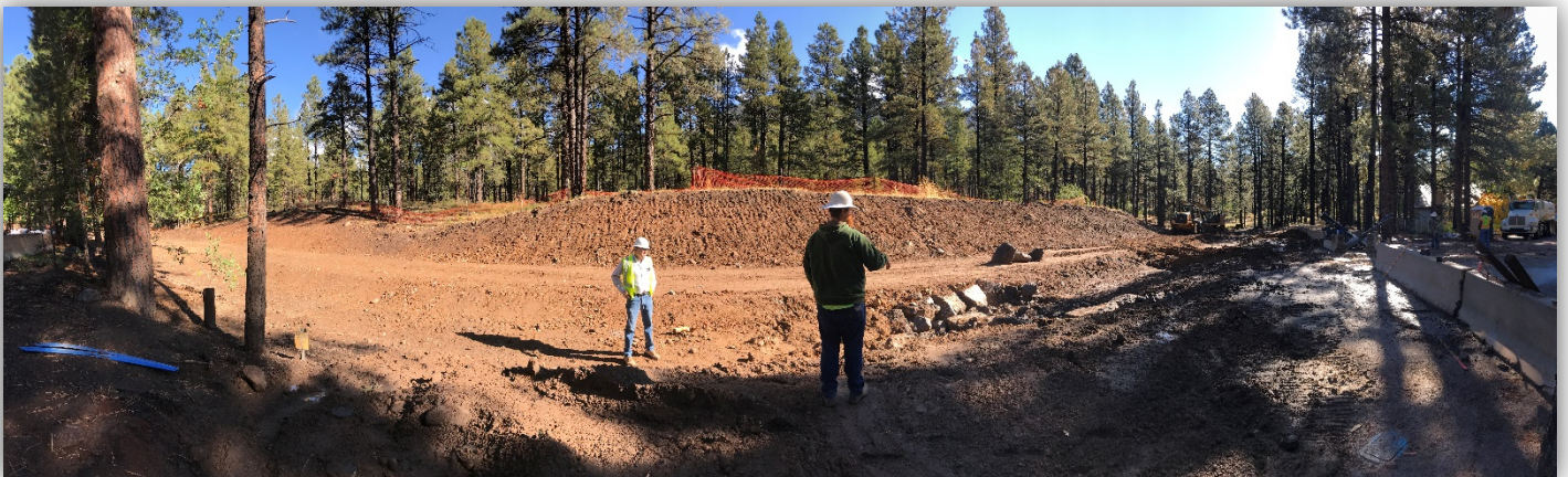
Image Taken on 6 October During Walkthrough Meeting of Channel Widening Project.
