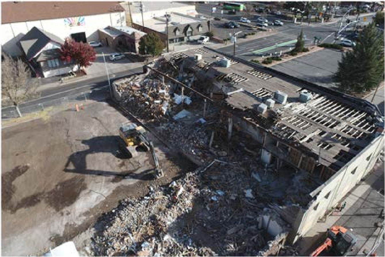
Old Municipal Court Building Demolition
