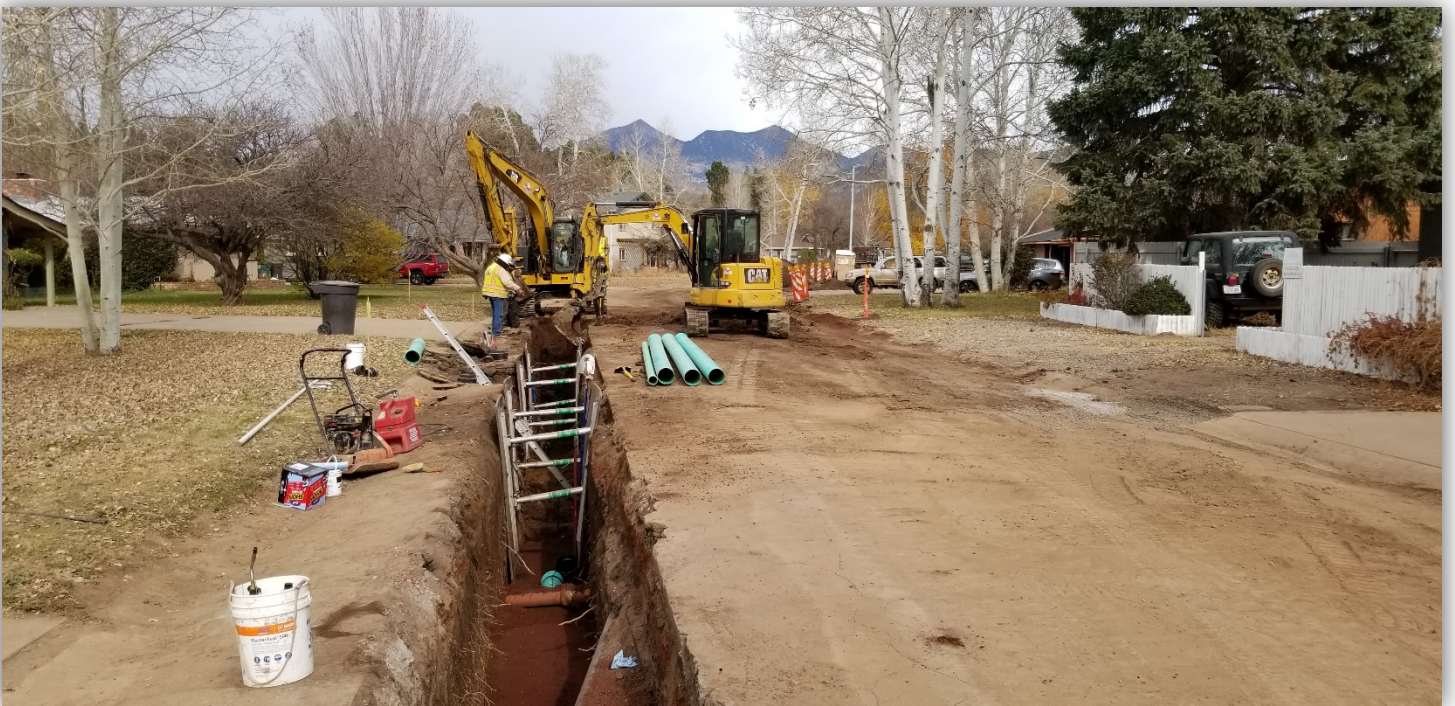
Navajo Rd. north of Beal Rd., looking north at sewer installations.
