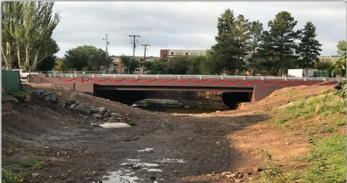
Bridge structure with new paint
