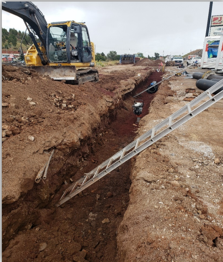
Installation of the 16" waterline
