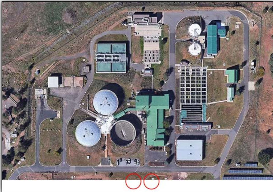
Existing Wildcat Plant, red circles represent proposed location of the two new digesters
