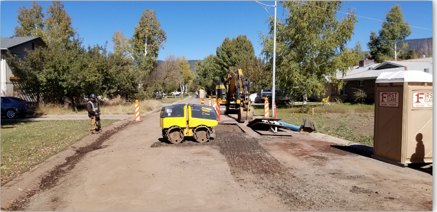
Navajo Rd. north of Beal Rd., looking north at water installations.
