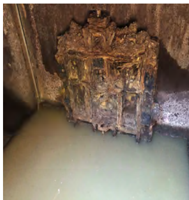
Old Valve – Replaced
