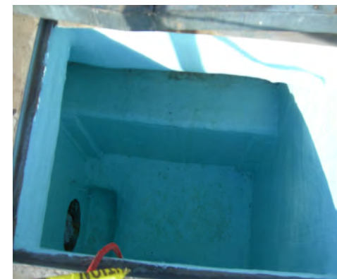
Repaired and coated concrete
