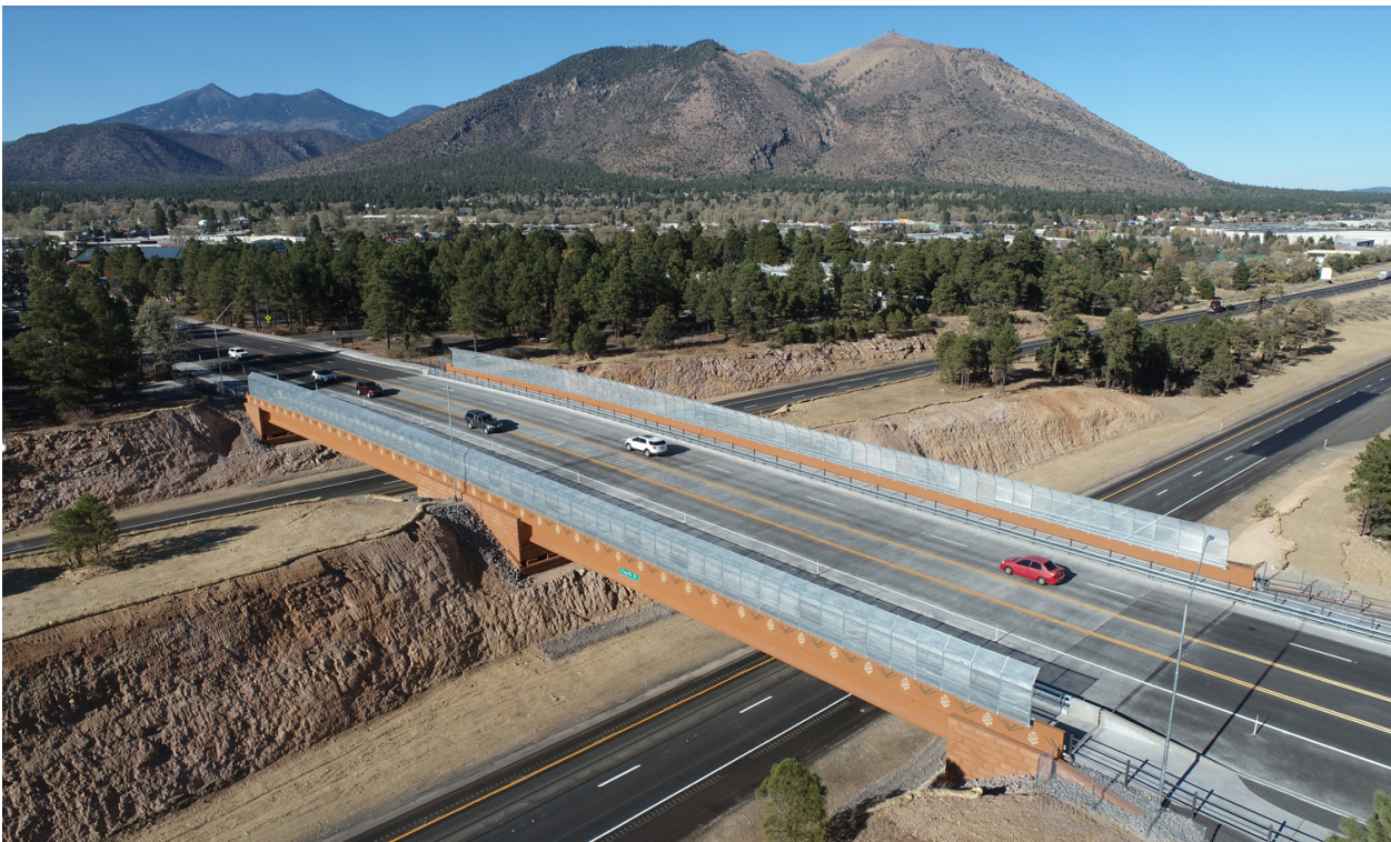
2020 Fourth Street Bridge After Completion: The project utilized an innovative bridge slide method that significantly reduced closures of Fourth St from 3-4 months with traditional methods to 17 days.
