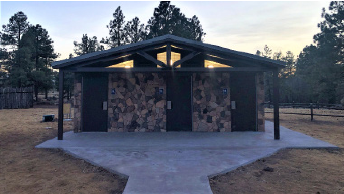
New restrooms at Buffalo Park
