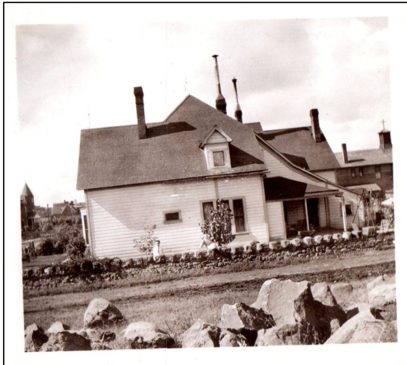
Figure B-2. North elevation as seen along West Dale Avenue, ca. 1906 (scan provided by FSL Real Estate Services).
