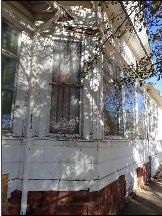
Figure C-15. Detail of the cutaway bay window with canted walls of the formal living room, built by 1901.
