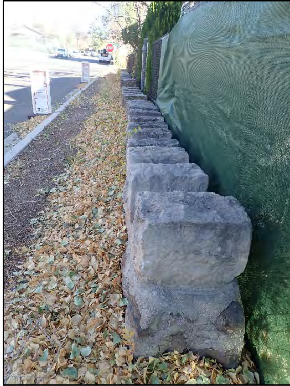
Figure C-61. Detail of the original masonry wall along West Dale Avenue.
