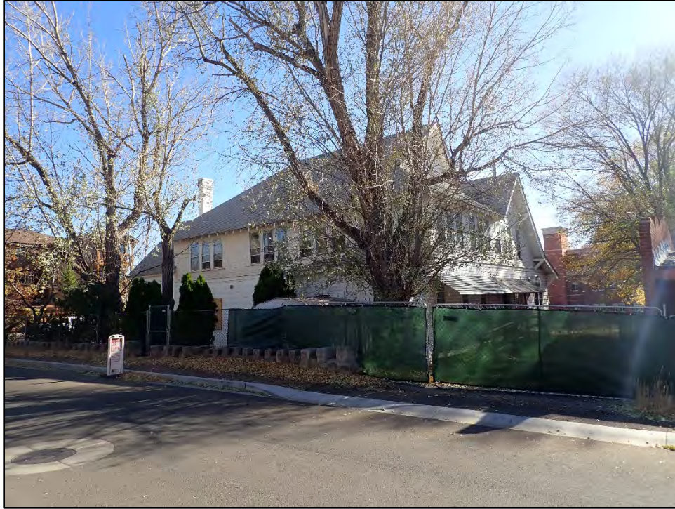
Figure C-5. North and west elevations as seen from West Dale Avenue.
