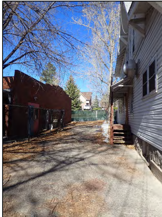
Figure C-56. Alternate view of the side yard between the former school and the residence, showing how close the former classroom annex was placed when constructed in the mid-1950s.
