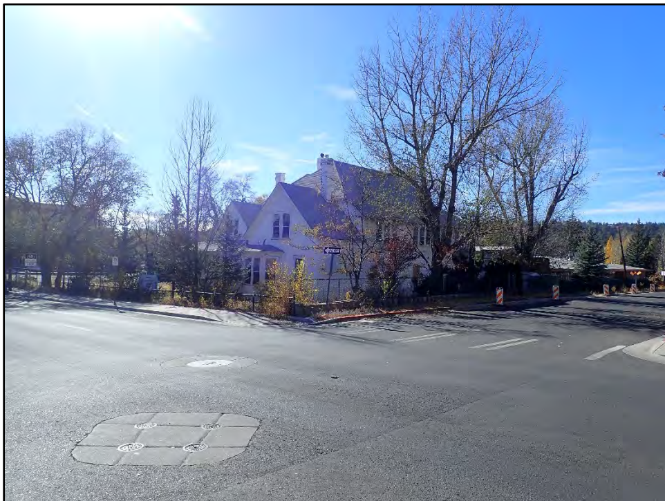
Figure C-2. East and west elevations as seen from the intersection of North Beaver Street and West Dale Avenue.
