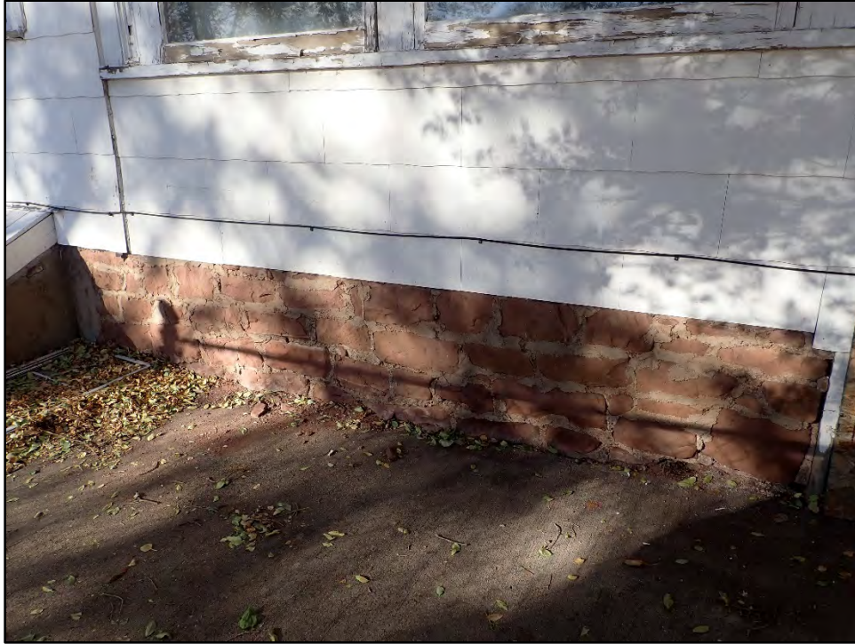
Figure C-37. Detail of the red sandstone foundation constructed to support the dining room and kitchen added to the southwest corner of the residence between 1910 and 1916.
