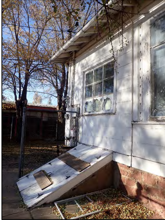
Figure C-11. Detail of the outside entrance to the partial basement and the exterior window of the kitchen, both of which were added between 1910 and 1916.
