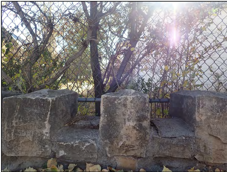
Figure C-62. Detail of the top of the original masonry wall with the large Coconino sandstone blocks as seen along West Dale Avenue.
