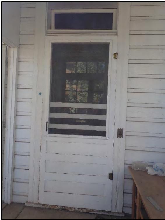
Figure C-22. The existing screen door of the front entrance, showing the simple-drop wood siding, upper transom, door trim, and doorbell, all of which are original to the 1886 home (see Figure B-7 in Appendix B).
