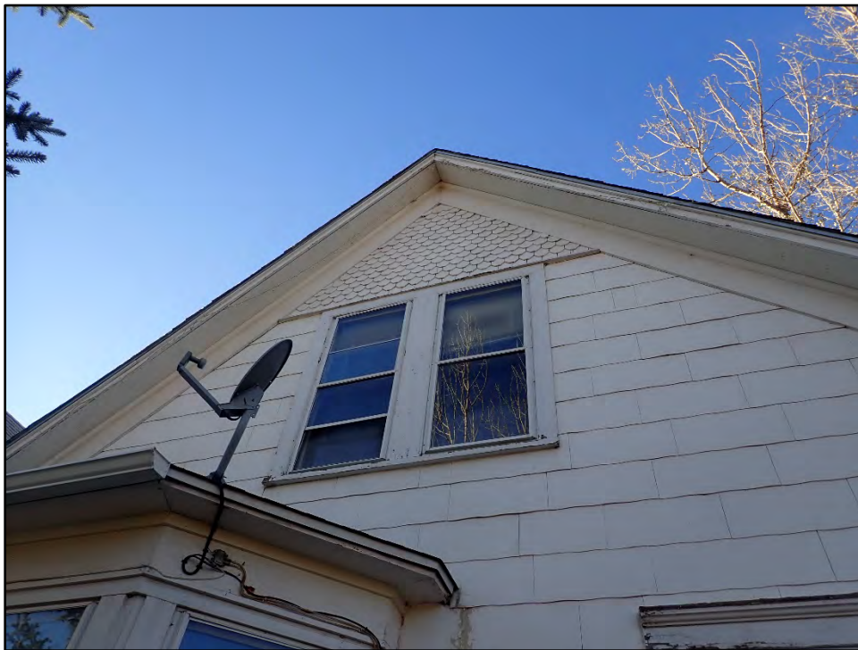
Figure C-26. Detail of the lower cross gable above the master bedroom.
