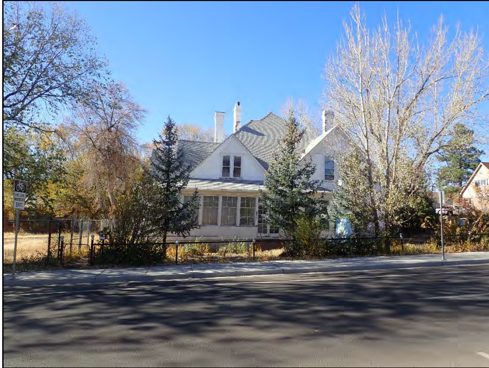
Figure C-1. East elevation as seen along North Beaver Street.
