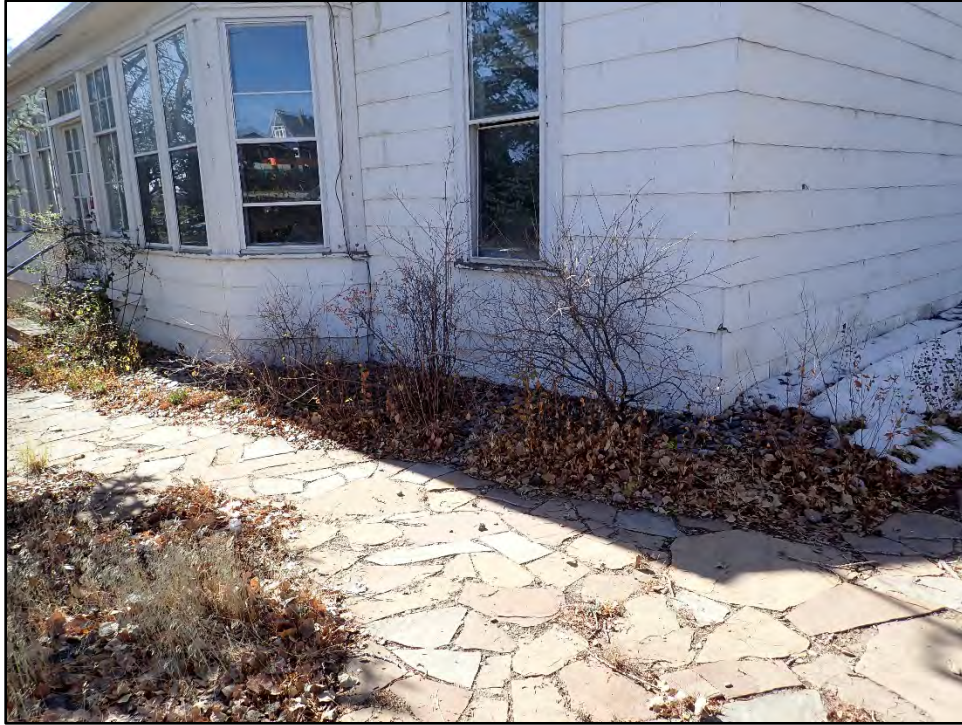
Figure C-47. View of the modern flagstone pavers placed to create a walkway around the east and north sides of the residence.
