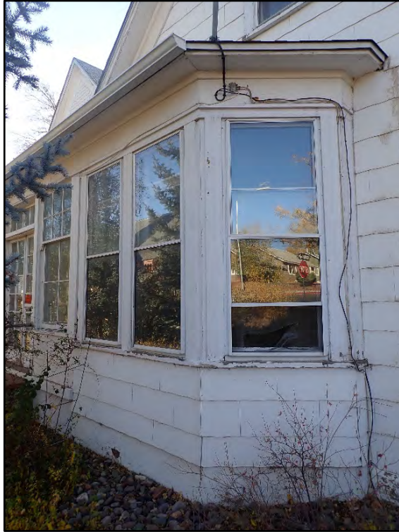
Figure C-25. Detail of the cant bay window of the master bedroom, the exterior shape of which was lost when the porch was enclosed after 1958).
