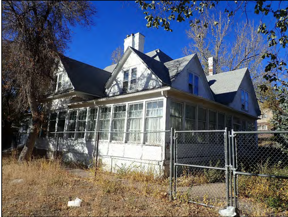
Figure C-35. Details of the south and east elevations showing the enclosed porch (dating to after 1958), three original 1886 lower cross gables, and the larger gable added by 1901 (on the left).
