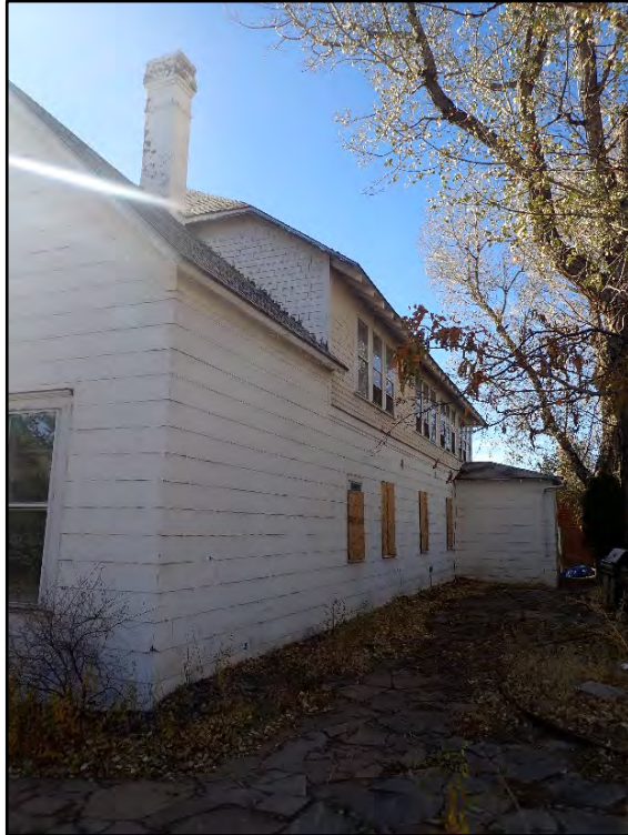
Figure C-29. North elevation, showing the profile of the addition to the chapel added between 1948 and 1958.
