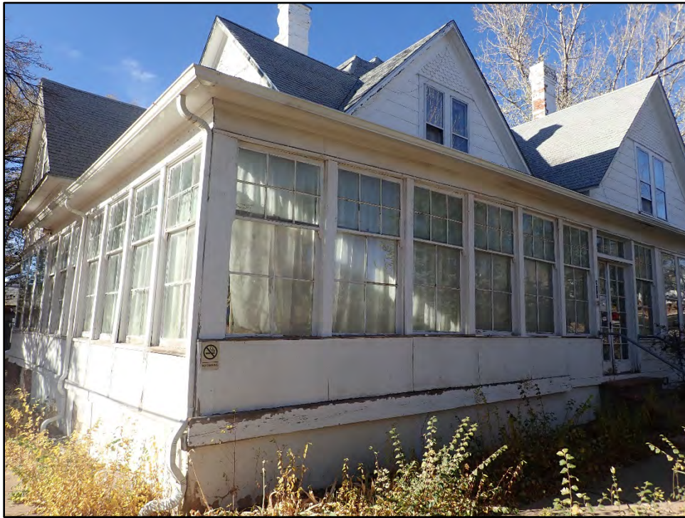
Figure C-16. Detail of the existing wrap-around porch, which incorporates Craftsman-style windows repurposed from an older building (porch was reconstructed and enclosed after 1958).
