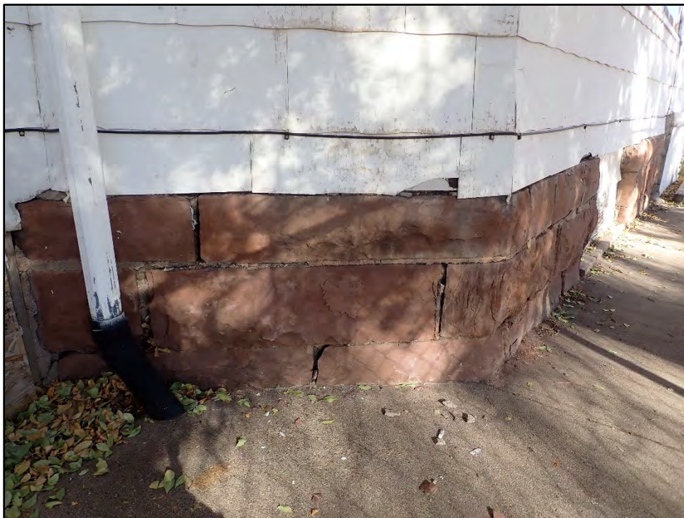
Figure C-36. Detail of the Moenkopi red sandstone foundation of the cant bay window of the formal living room, constructed between 1895 and 1901.
