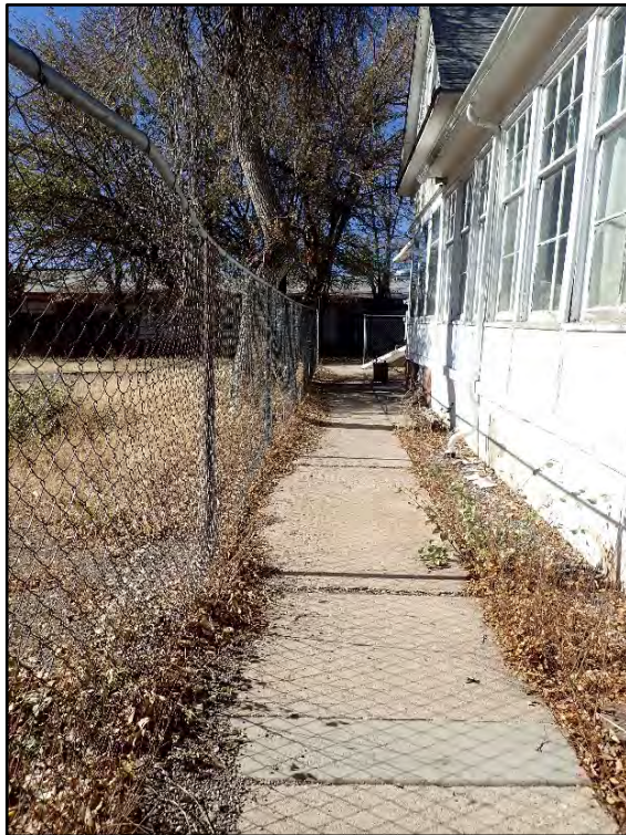
Figure C-58. Alternate view of the modern concrete sidewalk along the south side of the residence from North Beaver Street.
