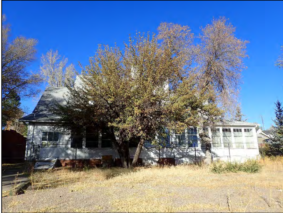
Figure C-33. Overview of the south elevation.
