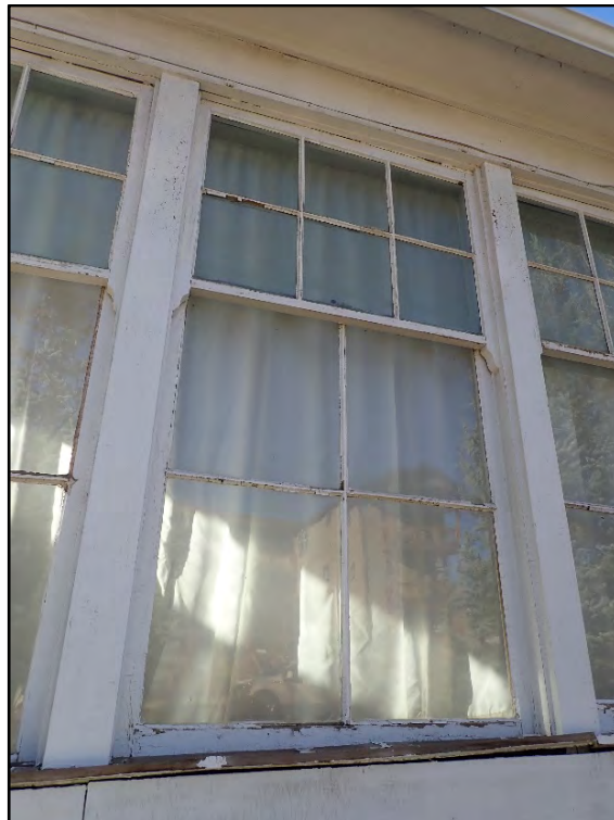
Figure C-18. Detail of one of the porch windows, which still retain their original glass panes.
