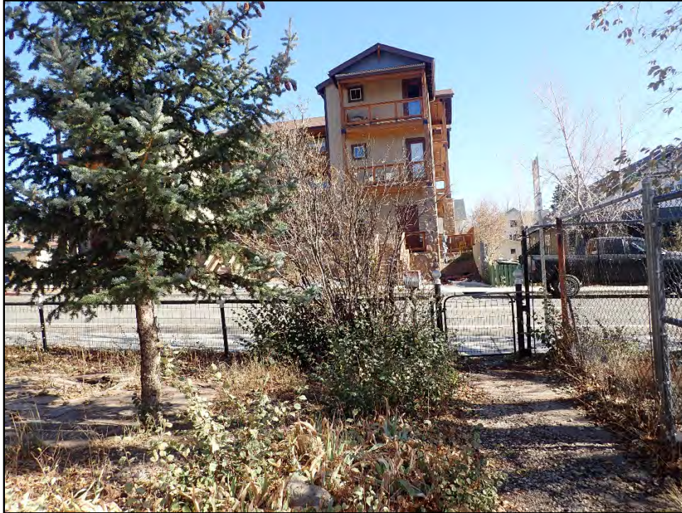
Figure C-39. View of the West Dale condominium development completed in 2018 on the east side of North Beaver Street.
