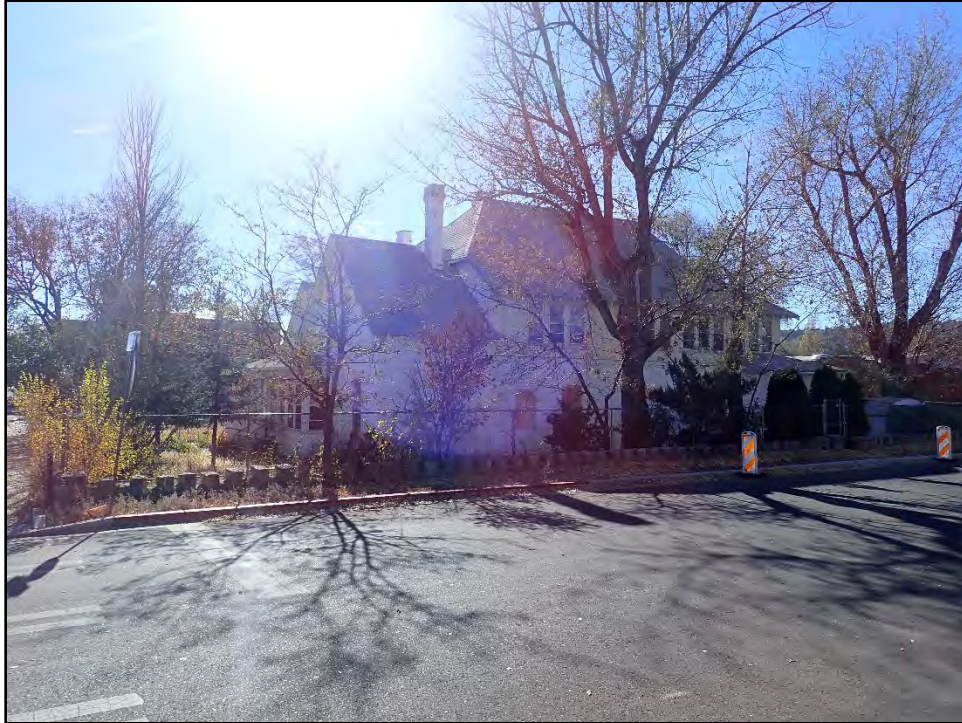
Figure C-3. East and north elevations as seen along West Dale Avenue.
