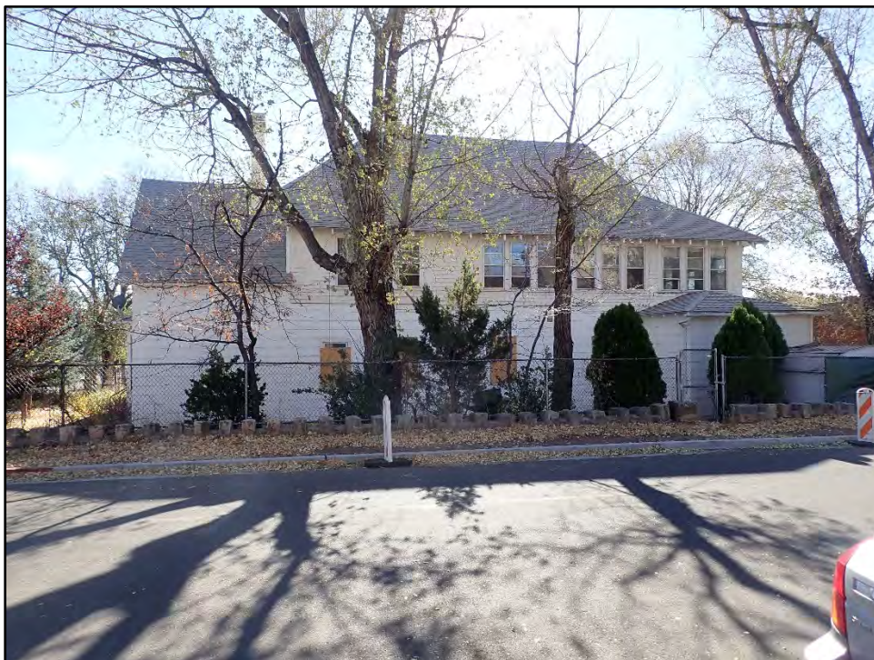
Figure C-4. North elevation as seen along West Dale Avenue (note the original masonry retaining wall along the edge of the roadway).
