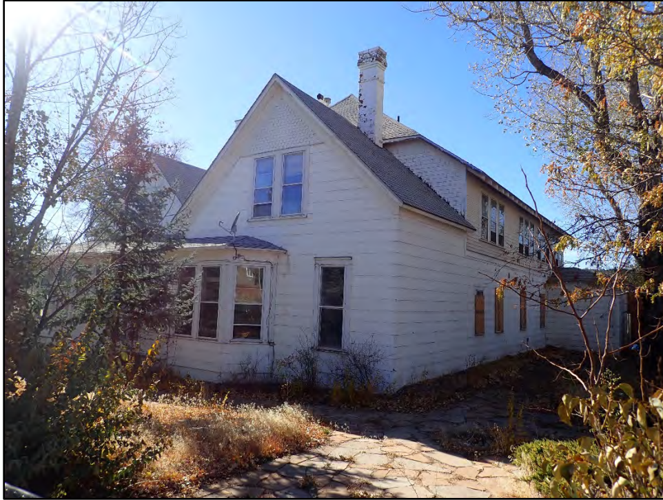
Figure C-27. East and north elevations, showing portions of the original 1886 construction and the major renovations completed between 1910 and 1916.
