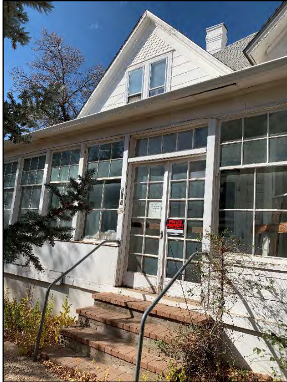
Figure C-19. Detail of the wrap-around porch facing North Beaver Street below one of the lower cross-gables of the original 1886 construction.
