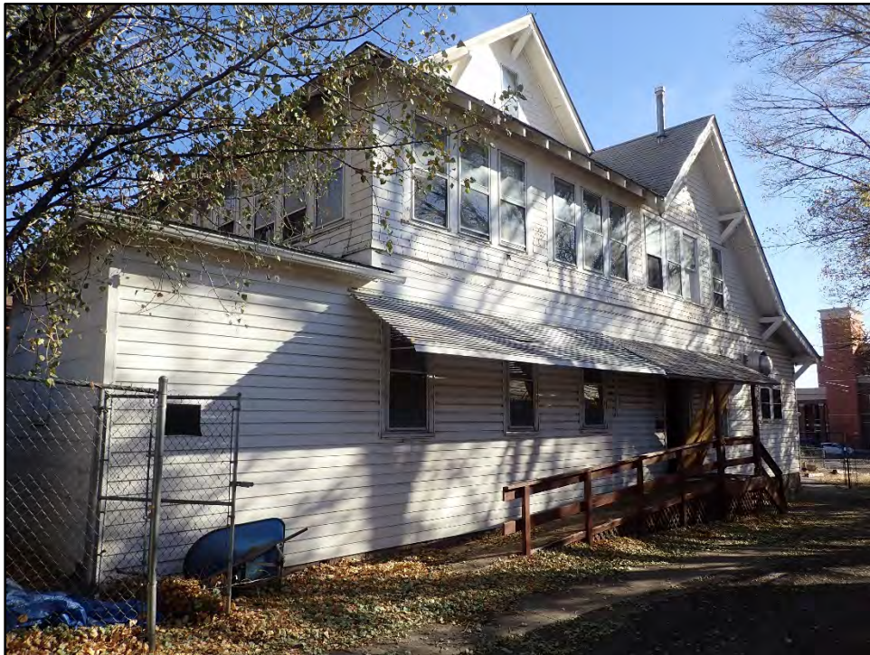
Figure C-6. West elevation as seen from next to the former Catholic school.
