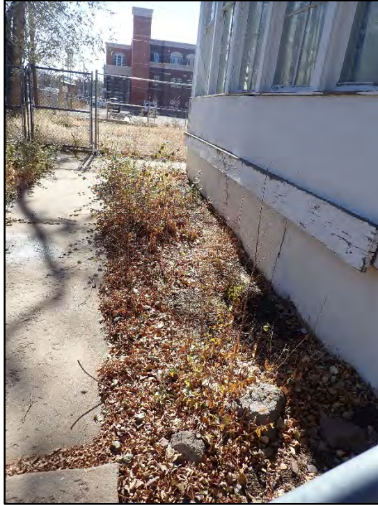
Figure C-41. Detail of the sidewalk and concrete foundation of the wrap-around porch (the new Flagstaff Municipal Courthouse towers in the background).
