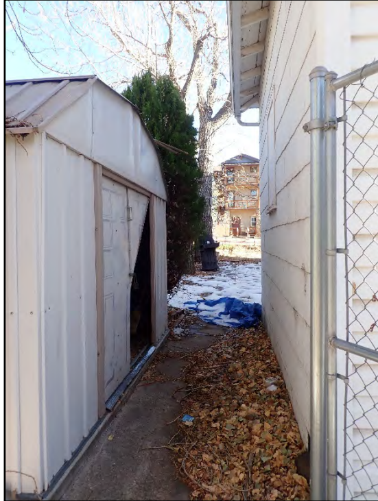
Figure C-53. Detail of the north side of the chapel extension with the modern shed (recently broken into while field documentation was occurring).
