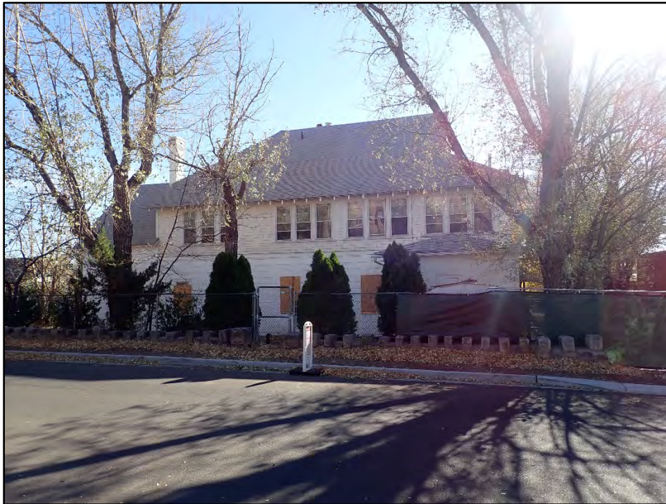
Figure C-60. Overview of the north side of the residence, showing the original masonry wall (with Coconino sandstone blocks) along West Dale Avenue (see Figures B-2 and B-5 in Appendix B for comparison).
