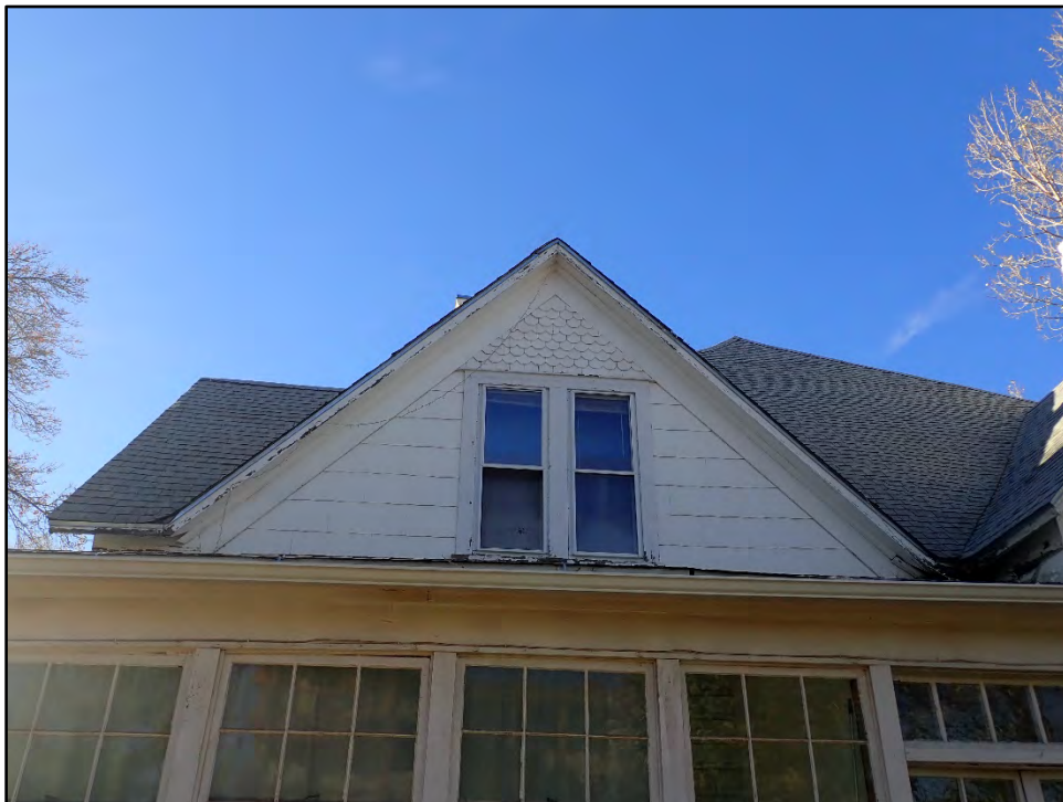
Figure C-24. Detail of one of the lower cross gables above the existing wrap-around porch.
