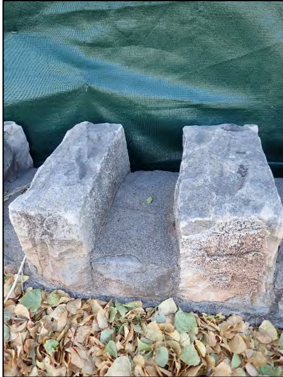
Figure C-63. Alternate detail of the Coconino sandstone blocks, showing the workmanship of the masonry wall.
