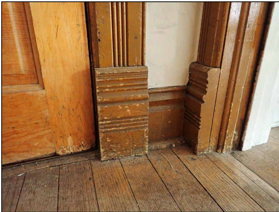
Figure D-38. Detail of the decorative plinth blocks and baseboards over the original hardwood floors near the front door and sitting room.
