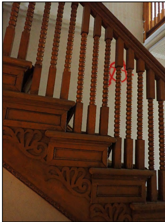
Figure D-52. Alternative view of the wood detailing of the balustrade and staircase.
