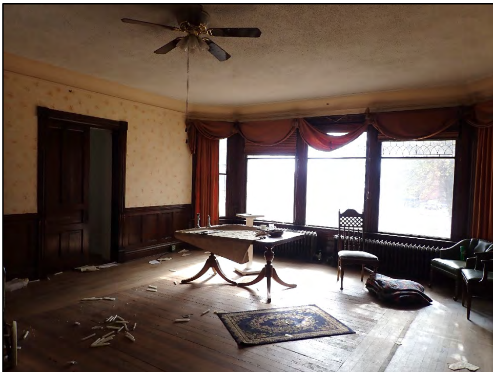
Figure D-90. View of the cottage windows with canted walls and the pocket door to the sitting room (right).
