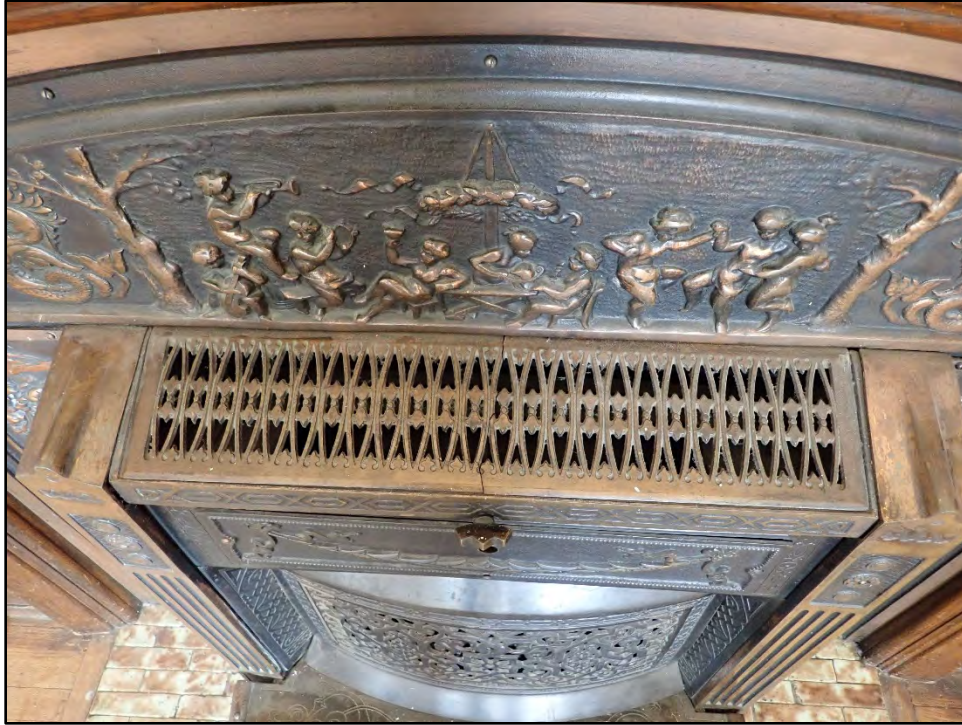
Figure D-105. Detail of the top of the fireplace inset.
