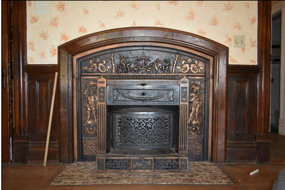
Figure D-103. The fireplace of the formal living room.
