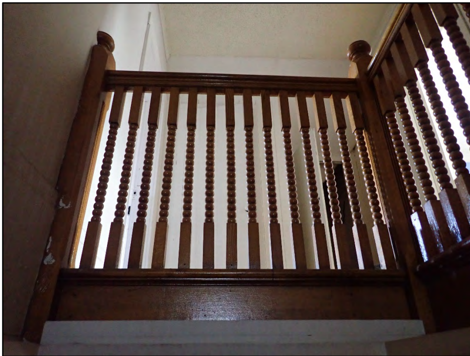
Figure D-46. View of the balustrade (with newel post at each side) on the second floor.
