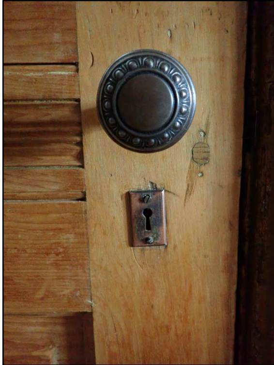
Figure D-31. Detail of the embossed copper doorknob and small key opening as seen on the interior of the front door.
