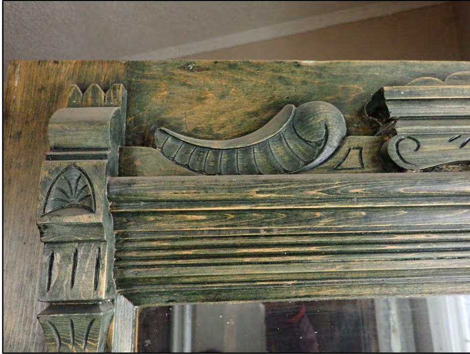
Figure D-25. Close-up view of the decorative door details.
