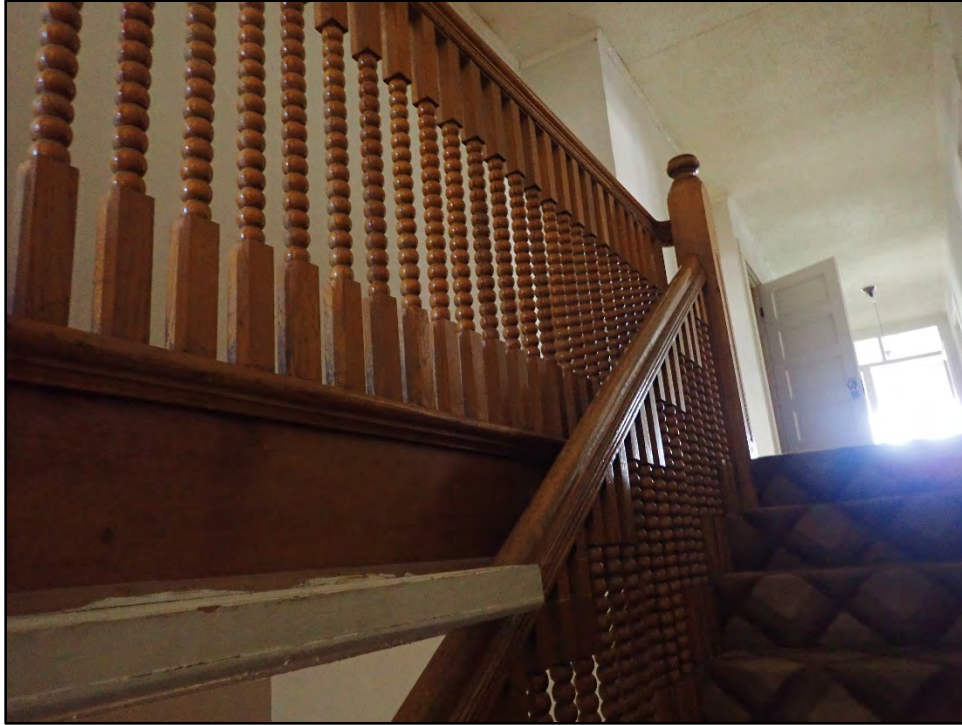
Figure D-45. Detail of the balustrades up the stairs and along the second floor.
