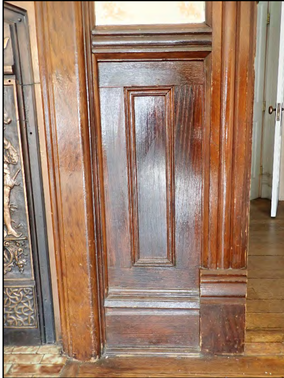
Figure D-115. Detail of the wood panel between the fireplace and the door jamb.
