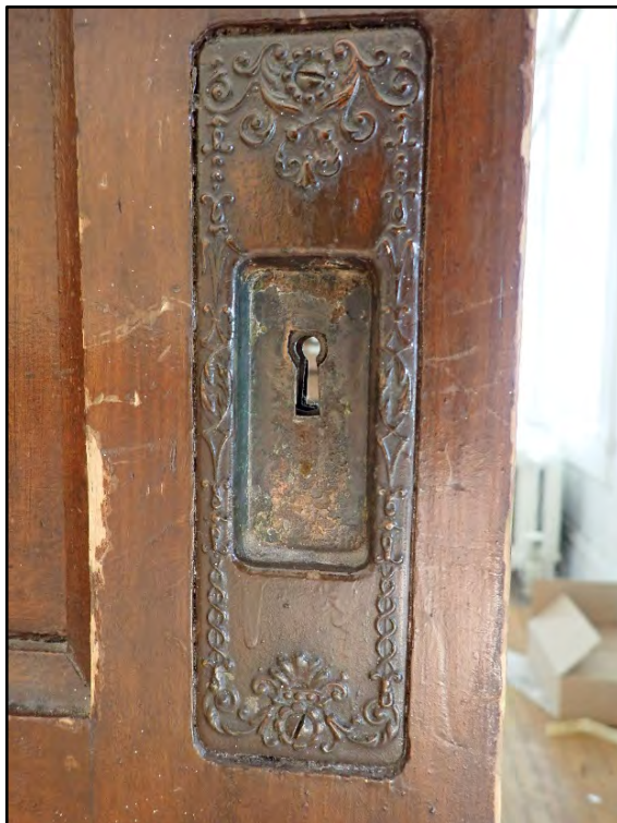
Figure D-84. Close-up of the lock plate of pocket door to the sitting room.
