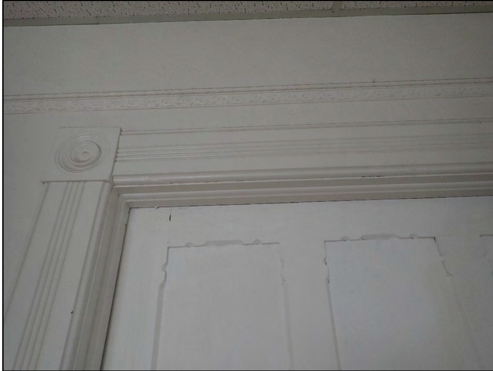
Figure D-63. Detail of the pocket door's decorative side casings and corner blocks, with the strip of ornate picture molding on the wall above.
