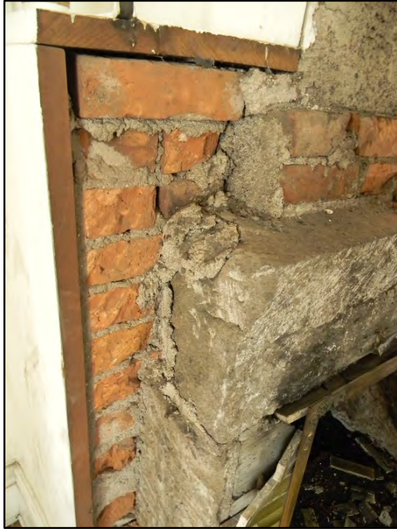
Figure D-73. Detail of the construction and workmanship of the sitting room fireplace.
