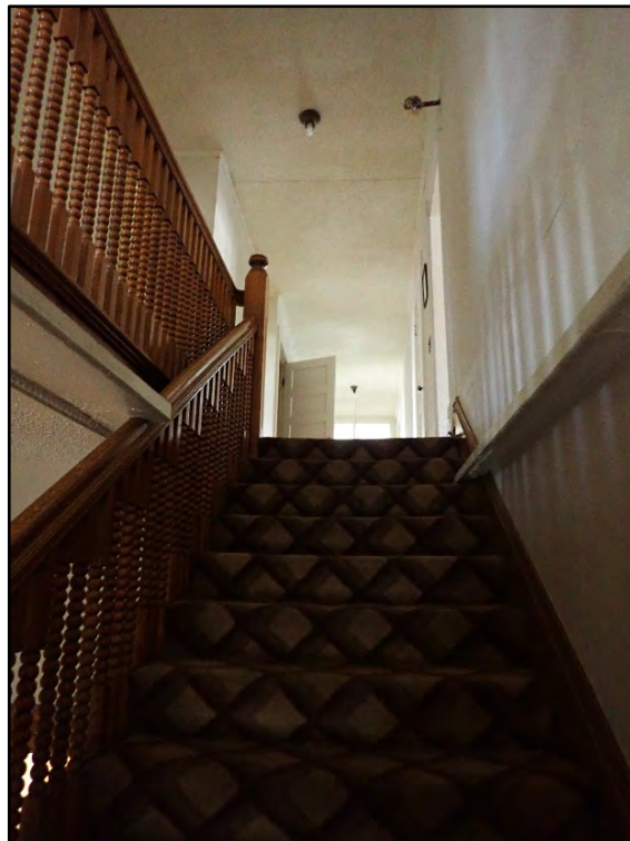
Figure D-44. View of the second floor as seen from midway up the main staircase.
