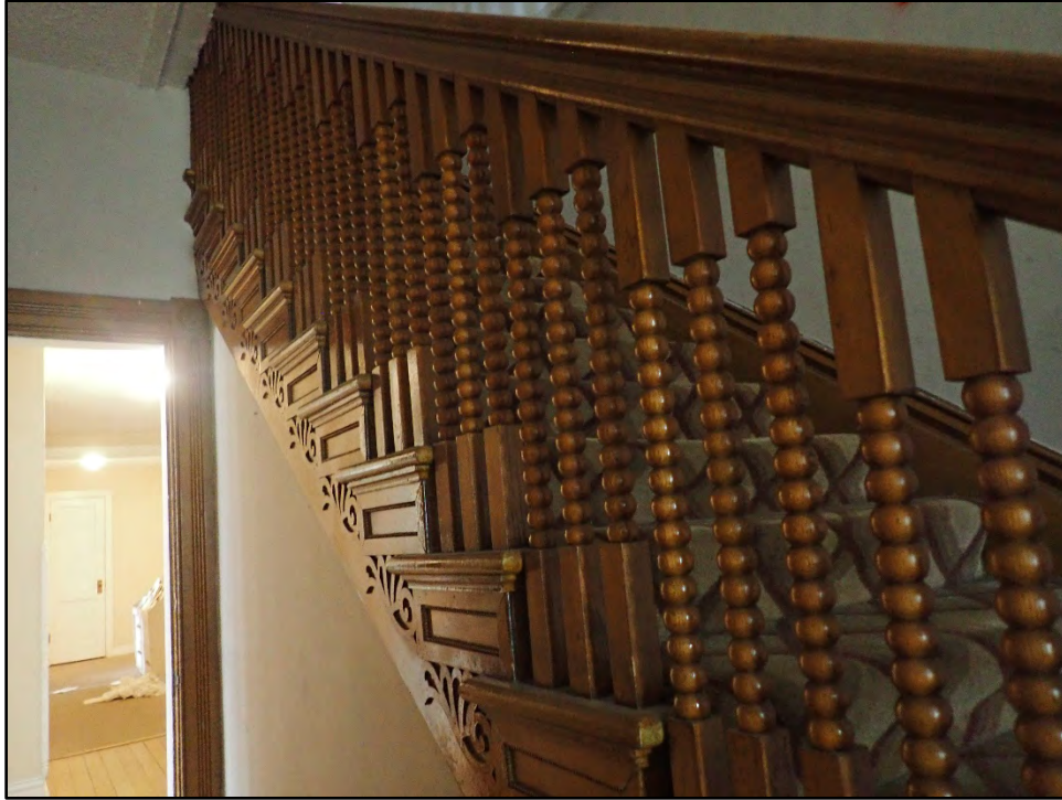
Figure D-51. View of the face stringerboard, turned balusters, and railing of the main staircase.
