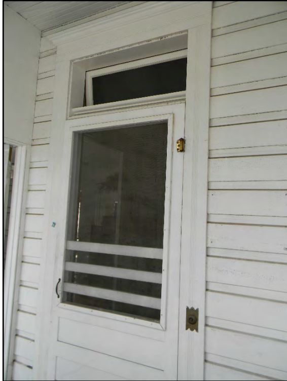
Figure D-5. View of the screen door and upper transom (note the doorbell).
