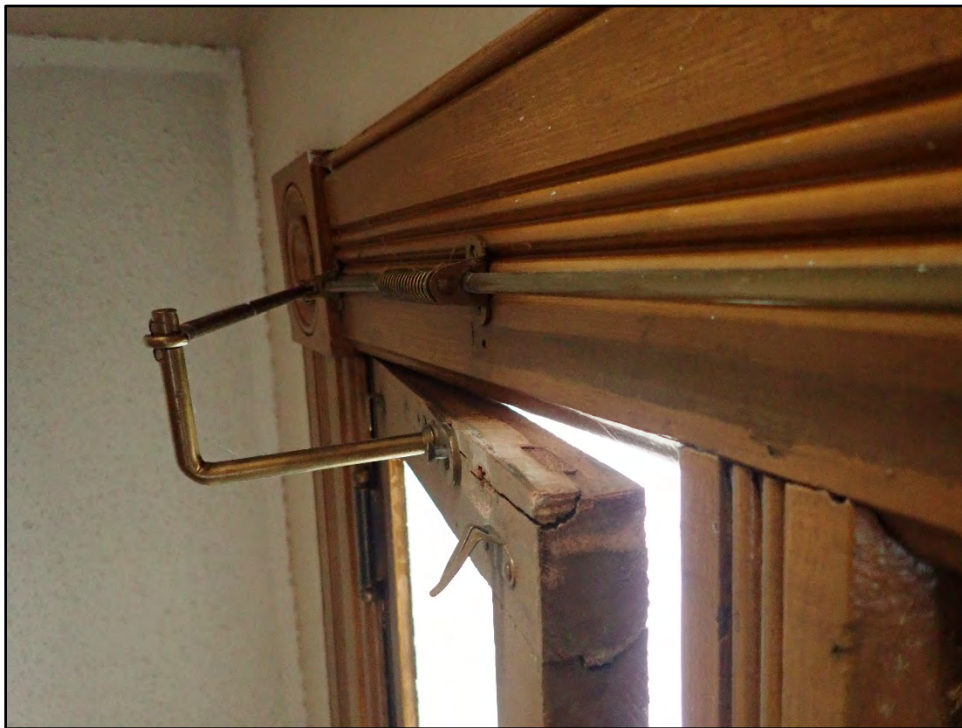
Figure D-34. Close-up view of the opening mechanism for the transom window.
