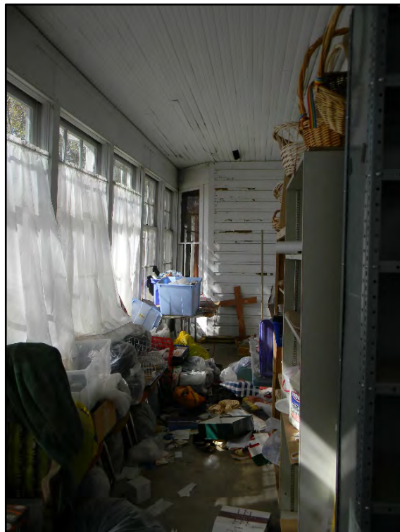
Figure D-12. View of the south side of the enclosed porch (toward the formal living room).
