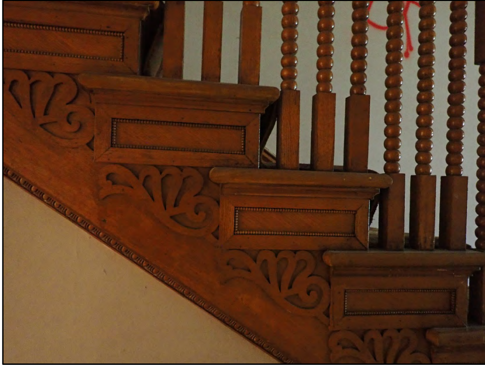
Figure D-53. Detail of the decorative wood details, including carved wood appliques.
