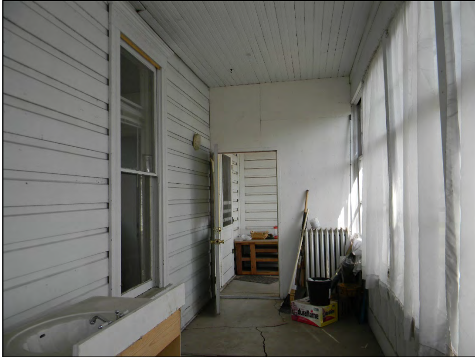
Figure D-19. View back toward the front door and entryway as seen from the enclosed porch (the drywall divider and door are modern).
