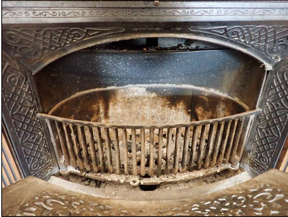
Figure D-109. Interior of the fireplace with the fire screen removed.
