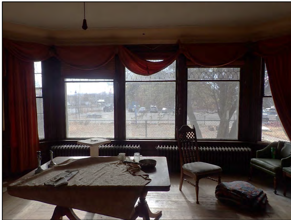
Figure D-98. View of the canted bay window in the formal living room (likely constructed as a formal dining room when built by 1901).
