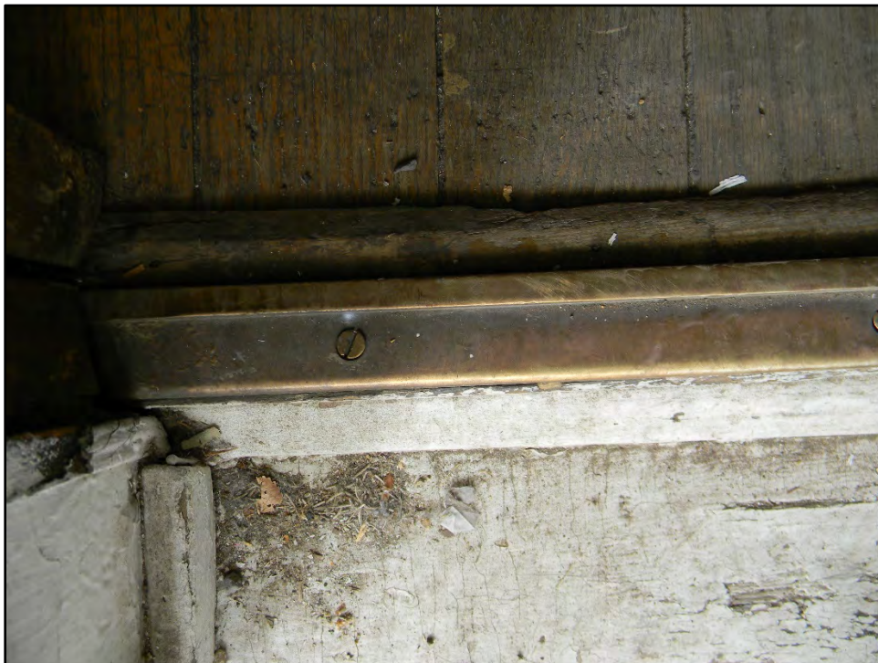
Figure D-8. Detail of the original brass floor strip at the base of the front door.
