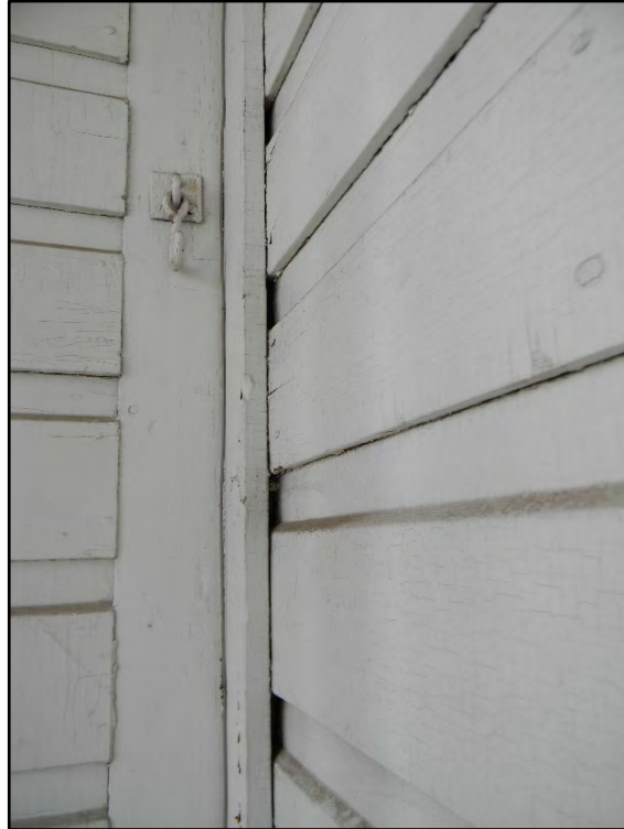
Figure D-17. Close-up view of the original simple-drop siding still visible today.
