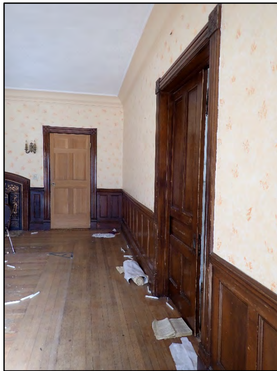
Figure D-82. View of the pocket door to the sitting room and the modern replacement door to the hall.
