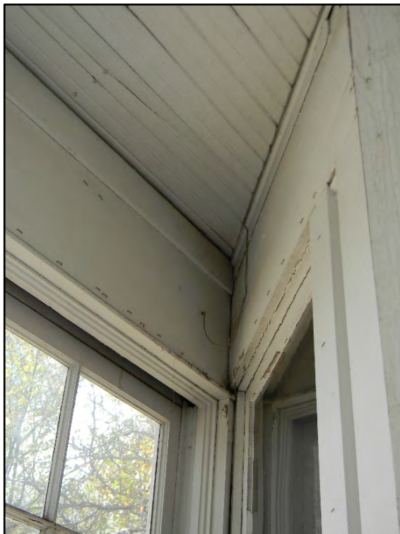
Figure D-16. Close-up view of the enclosed porch with cant bay window and the roof that was placed over it after 1958.
