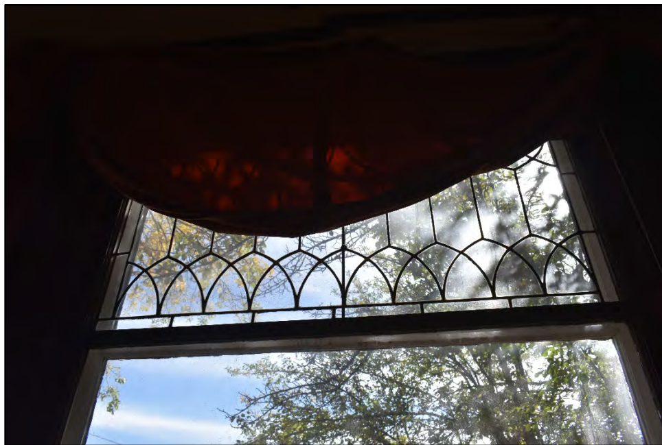
Figure D-102. Light has shown through these windows for upwards of 120 years.
