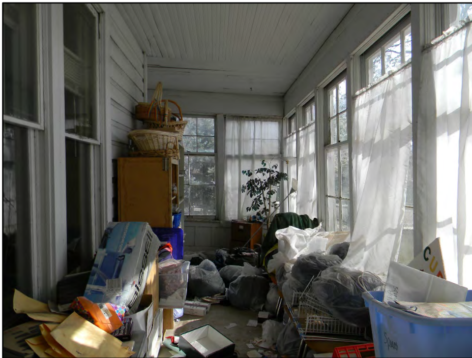
Figure D-18. View back toward the corner of the enclosed porch.
