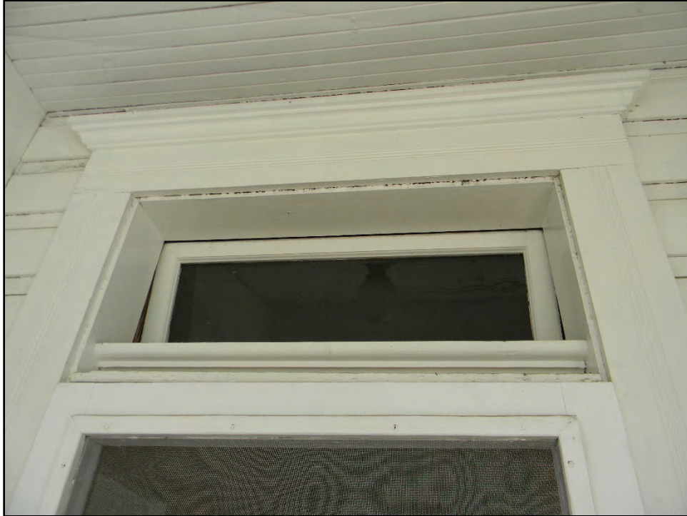
Figure D-7. Close-up view of the upper transom and decorative cap molding above.
