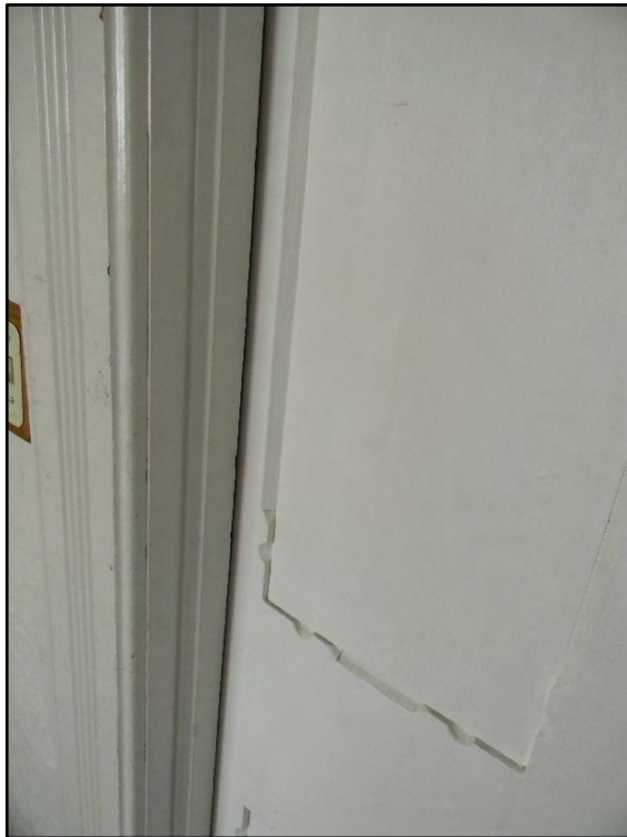
Figure D-62. Detail of the pocket door's scalloped recessed panels and door trim.
