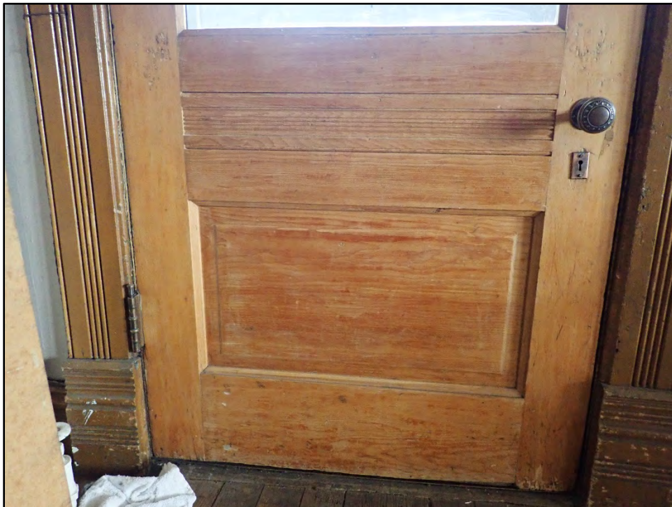
Figure D-30. Lower portion of the front entryway door.
